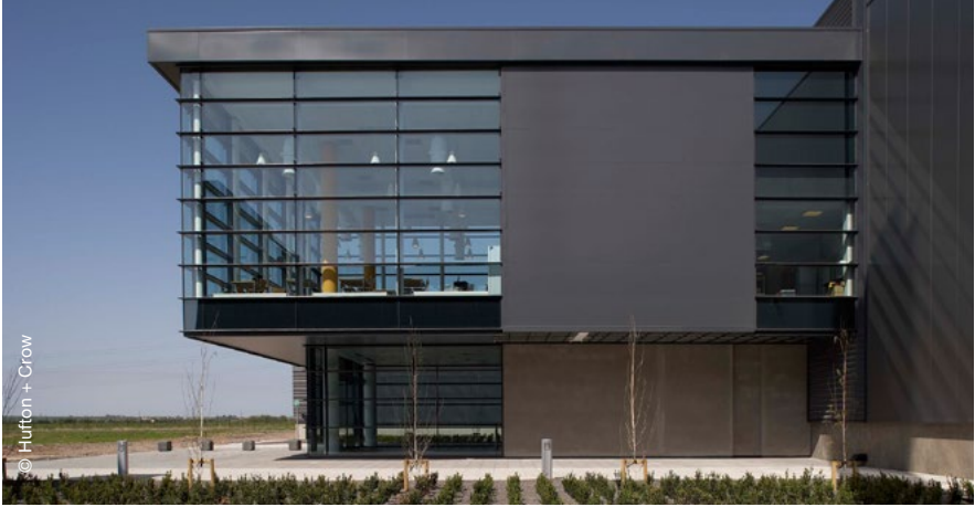
Packaging facility and warehouse for Gerber Foods & Soft Drinks Ltd, Somerset, UK (Arup)
