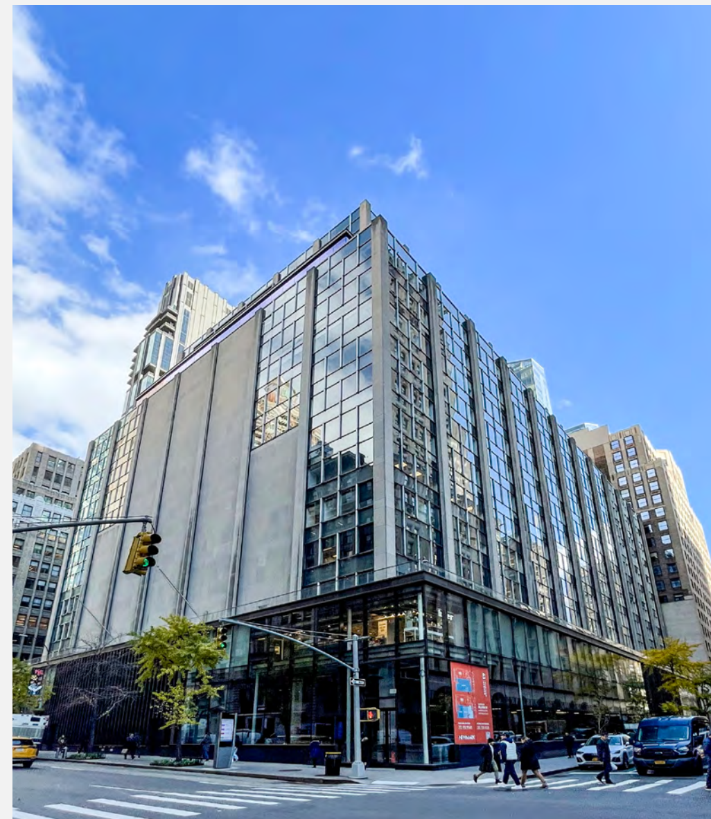
Wide Curtain Wall
