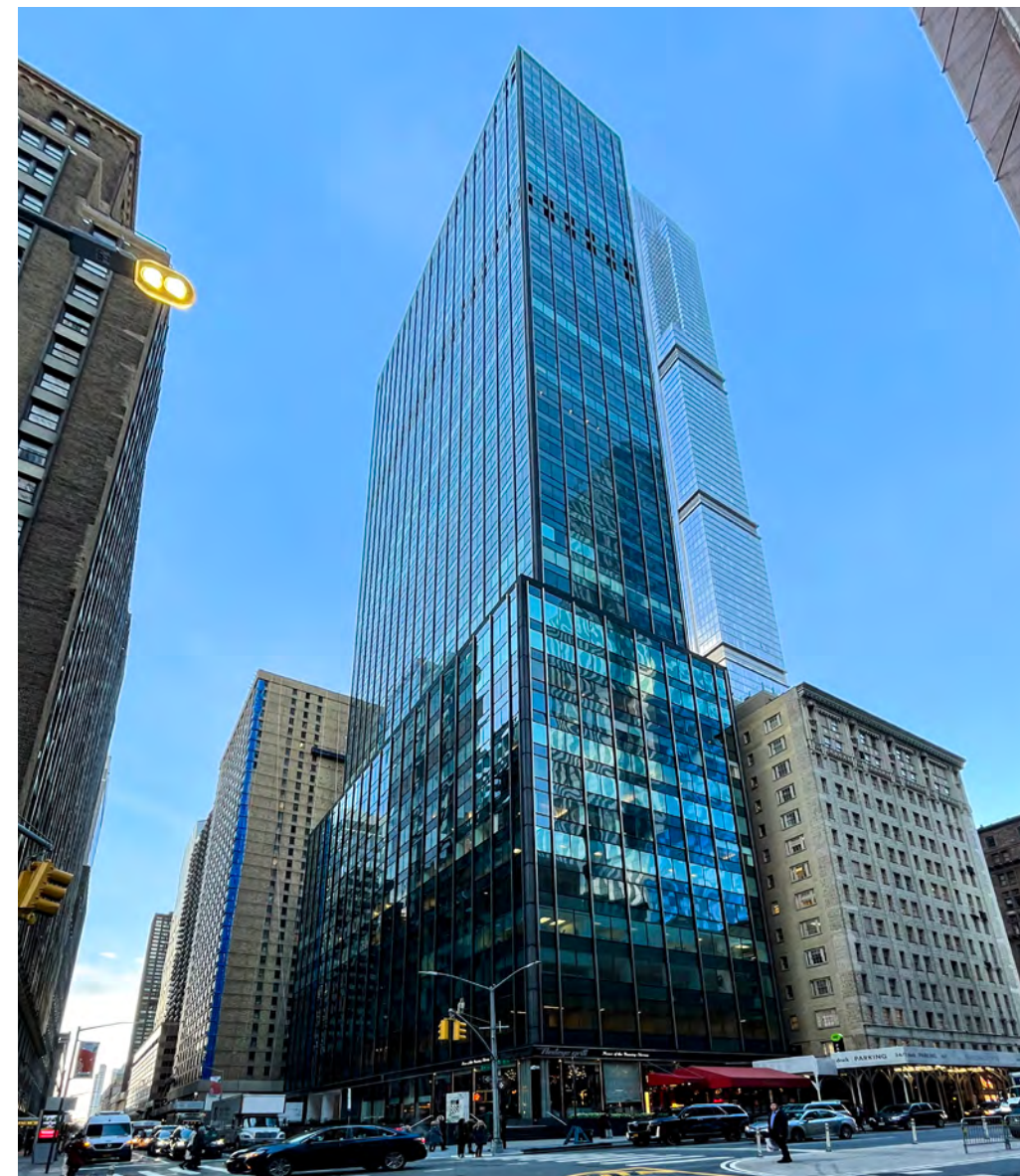
Wide Curtain Wall
