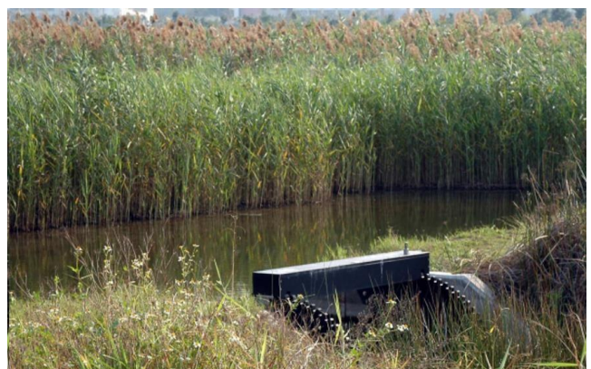
© Arup An extensive reedbed provides biofiltration function as well as habitat for reed-associated wildlife.
