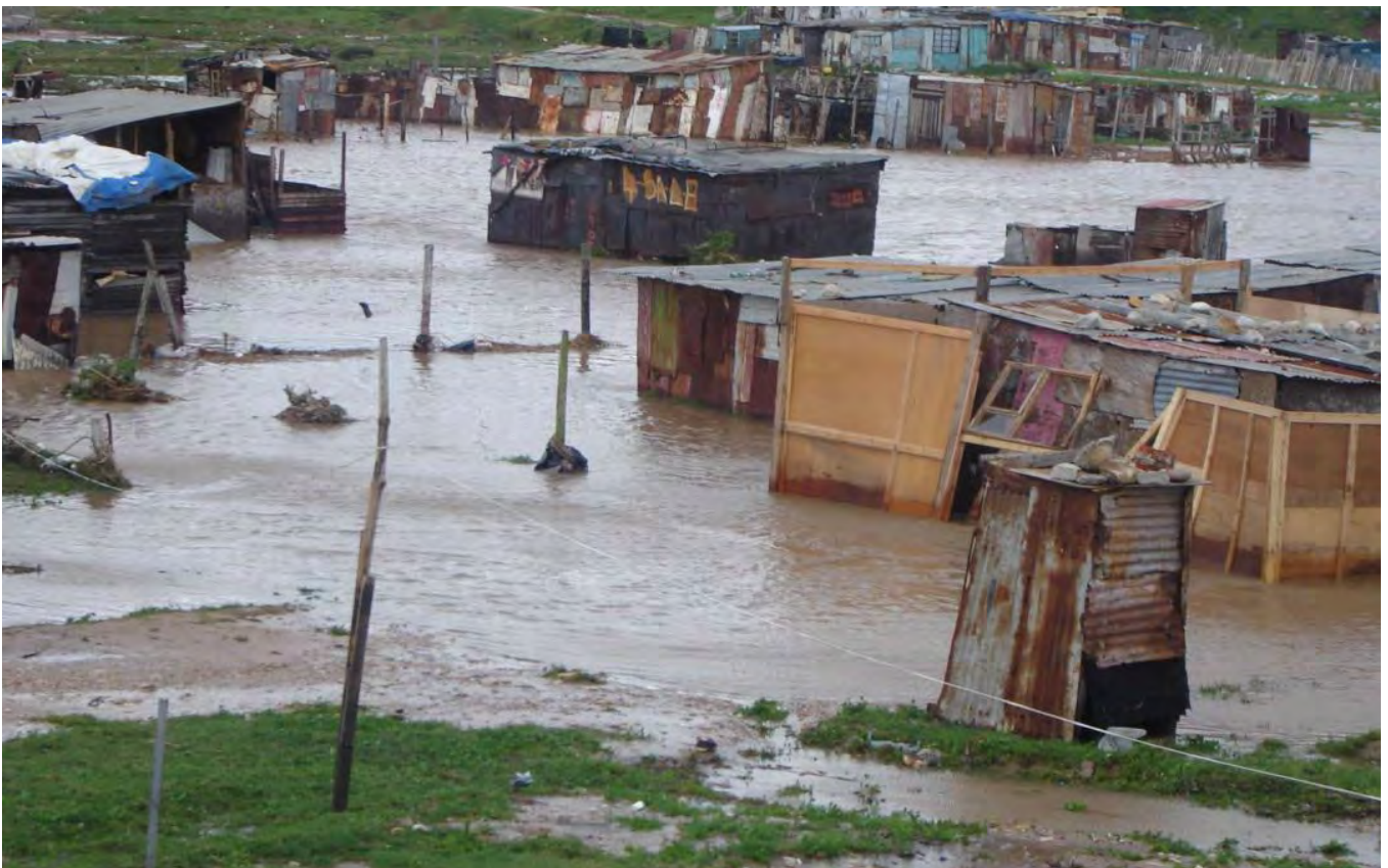
Figure 4-9. Impacts of flooding on an informal settlement in Gqeberha in 2006 (NMBM, n.d.)
