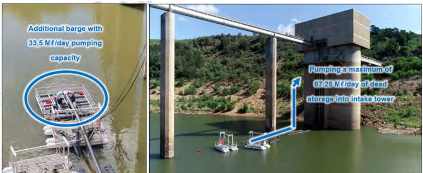
Figure 8-1: Upgrading barges in Impofu Dam (NMBM, 2022a)
