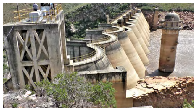
Figure 3-5. Top View of Churchill Dam Wall and Intake Tower (Nov 2021) (Zutari, 2022)
