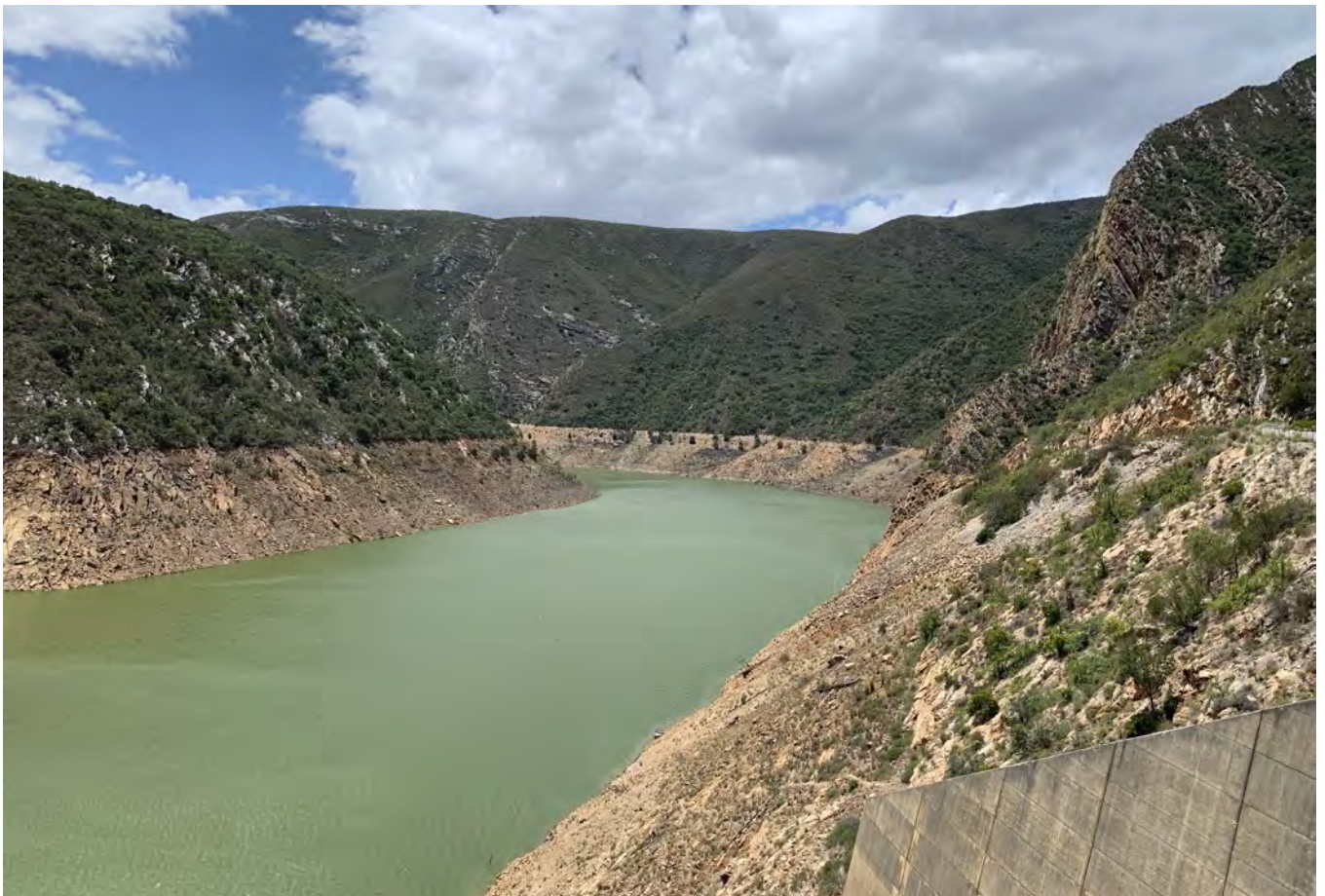
▲ Figure 4-6. Kouga Dam spilling (left) and Kouga Dam in 2022 (right) (DWS, 2022)
