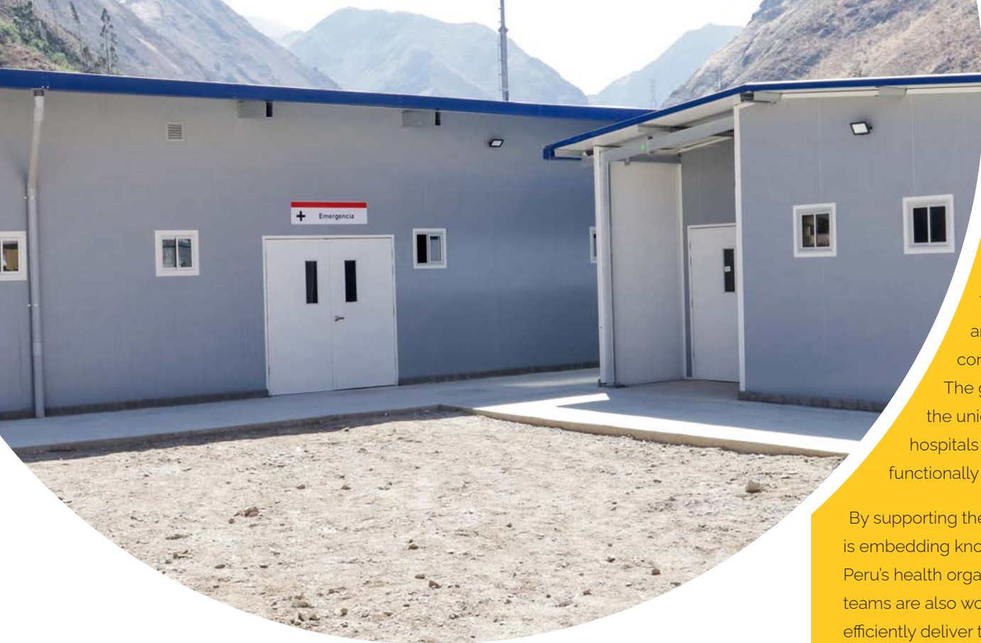
Temporary hospital in Matucana built in half the usual time
