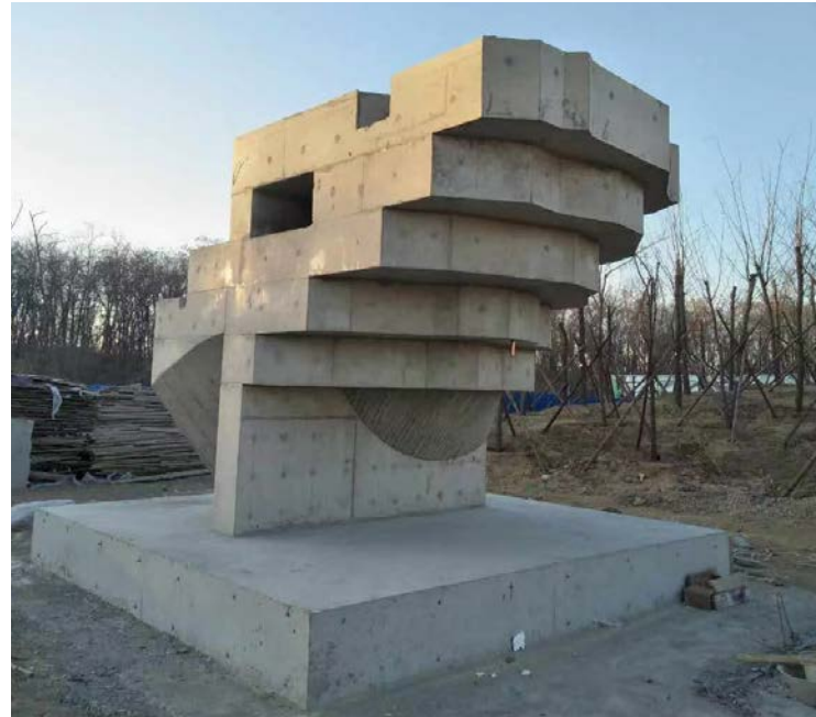
13: A full-scale mock-up was made of the most challenging area of the outer shell
