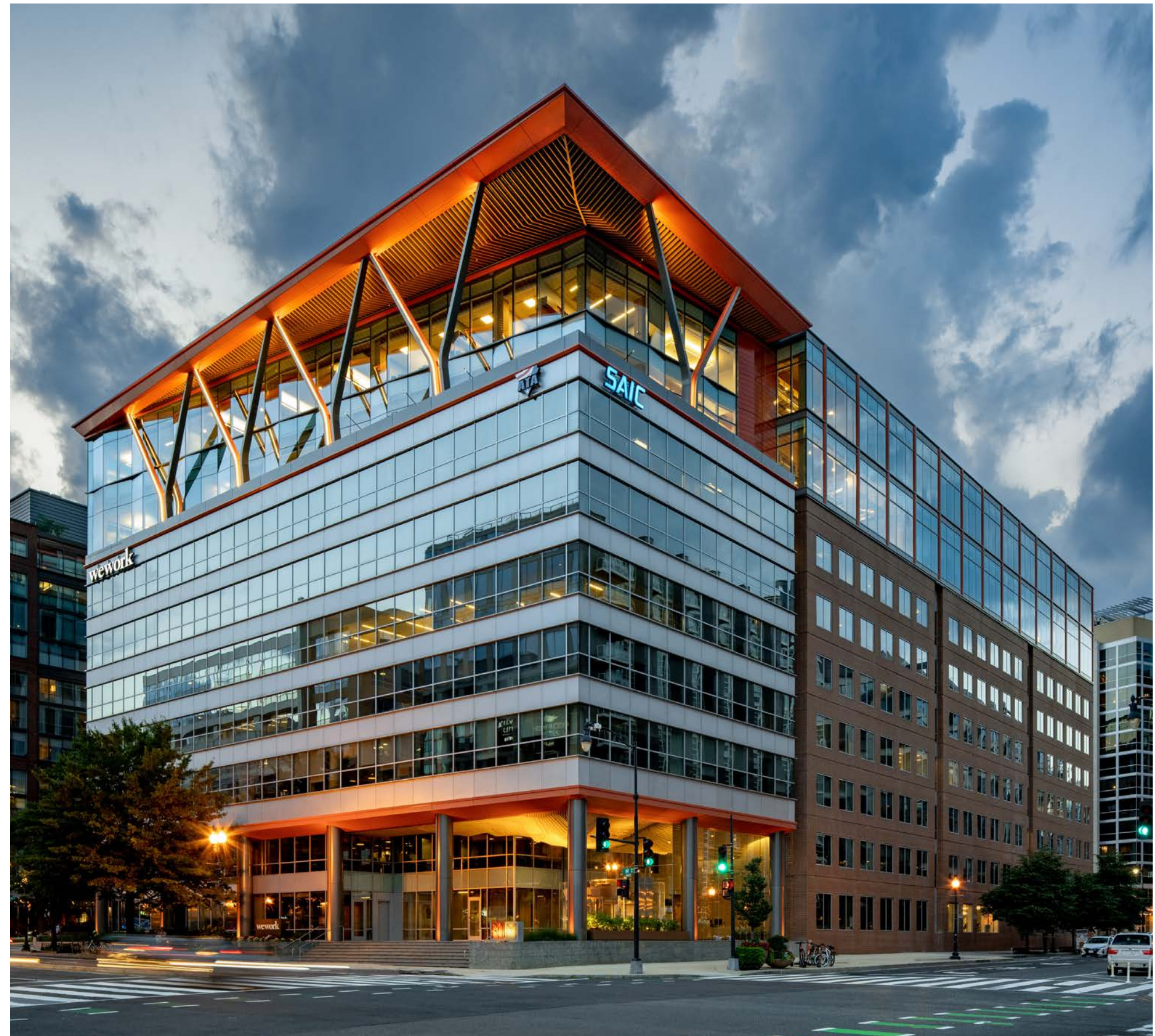
1: 80 M Street SE is the first commercial office space in Washington D.C. to incorporate a vertical mass timber extension
