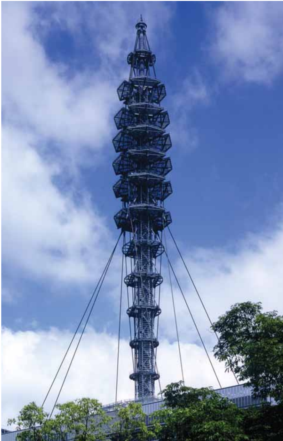
52. Close-up of the tower.
