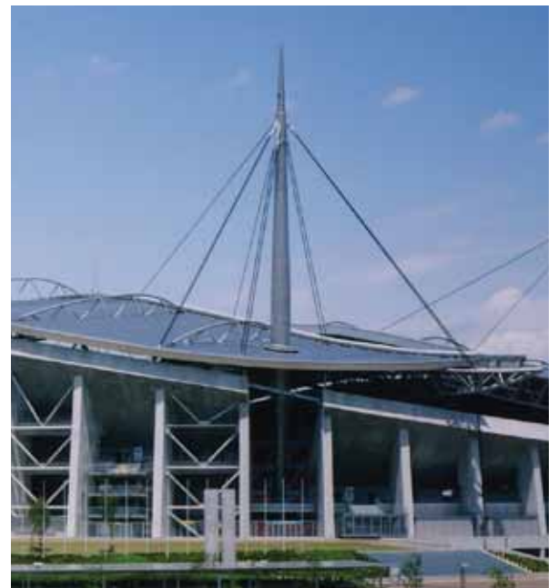
37. Mast and cables.
