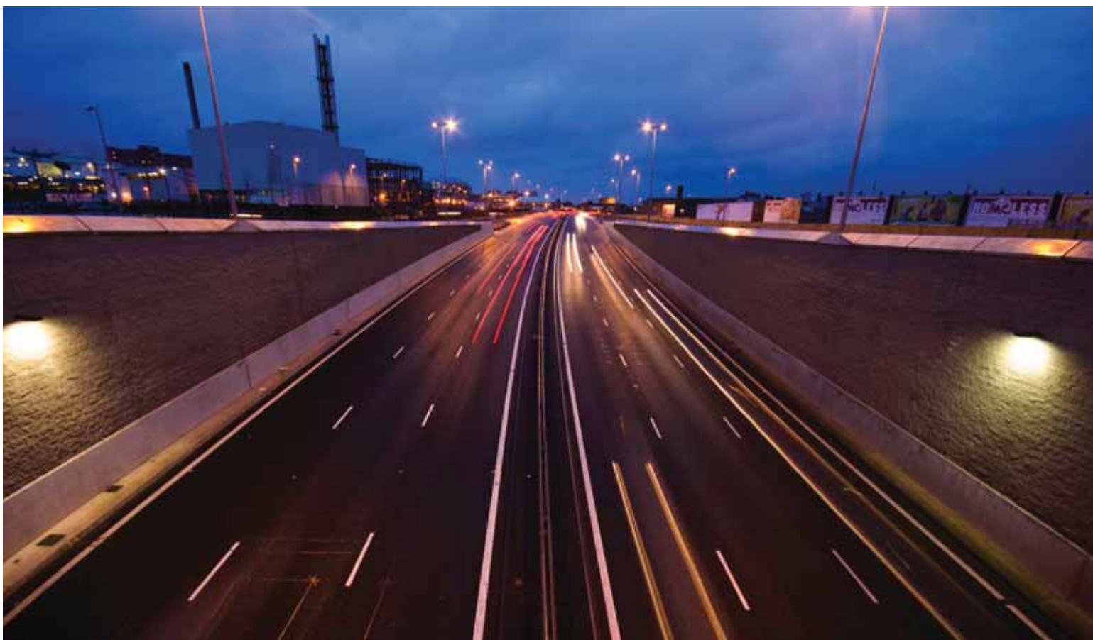
14. Broadway underpass northern approach.
