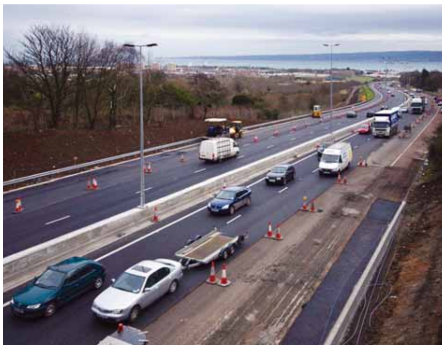
13. Scheme 3 under construction.
