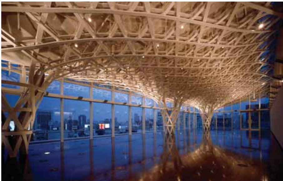
77. Free-form roof structure.
