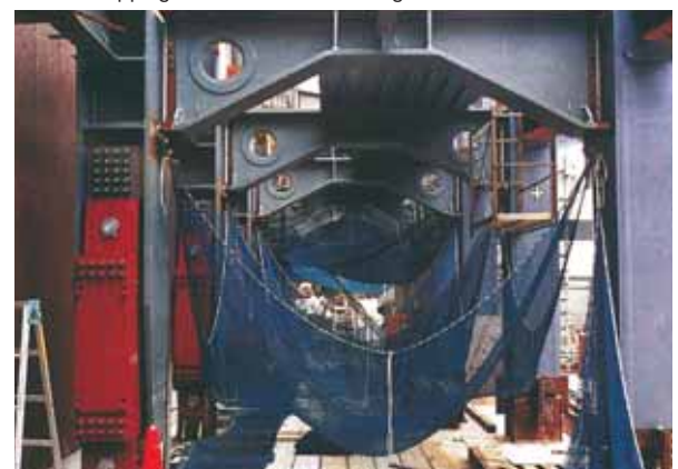
46. Stepping column and surrounding frame.
