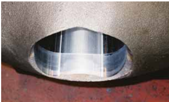
21. Interior of vertical connection before insertion.
