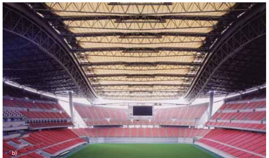
30. Interior view showing movable screen and retractable roof in (a) open and (b) closed positions.
