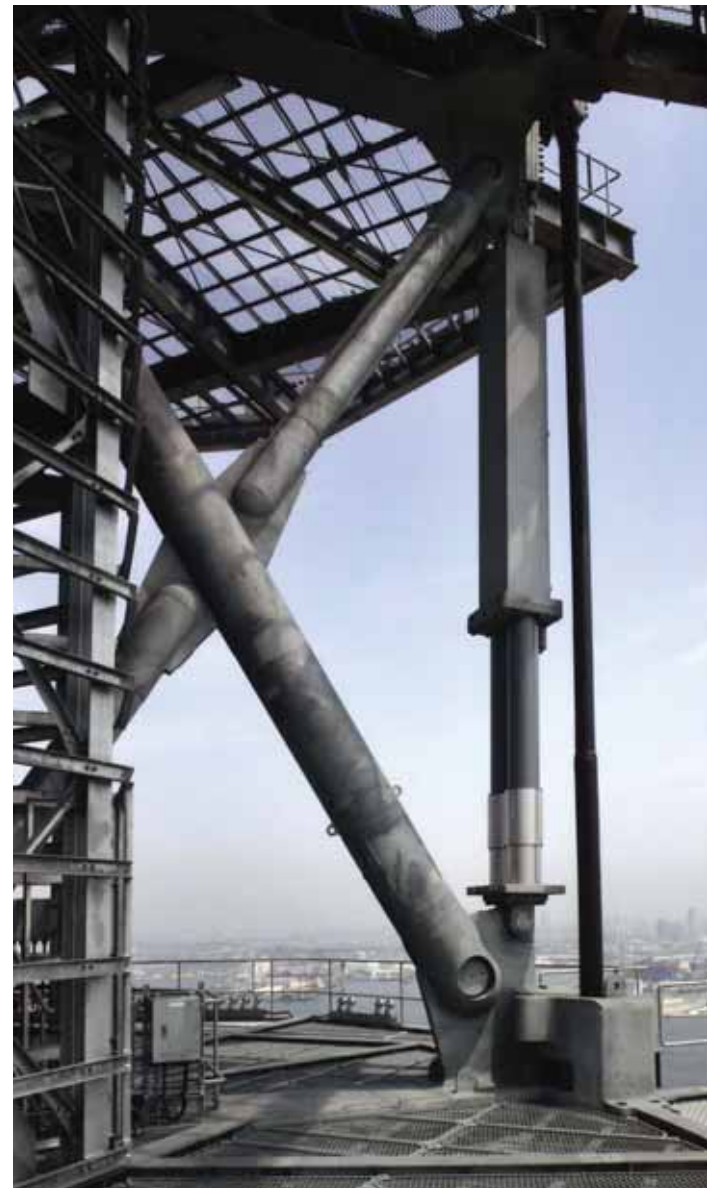
57. Rotational damping tubes.
