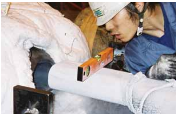
23. Commencing shrinkage fit (fitting time two seconds).
