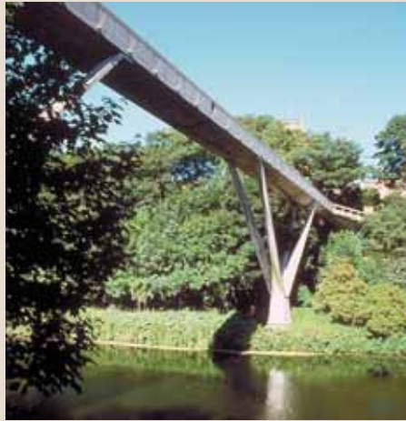
Kingsgate footbridge, Durham.
