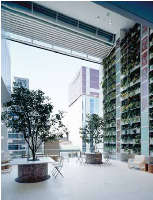
74. Fifth floor atrium with retracted glass exterior wall.
