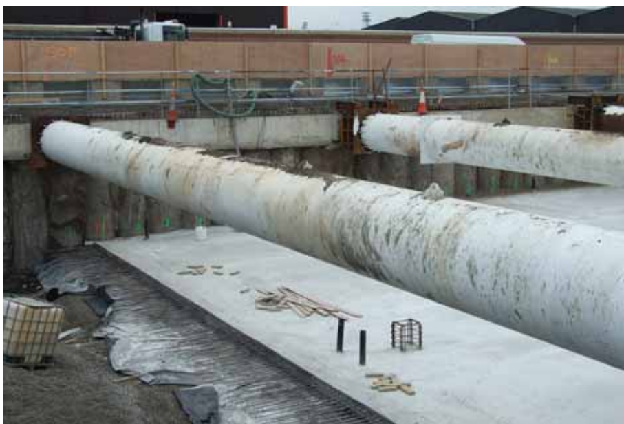
16. Temporary propping at Broadway underpass.
