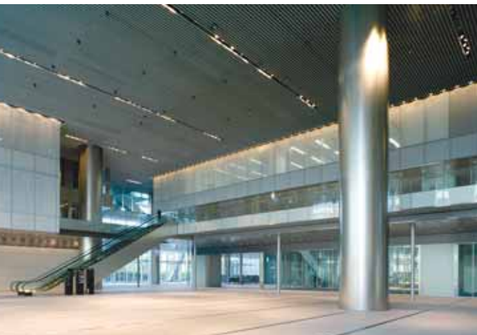
65. CFT internal columns.
