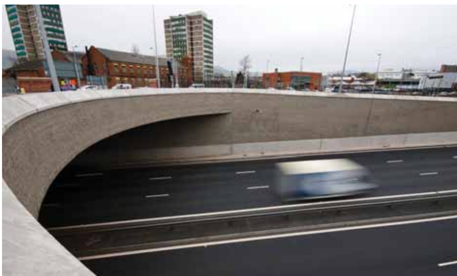
17. Broadway underpass northern portal.
