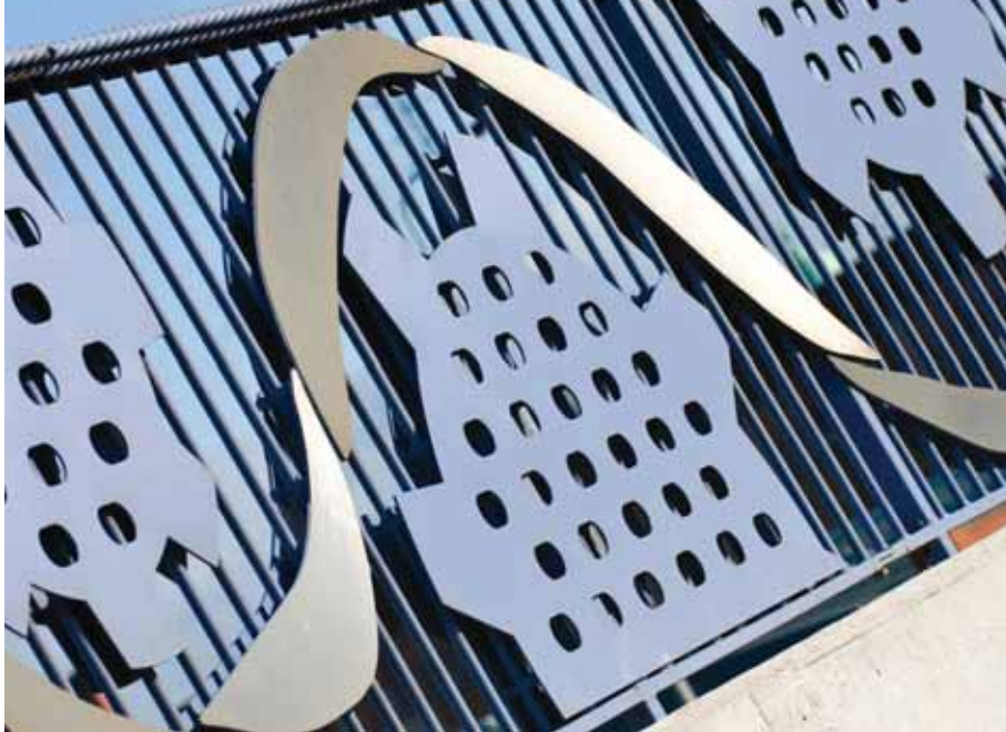
15. Parapet railings at Grosvenor Road junction.
