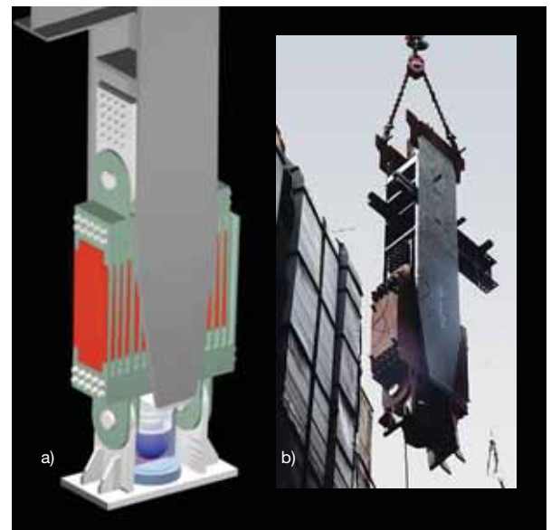
44. Rendering of stepping column detail (a) and stepping column being craned into place (b).
