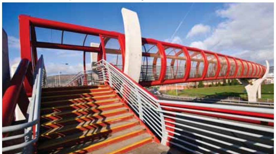
20. Exterior of the completed Roden Street footbridge.
