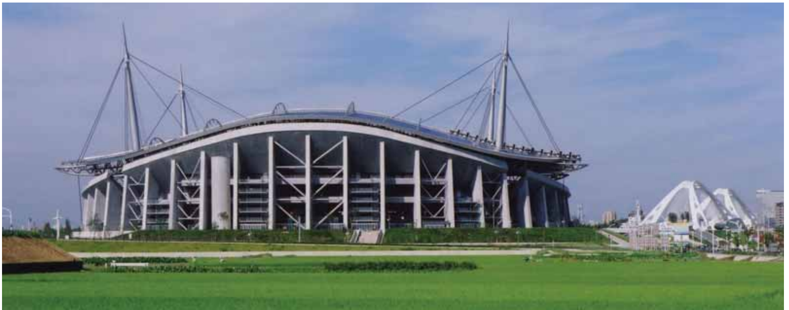
29. East side of exterior.
