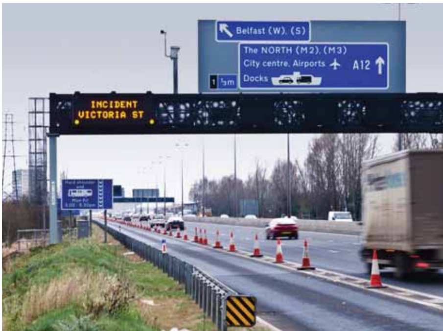
22. ITS in operation, north of Stockman's Lane junction.
