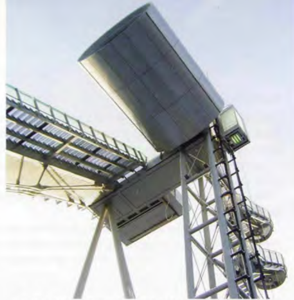
3. The capsule (warm-up room) and connecting bridge between tower and in-run.
