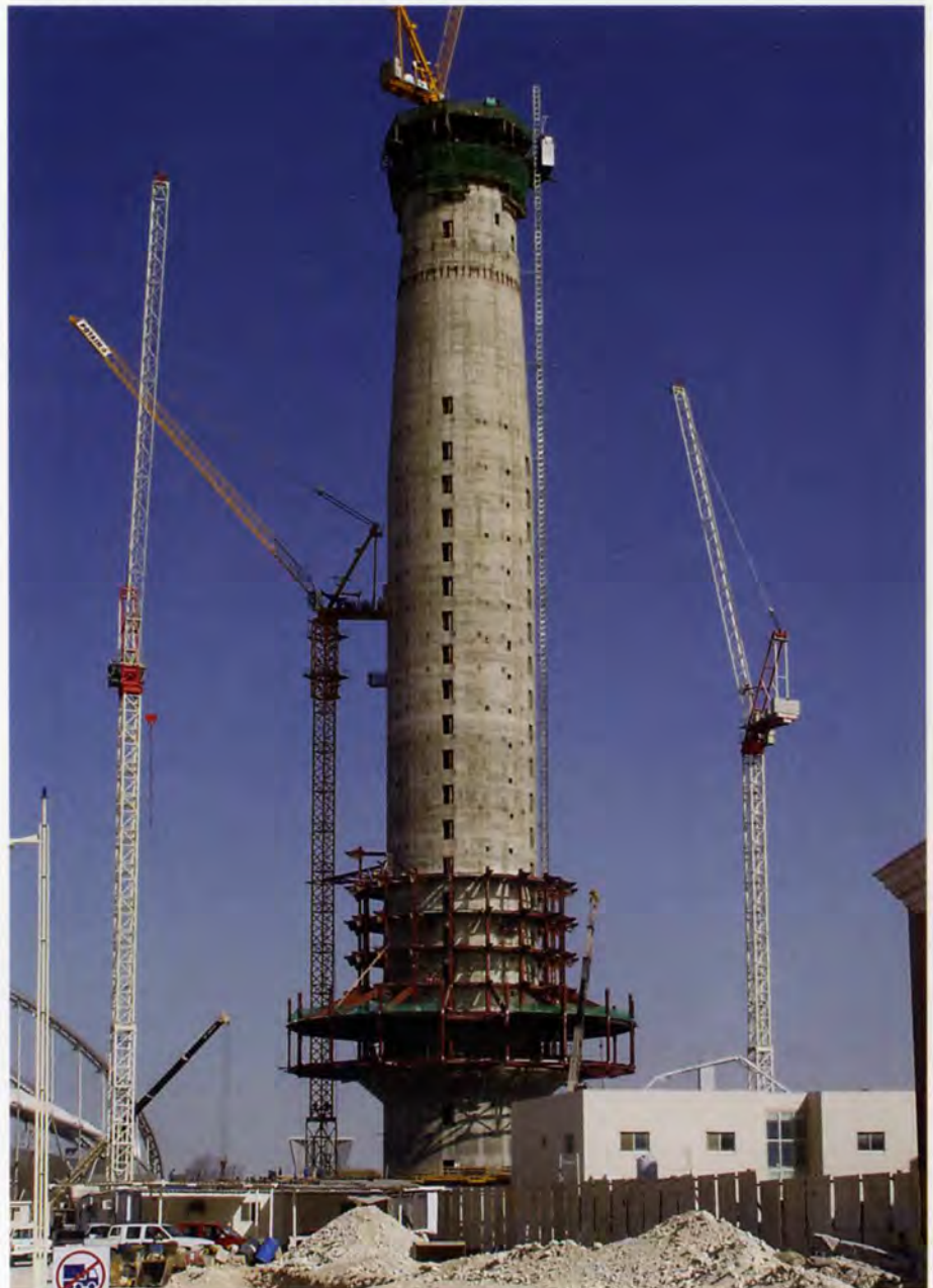
10. Concrete core under construction, March 2006.
