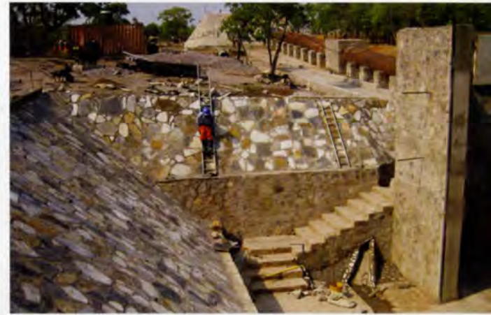
3. The powerhouse under construction.
