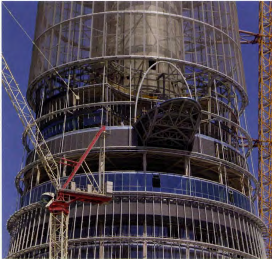
15. Swimming pool support truss in place.
