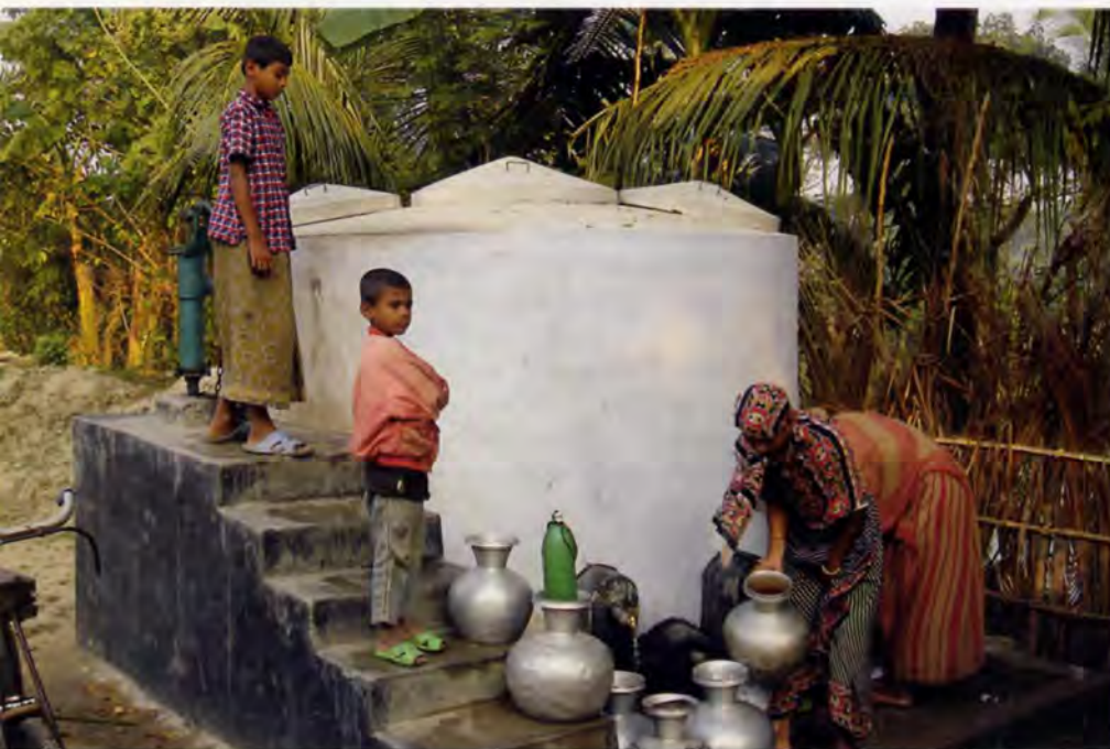
1. Pond sand filter.
