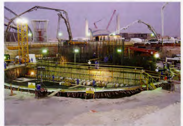
9. Pouring the 7m thick raft foundation.
