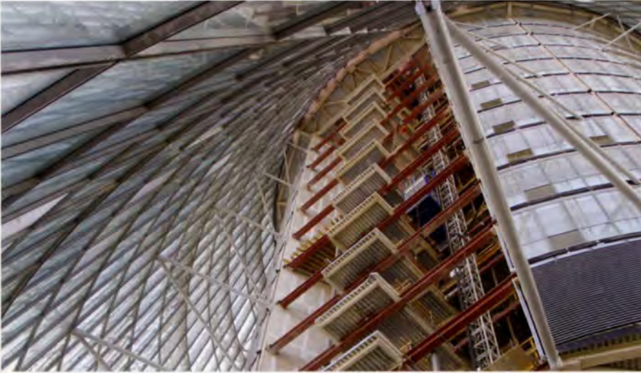
6. Hotel floors under construction behind glazed façade.
