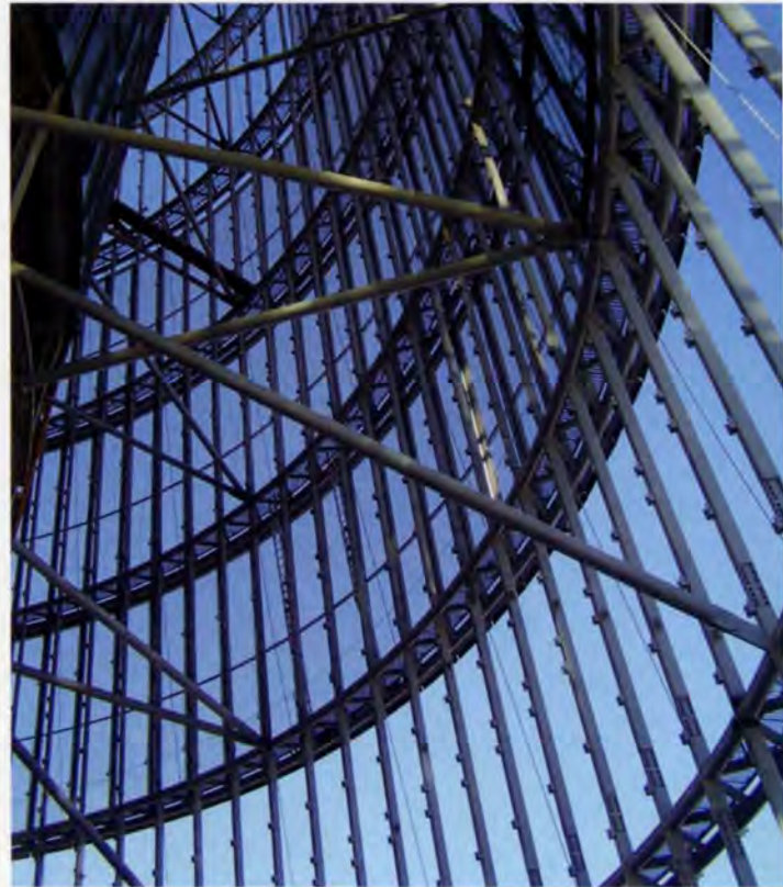
21. Detail of support for façade mesh.
