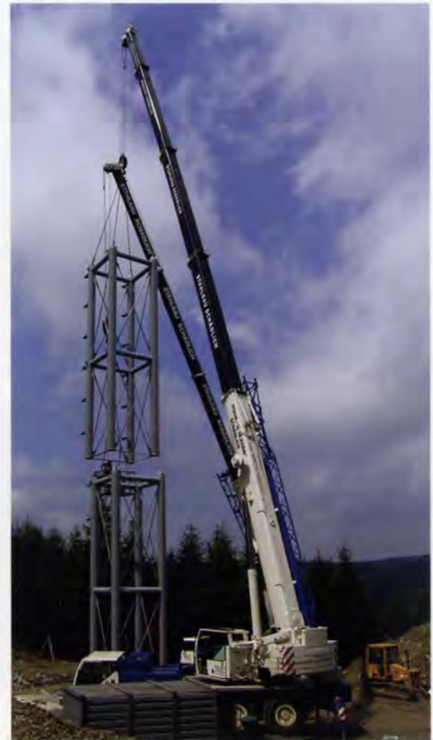
10. Assembling the second section of the tower.
