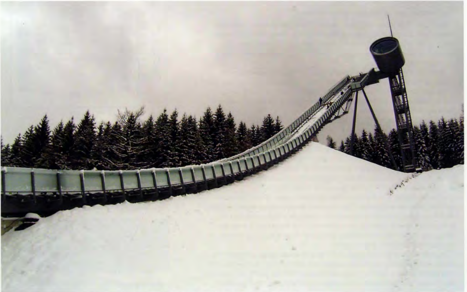
1. Overall view, showing the in-run, connecting bridge, and tower with the cantilevered warm-up capsule at the top.
