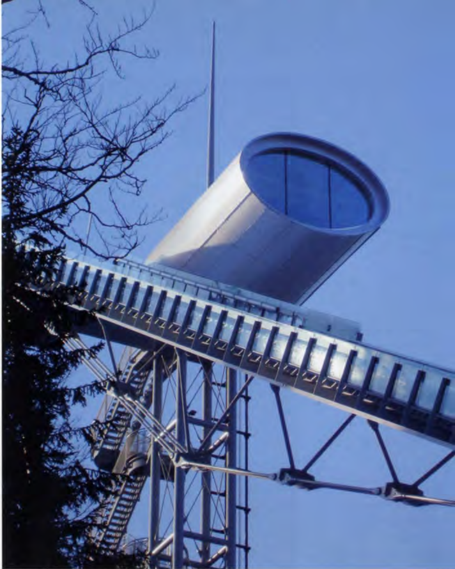
8. Side view of bridge support structure.
