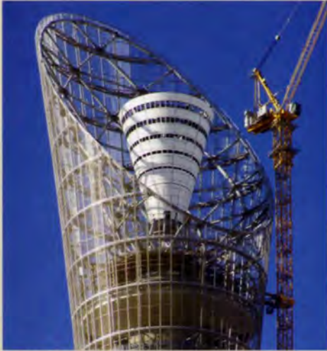
22. The diagrid and flame support, October 2006.
