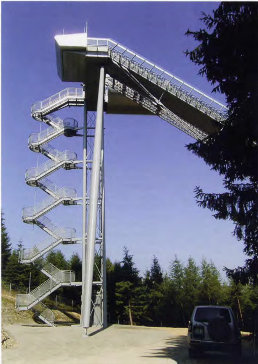
2 The tower with cantilevered staircase at the side.
