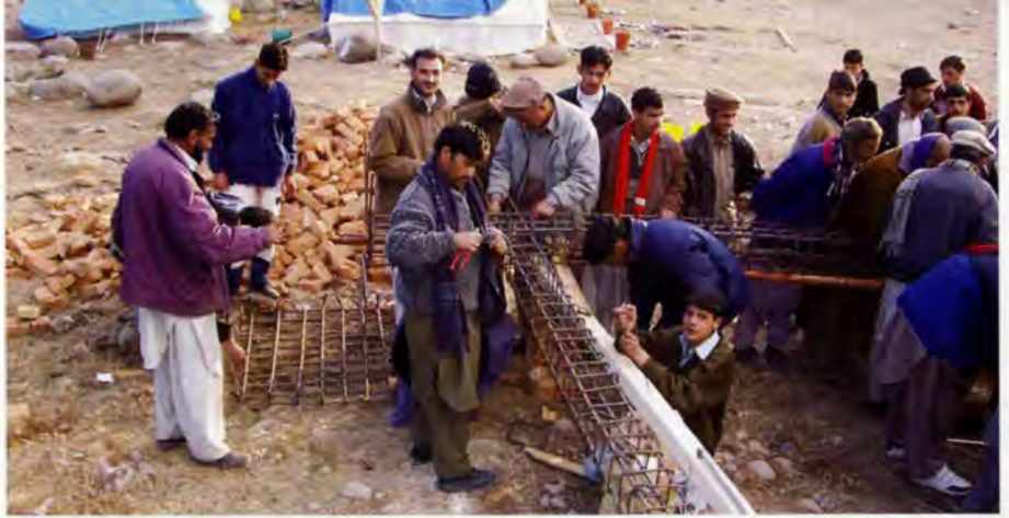
2. Steel fixing with seismic detailing.
