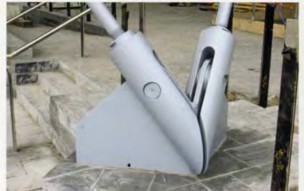
18. Ground anchorage of inclined roof tie.
