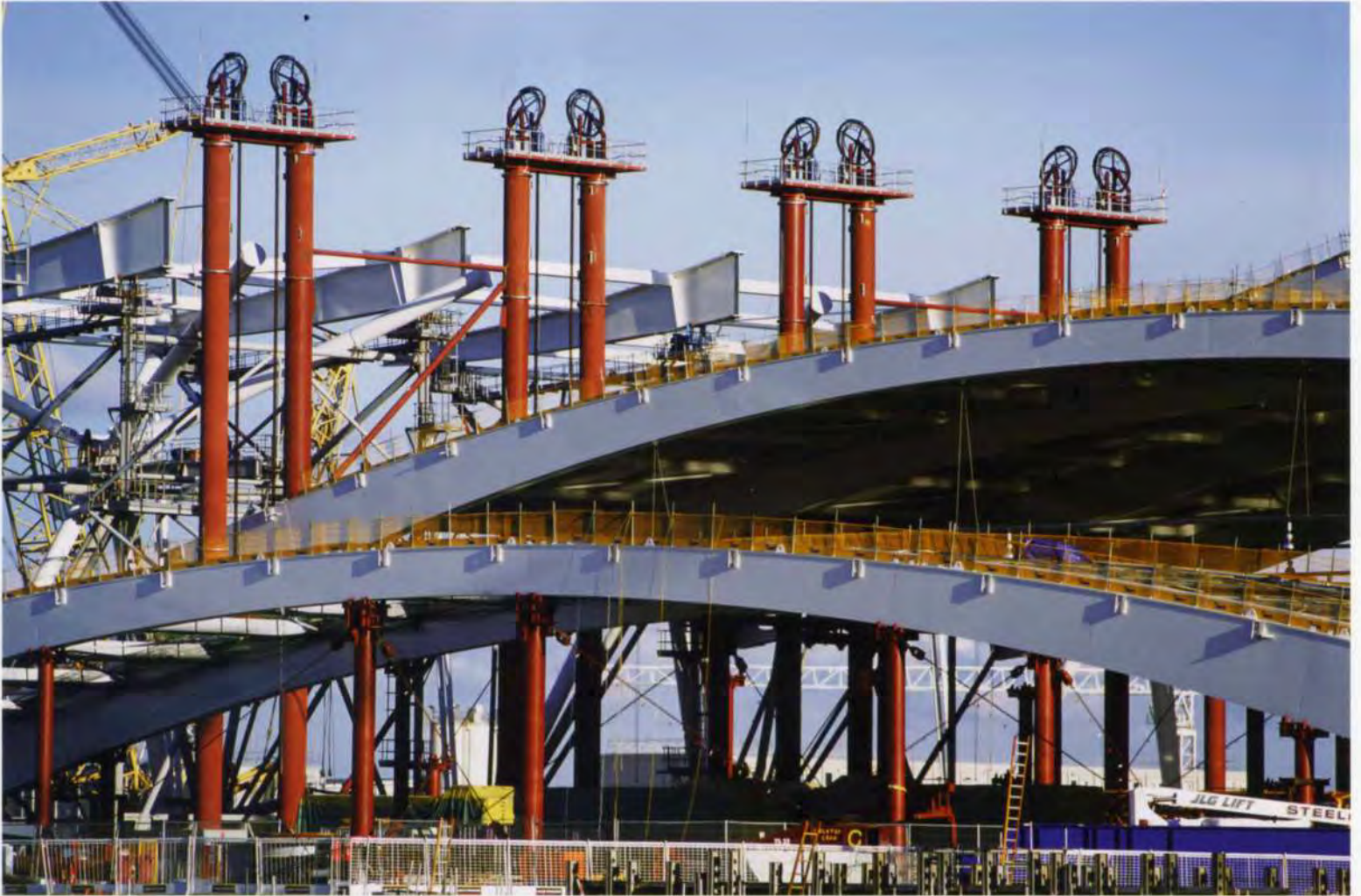
10. Jacking of roof elements.
