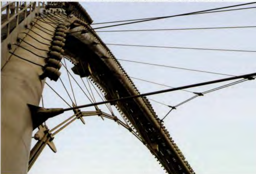
16. The lighting arch supports an array of sports lighting, as well as a loudspeaker array.
