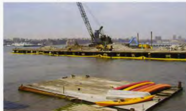
7. Pier 64 in Segment 5 cleared of its old shed.
