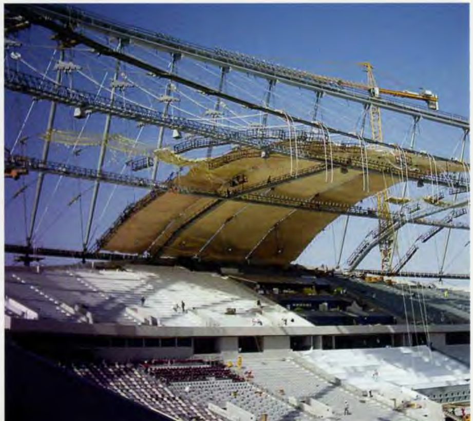
14. The roof being erected.
