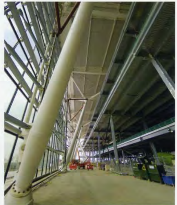
2. Dramatic full-height circulation space.
