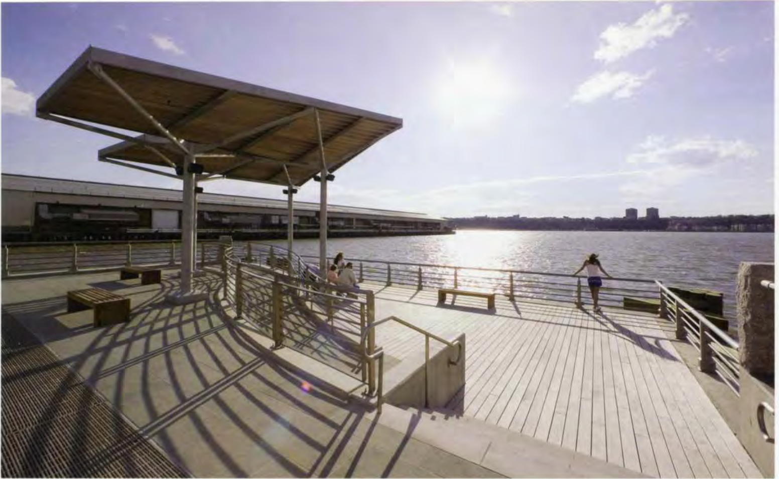
8. Pier 95 at Clinton Cove Park, Segment 7.
