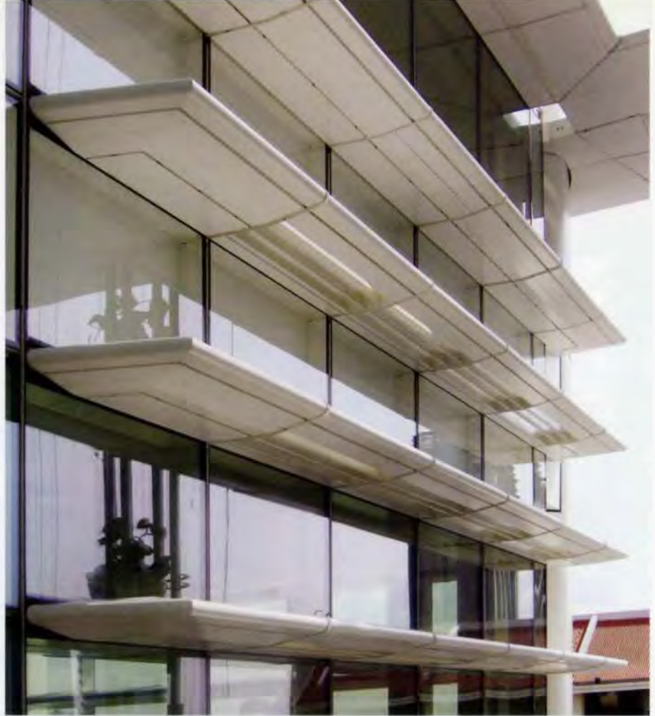
13. Exterior sunshades in place.
