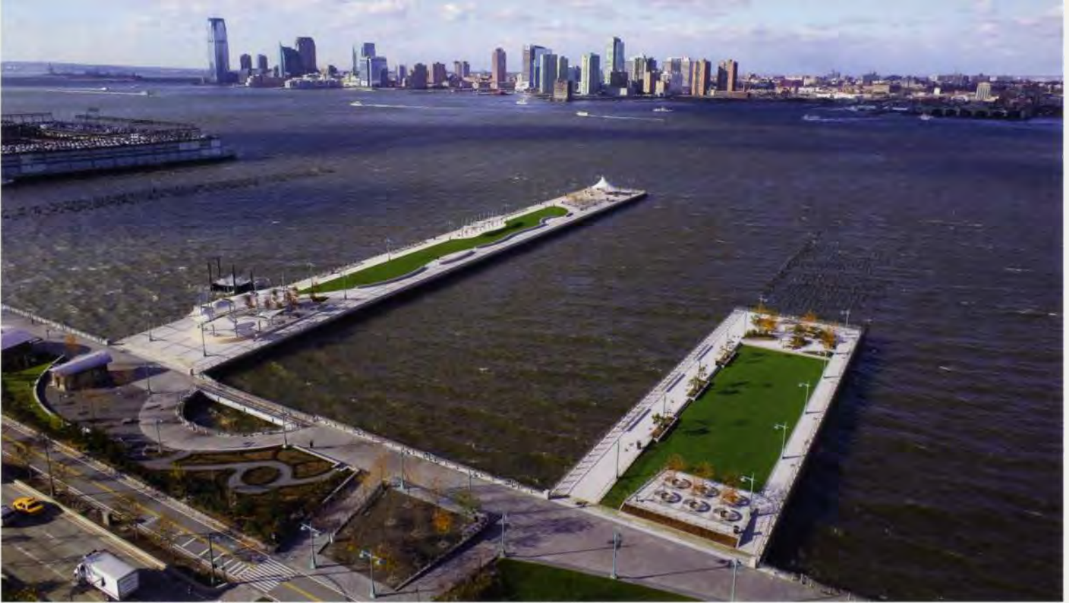
4. Piers 45 (left) and 46 in Segment 4, looking west to New Jersey across the mouth of the Hudson.
