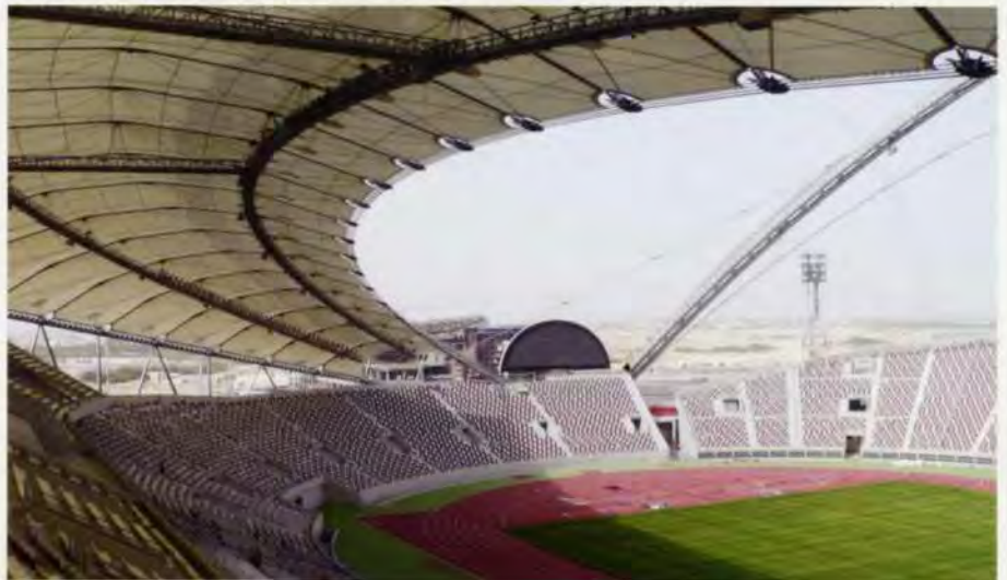
9. Detail of PTFE fabric membrane roof.
