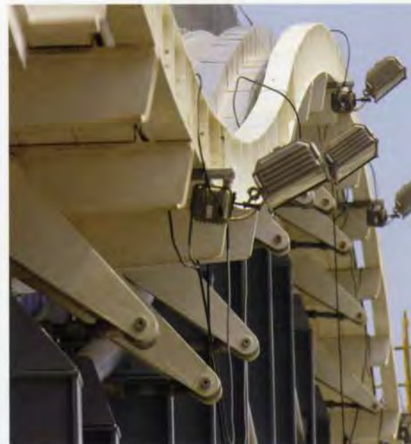
7. Joint at head of south façade.
