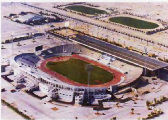
2. The stadium before upgrading.
