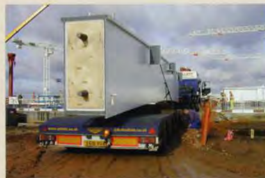
8. Rafter section arriving on site.
