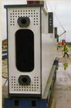
23. Close-up of shear key.
