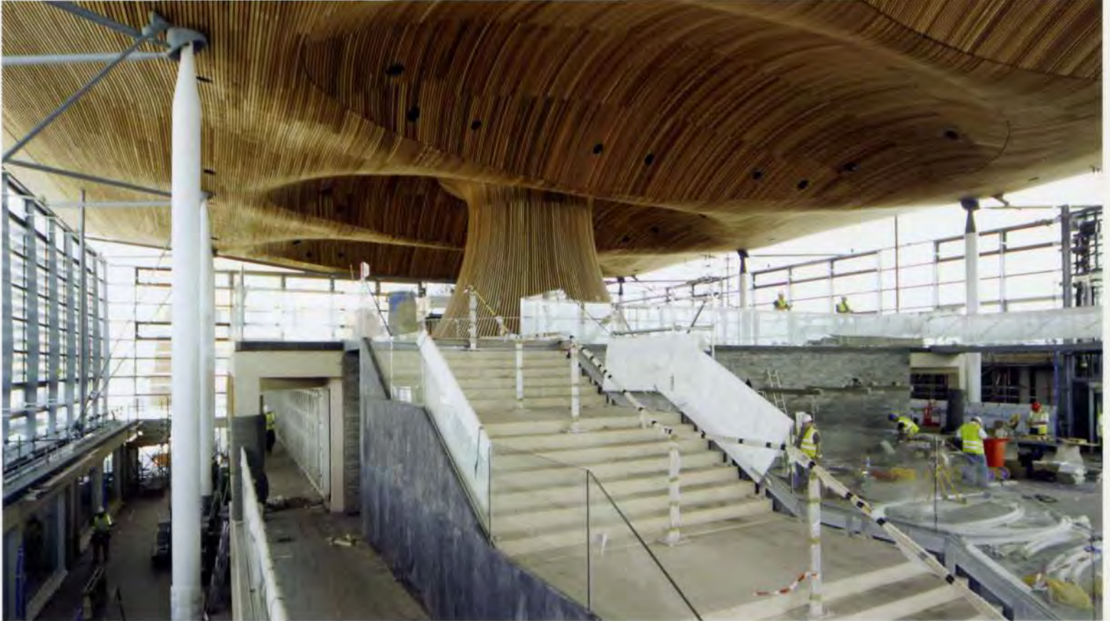
5. Canyon and public entrance under construction.
