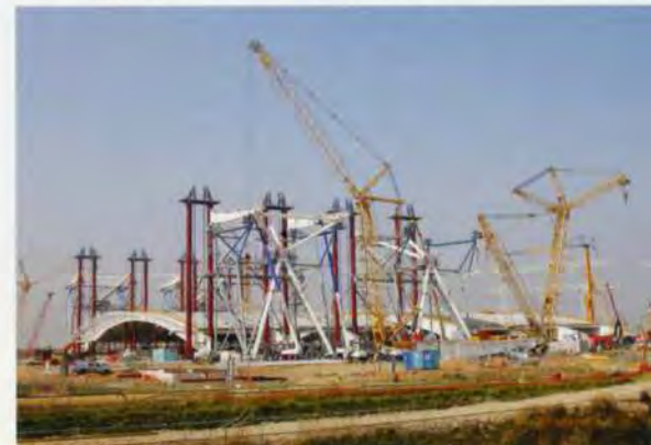
9. Roofing material in place prior to erection.
