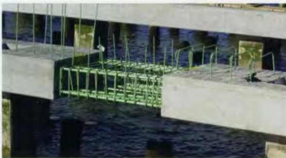
13. Precast pile caps at Pier 84, November 2004.
