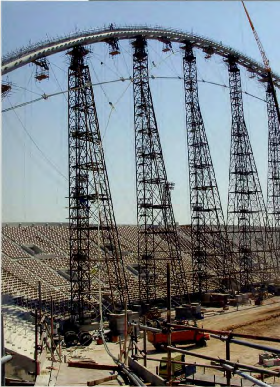
15. Erection: cables prior to stressing wing cable on the lighting arch.
