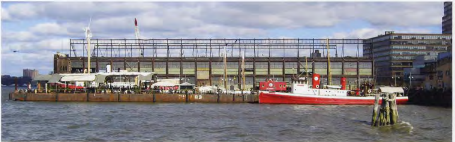
11. The two-storey shed on Pier 64 before it was cleared.
