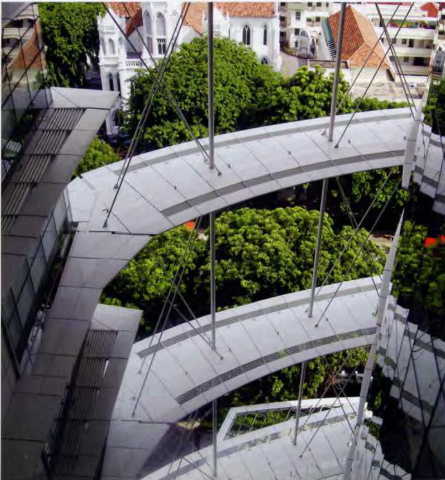
17. Sunshades in position in the laneway.
