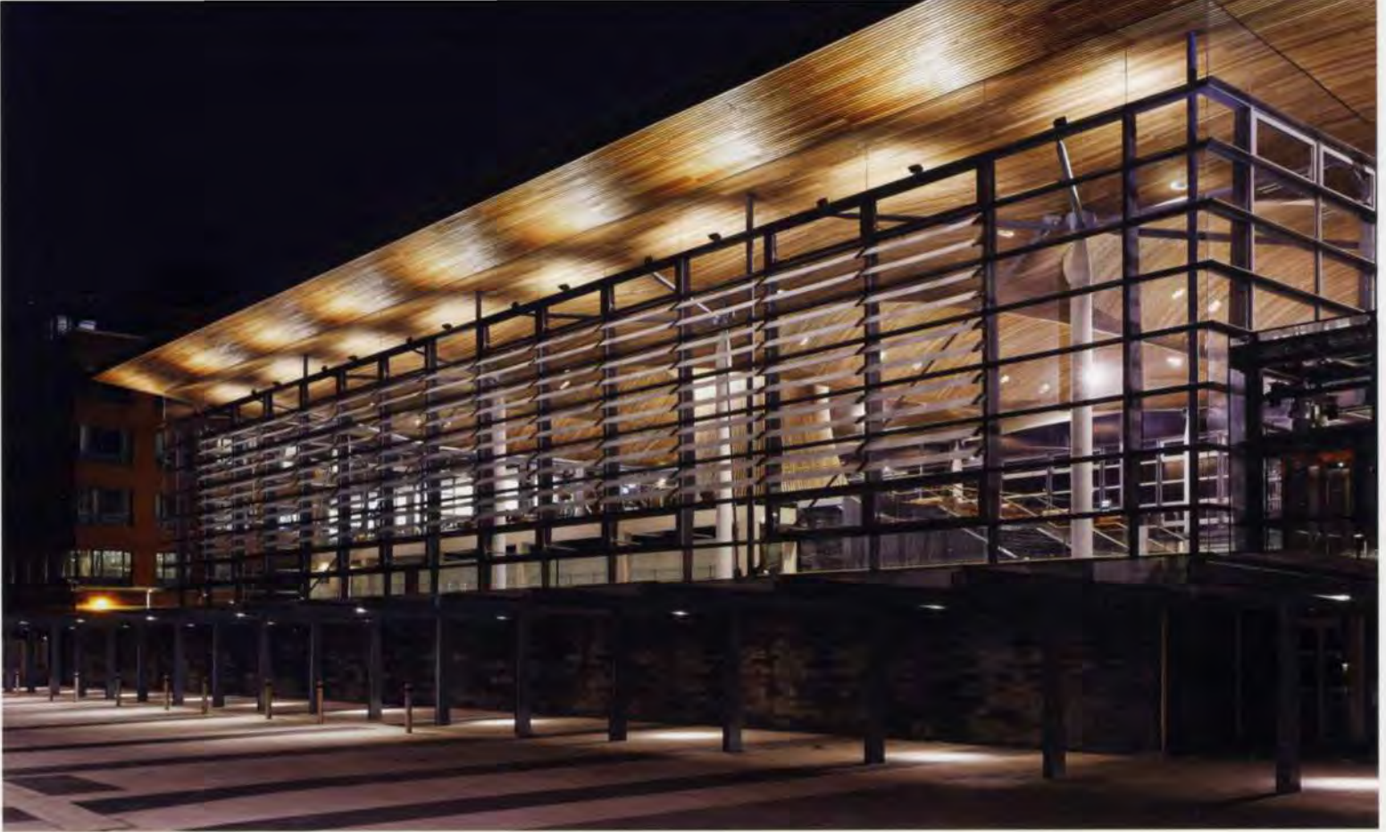
22. The glazed façade: side view at night.
