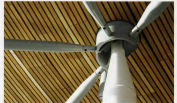
17. Roof column head.
