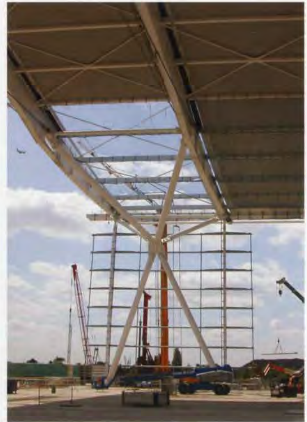
13. Bracing in roof plane and abutments.
