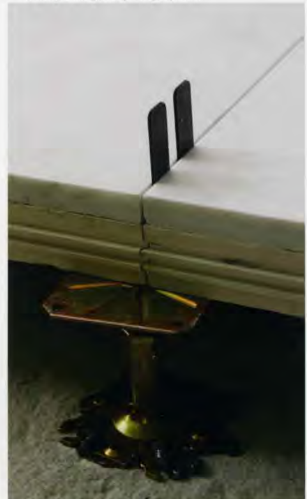
1. Tongue and groove jointing of panels.
