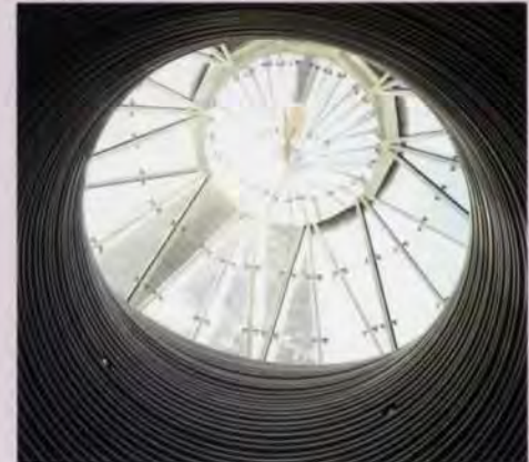
21. Underside of mirror cone in lantern.
