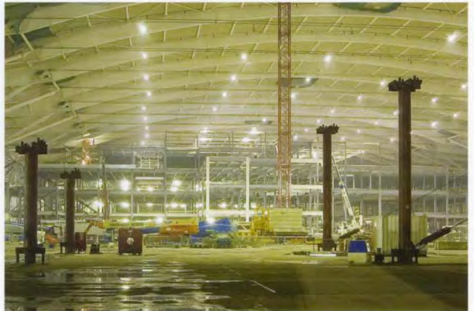
11. Central section clad and prestressed, May 2004.
