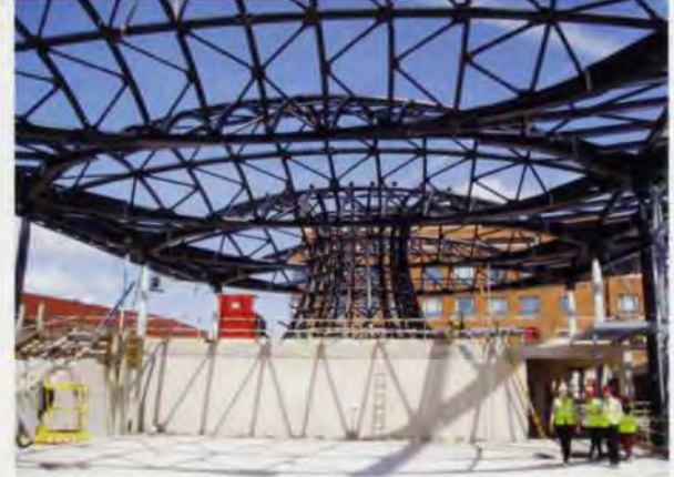
20. The roof under construction.
