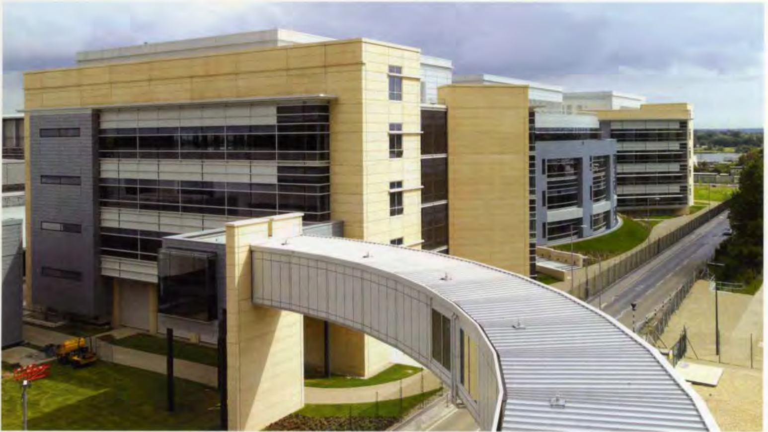
13. Connector link bridge and western elevation.
