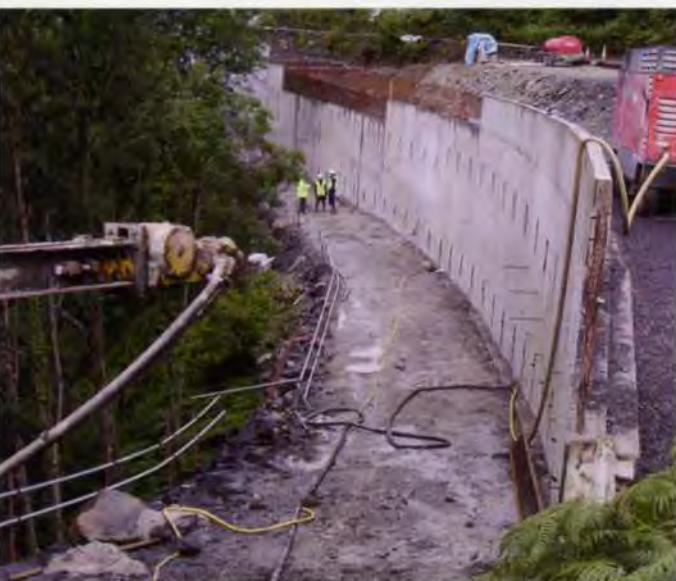
5. Anchored panel wall.
