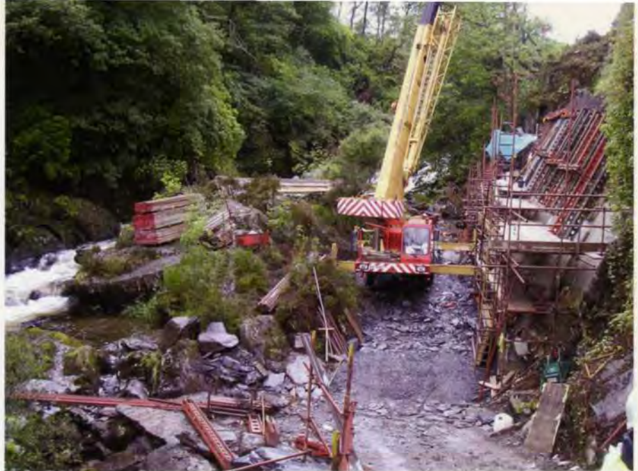
6. Constructing retaining wall No. 6 at Pont-y-Pant.
