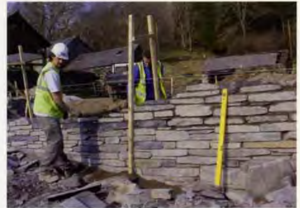
3. Constructing boundary walls.
