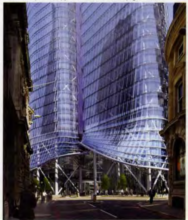
3. Complex canopy entrance to the Bishopsgate Tower.
