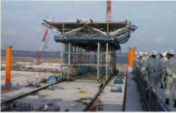
13. The first roof truss modules in position.
