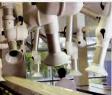
8. Laboratory air extractors.
