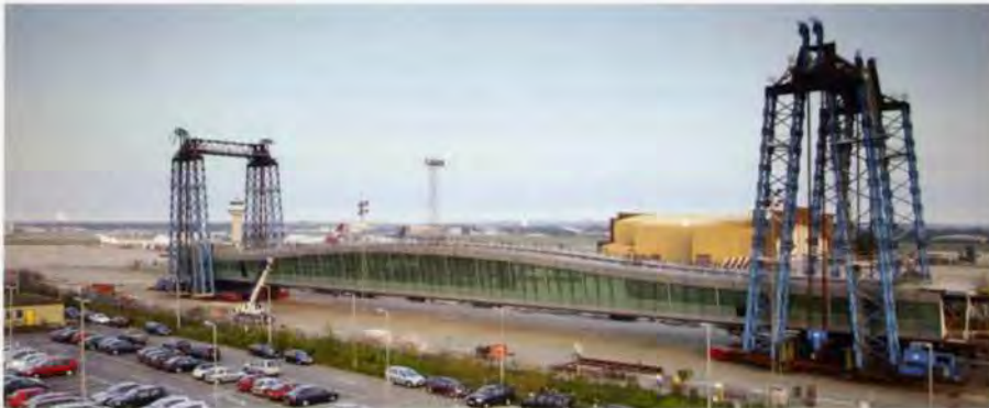
9. The 164m-long deck section with the lifting towers, on the transporters at the prefabrication yard.
