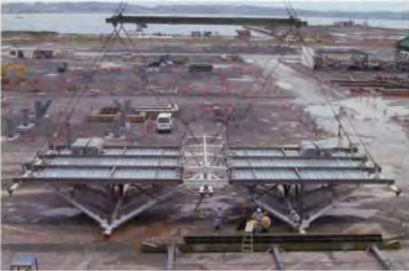
14. Roof truss module ready to be raised.
