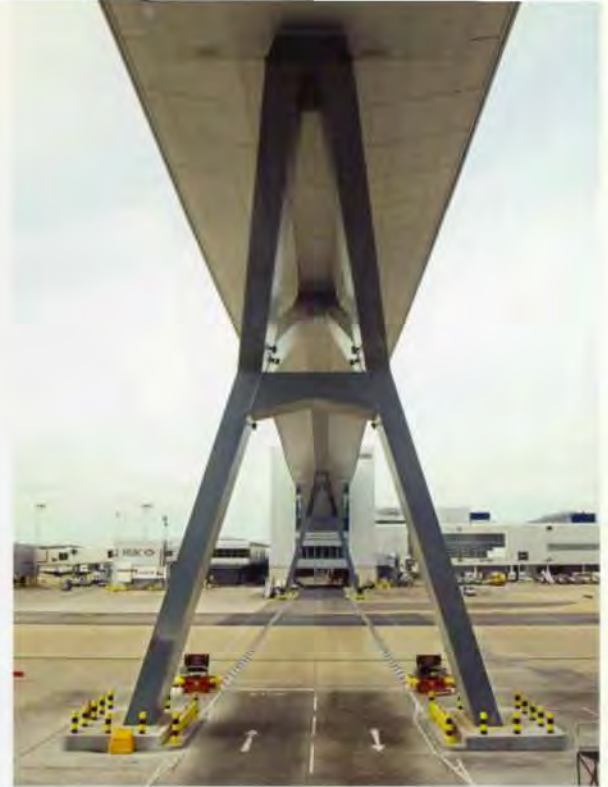
11. In their final position, the scale of the supporting columns is clearly apparent.
