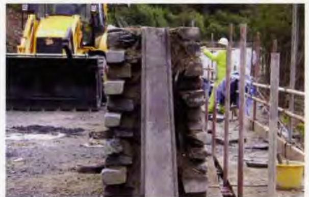
4. Stone-clad containment parapet.
