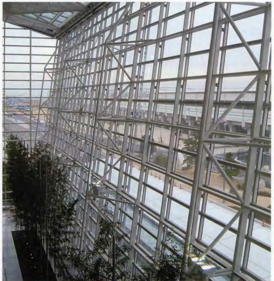
15. Façade support structure at the 'welcome garden'.
