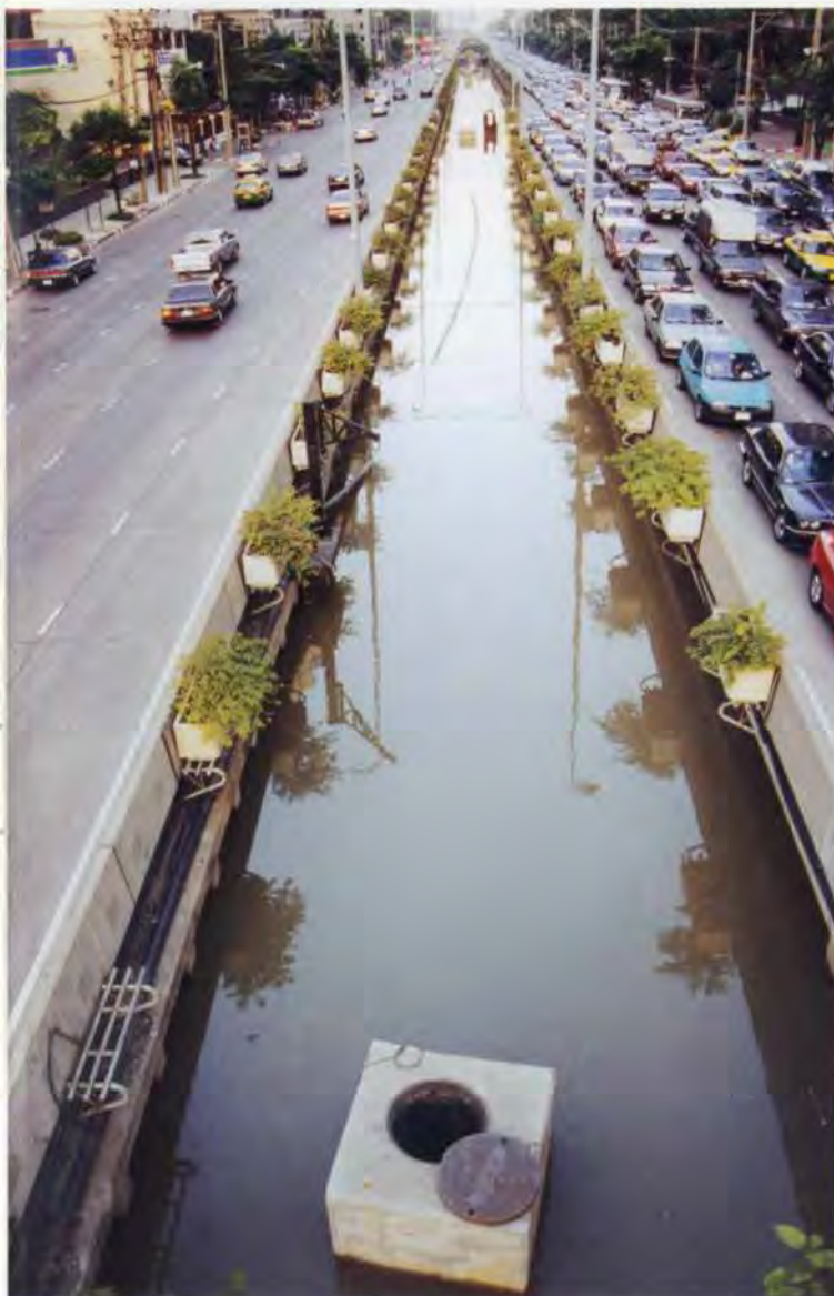
2. Khlong Sathern, with manhole in the foreground indicating sewer routing.
