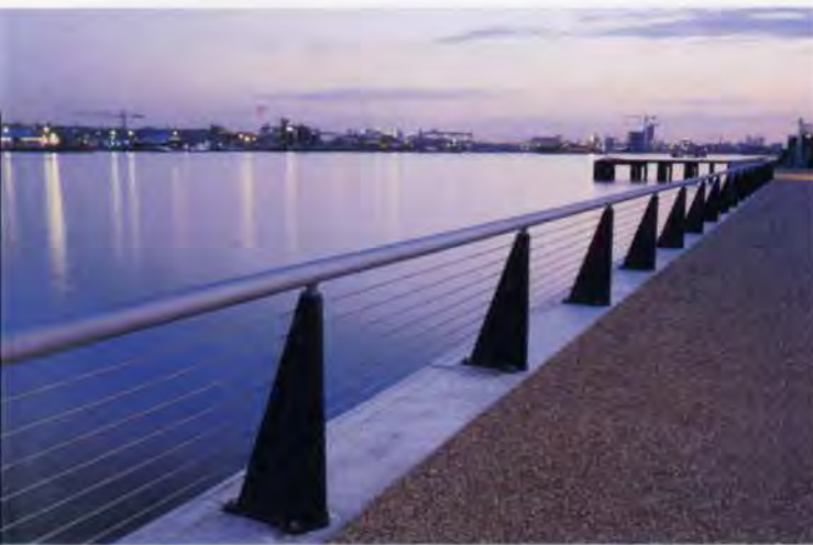
6. View along the riverside walkway.
