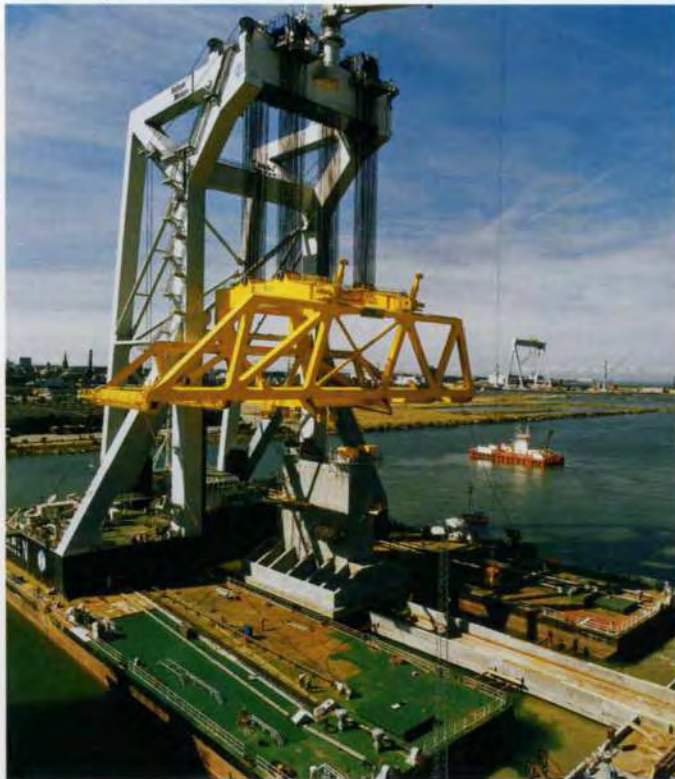
14. Svanen lifting caisson at the Malmö yard.
