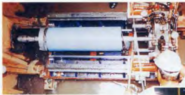
3. Direction drilling for small diameter pipe.
