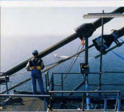
24 above: Placing the main cables.
