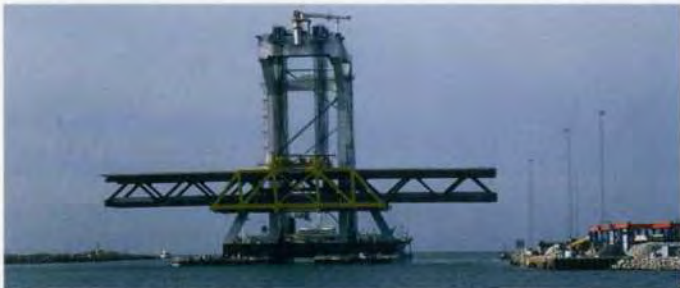
16 below: Approach girder being transported to bridge line by Svanen.
