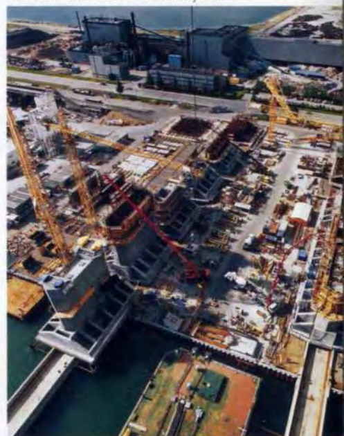
4. Caissons were cast at the Malmö yard.
