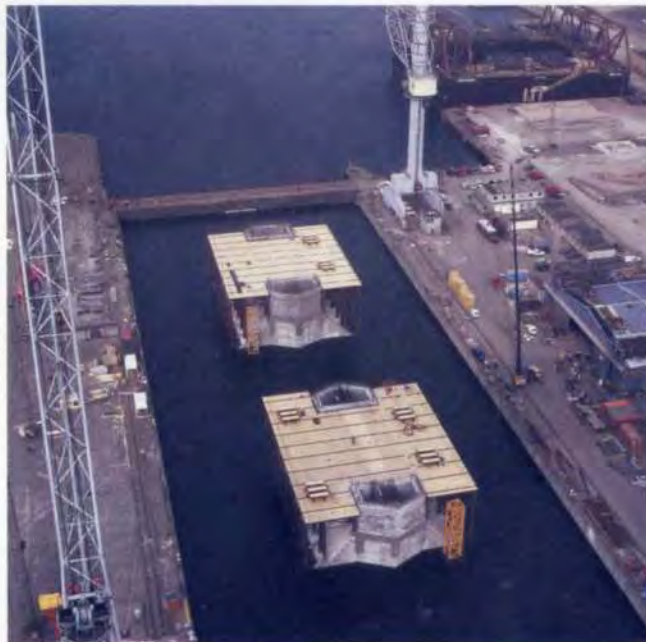
5. Caissons for the pylons were cast in Malmö in dry dock.
