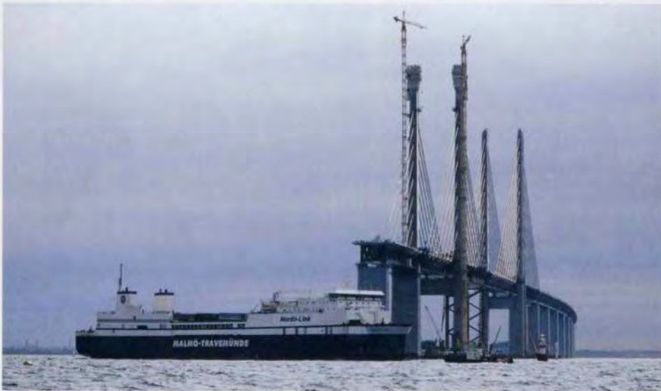
22 left: The original navigation channel was used until main span was completed.
