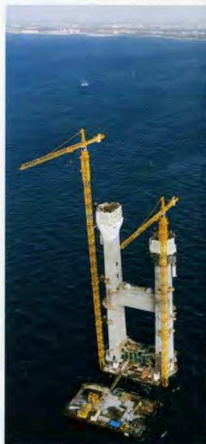
12 above, and 13 below: The main pylons were cast in situ.
