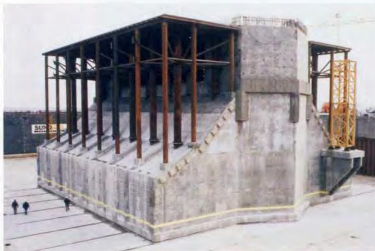
5. Caissons for the pylons were cast in Malmö in dry dock.
