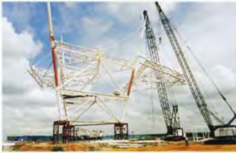
5. Large sub-assembly of node roof being lifted into place in the temporary construction yard.
