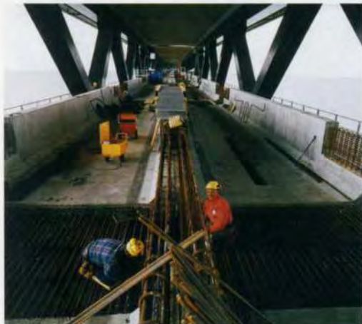
18. Completing the railway deck in approach bridge.
