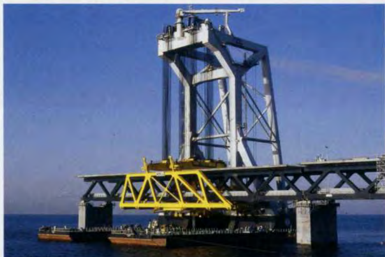
17 right: Svanen placing approach girder.
