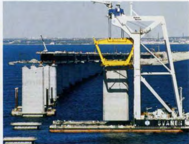
15 below: Svanen placing pier shaft.
