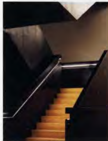
14. The main stair links all concourse levels and incorporates sheet steel and unfinished oak treads. Lighting is concealed above the stained oak handrail.
