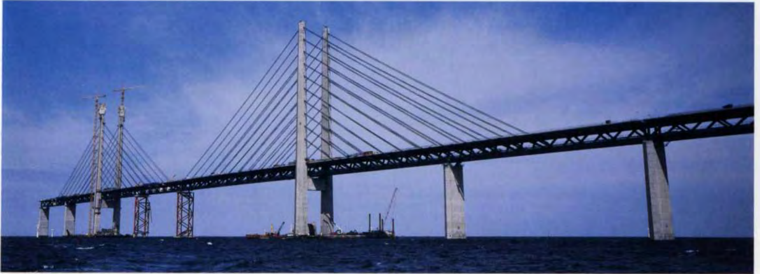
21 above: The main span nearing completion.
