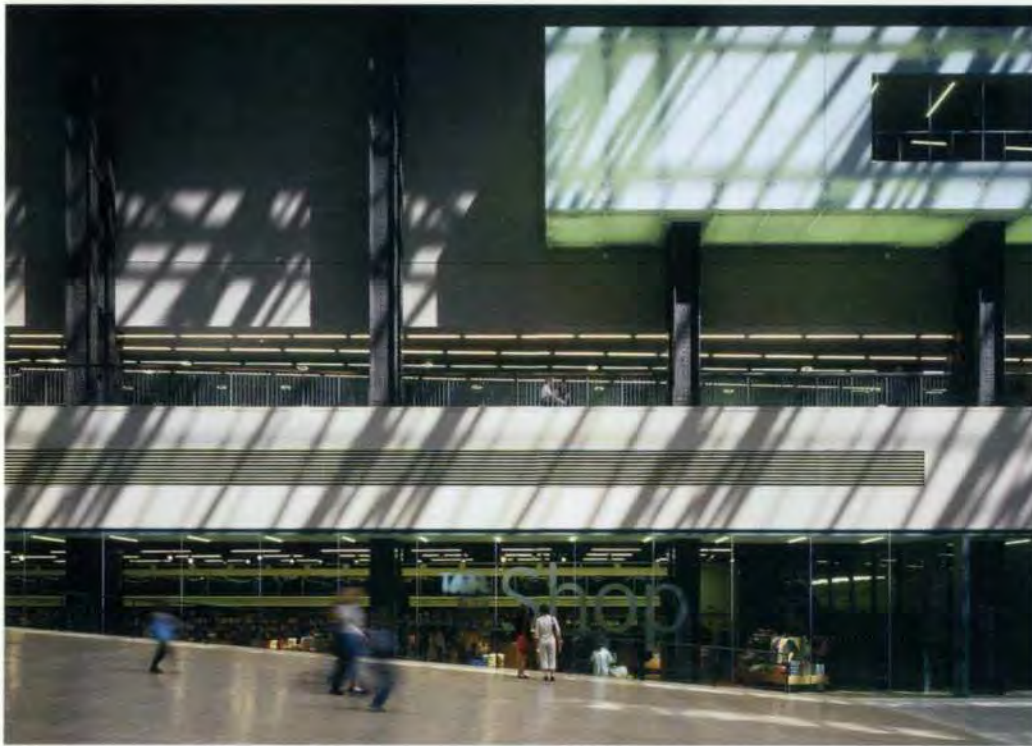
2. Exhaust air from the galleries is used to moderate the Turbine Hall environment. Glazed bay window enclosures provide lighting to the Turbine Hall.
