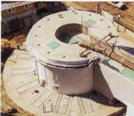
9. Inlet pumping station.
