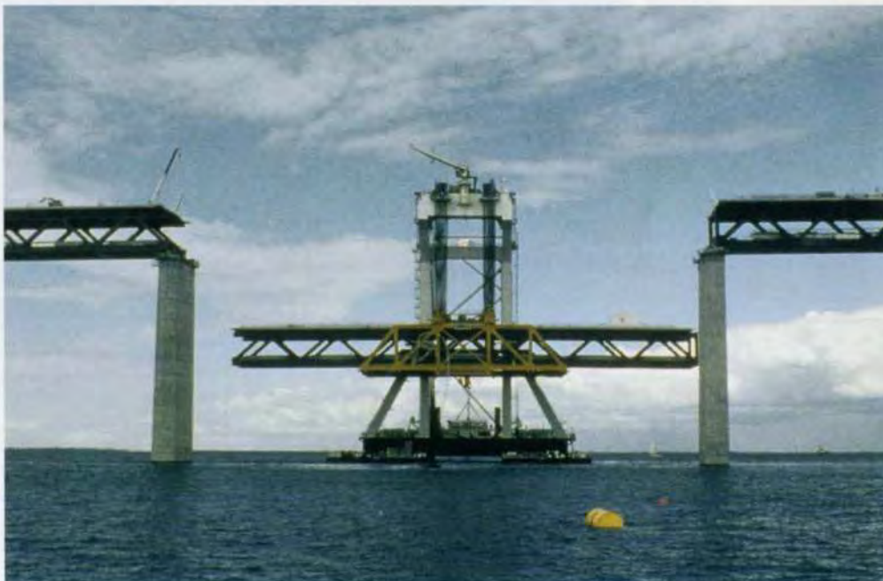
19. The last girder is placed.
