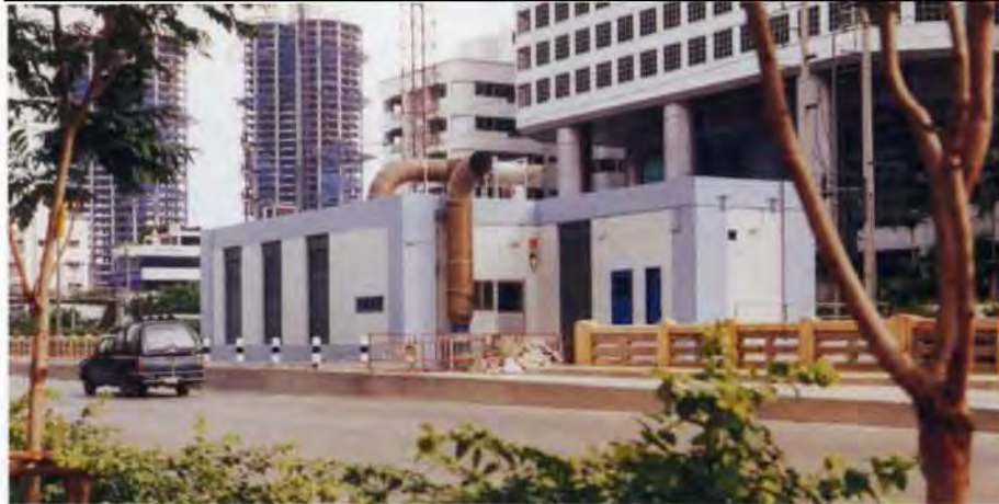
6. Collector system pumping station built over khlong.
