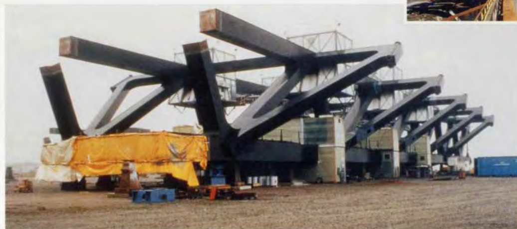
11. Main span girders were fabricated in Karlskrona.
