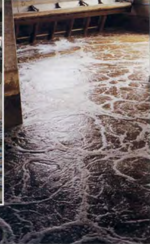
14. Treatment basin in aeration cycle.
