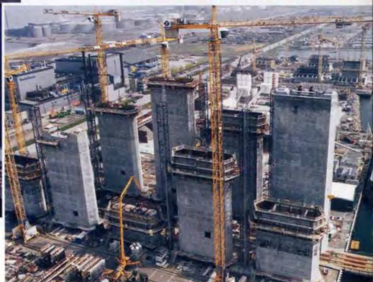
3. Pier shafts were cast at the Malmö yard.
