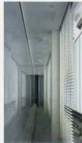
5 right: The interstitial space of the light beam, showing feature lighting and lighting control blinds.
