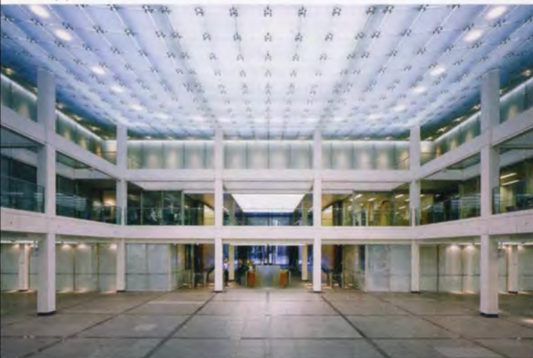
8 (a-d). Believed to be the largest installation of its kind in Europe, the 'artificial sky' is a 576m 2 translucent bowl formed of individually suspended glass tiles.
