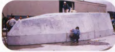
11. Shroud at the precasting yard.
