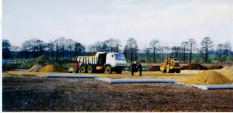
13. Poland site preparation.
