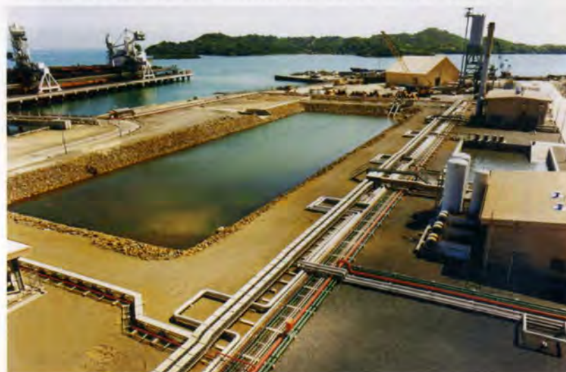
10 below: Site-wide services, including electrical distribution, potable water, seawater, fire-fighting, etc.
