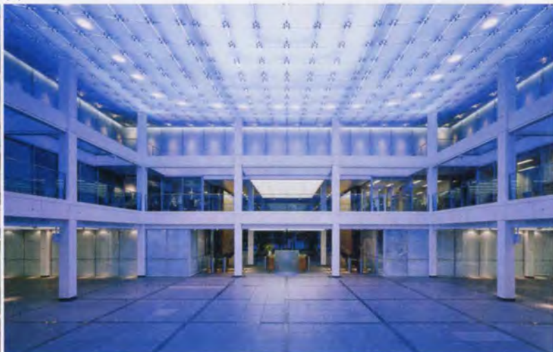
8 (a-d). Believed to be the largest installation of its kind in Europe, the 'artificial sky' is a 576m 2 translucent bowl formed of individually suspended glass tiles.
