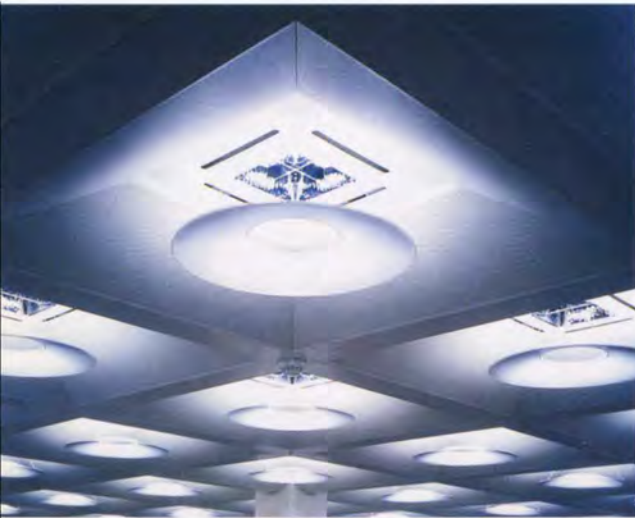
5. The specially designed luminaires for the dealer floor combine the recommended provision for VDU use with an uplit ceiling from a single standard fitting. This increases the apparent height of the space and avoids the gloomy interior that can result from sole use of a Category 1 luminaire.
