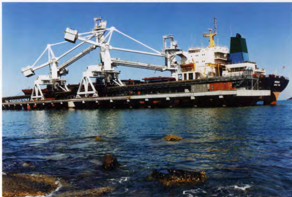
3. Coal unloading jetty.
