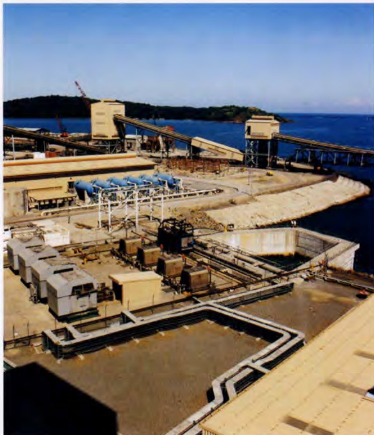
8. Cooling water intake and pumphouse.
