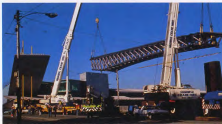
7: Installation under way.
