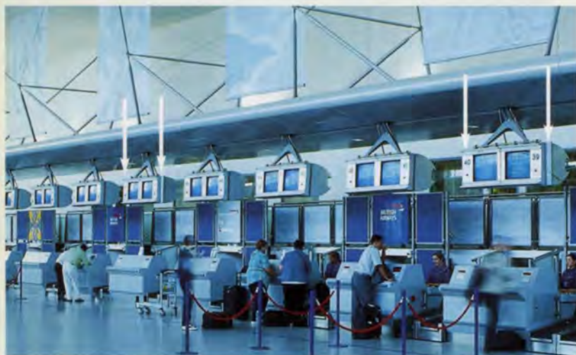
11. Completed T1 BA check-in hall showing Penton MC-402 column loudspeakers on the row of monitor housings (arrows indicate typical positions.)
