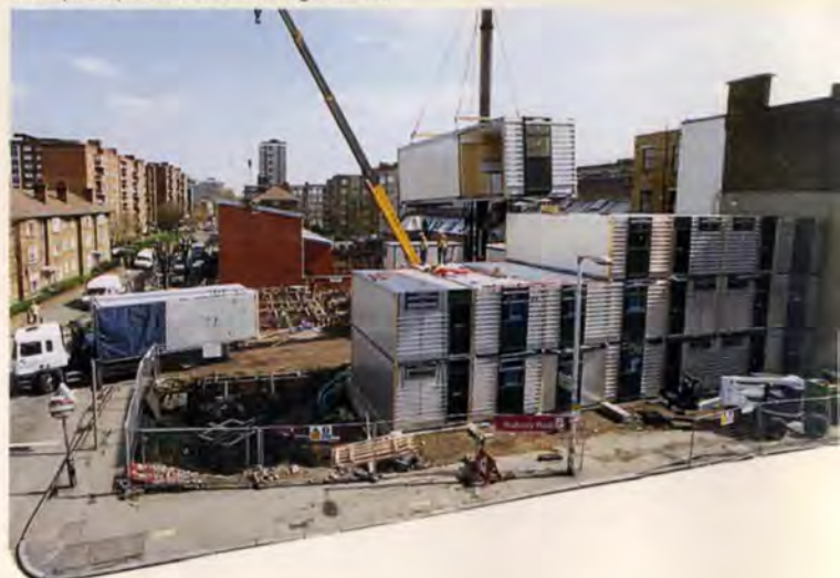
6. Example of paired modules being installed.
