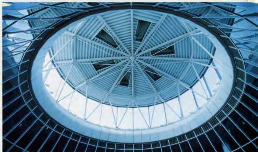
13. Clerestory frame above new international lounge, T3, containing smoke ventilators.
