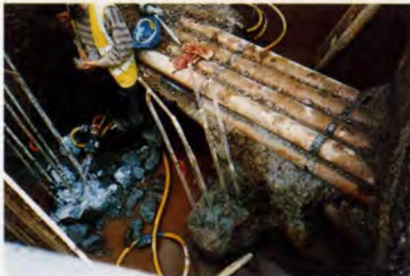
8. Proximity of piles to existing services.
