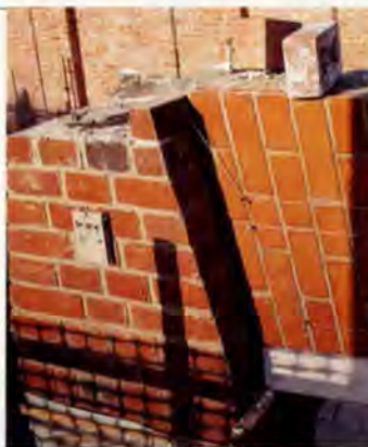
◀ 4. Brickwork detail on arch.
