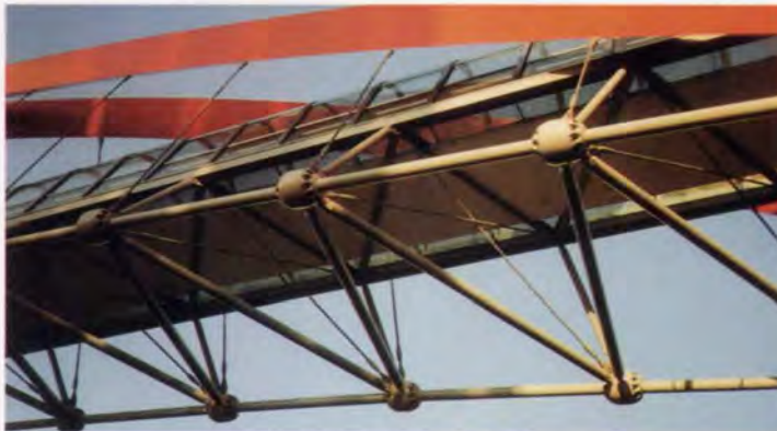
▲ 5. Underside of bridge, showing nodes and struts. ▼ 6. Welding attachments to node.
