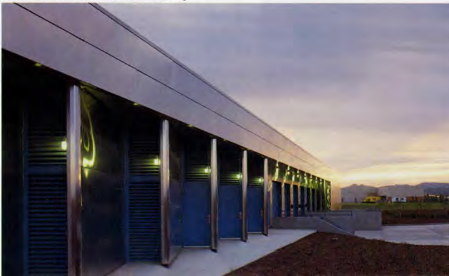
14. Serrated service bar at rear of building.
