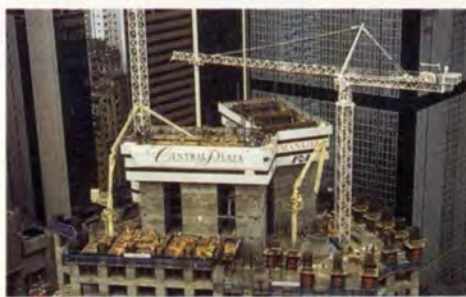
13. above: Steel table forms for floor system construction.
