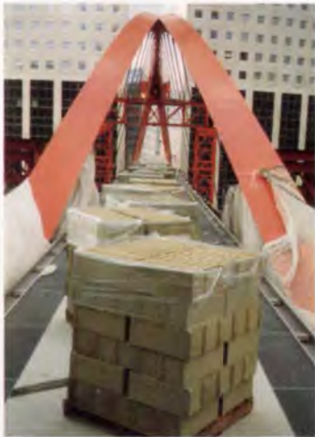
4. French regulations require a full-scale load test for any public bridge.
