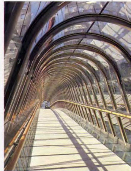
7. Inside the completed bridge.
