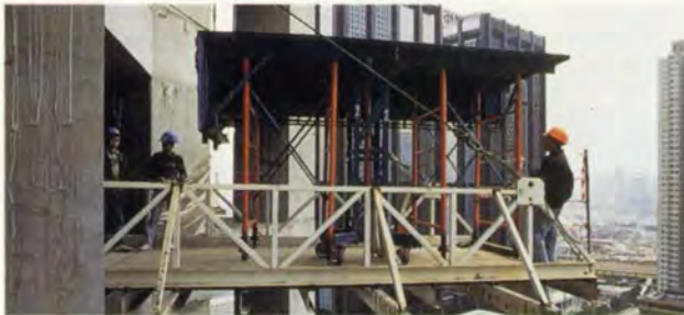
13. above: Steel table forms for floor system construction.
