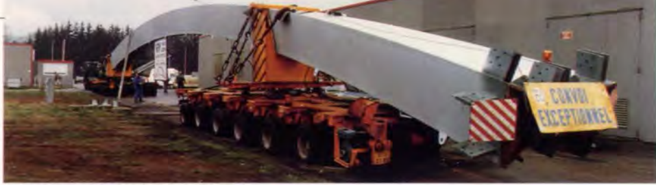
3. Transporting the central section of the arches.
