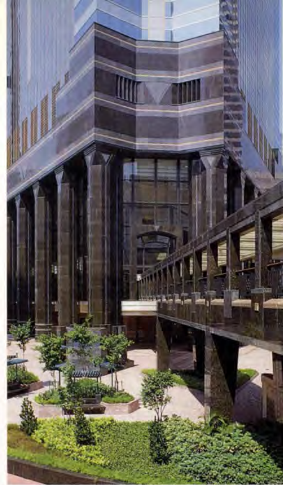
3. First floor pedestrian bridge.
