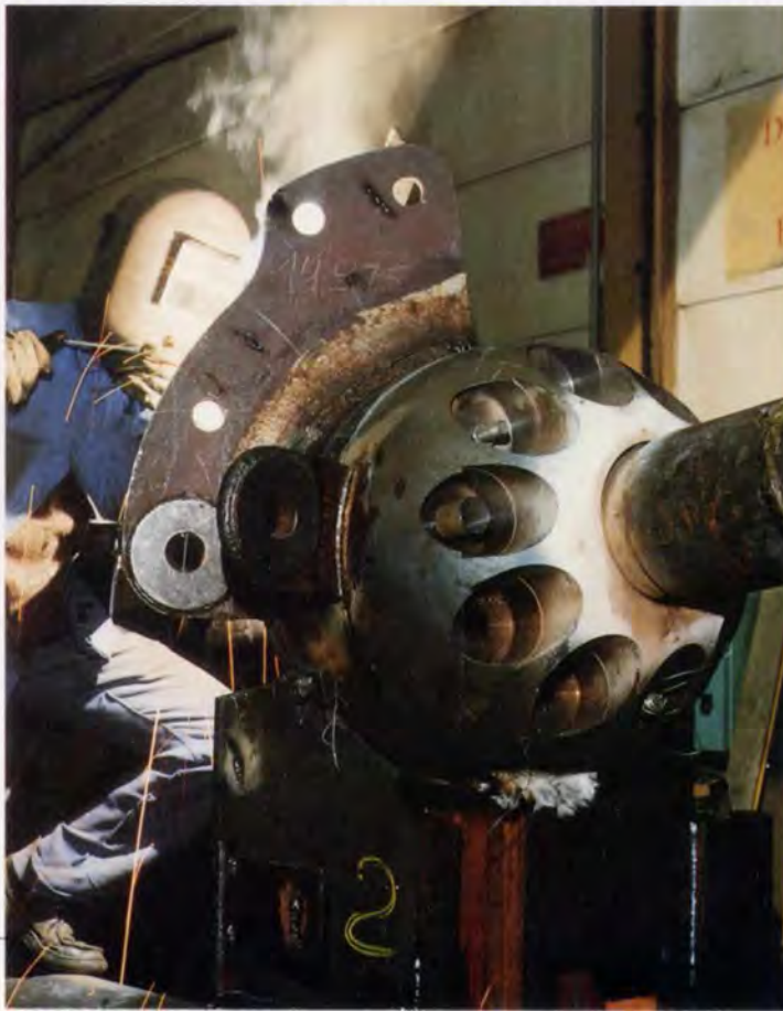
▲ 5. Underside of bridge, showing nodes and struts. ▼ 6. Welding attachments to node.
