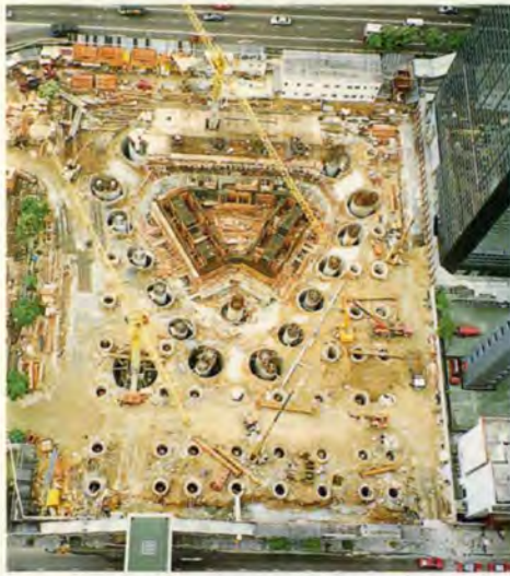
9. Foundations from the air, showing the very large diameter main caissons.
