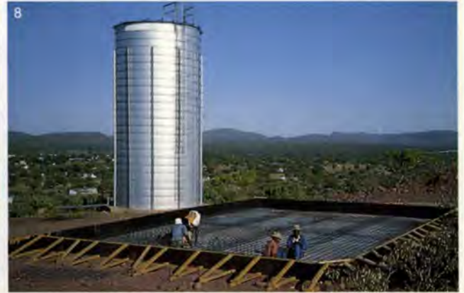
8. Construction of foundation slab for 500m 3 ground tank, with existing 150m 3 tank in background.
