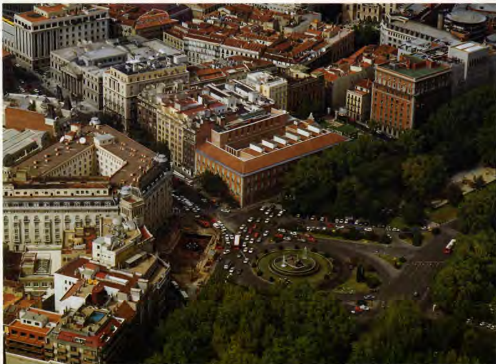
3. Aerial view facing north-west: Plaza de Cánovas de Castillo in foreground.
