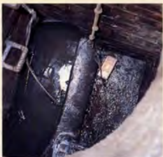
5. Installation of flow monitors.
