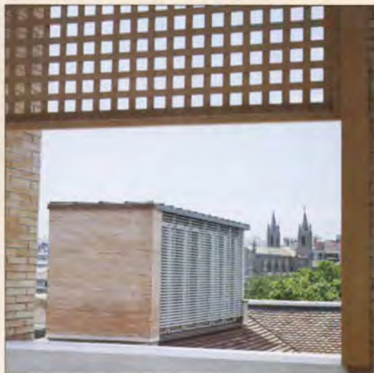
C. Main pump room.
