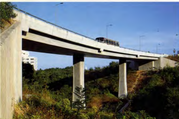
◀ 10. Northern access road bridge.
