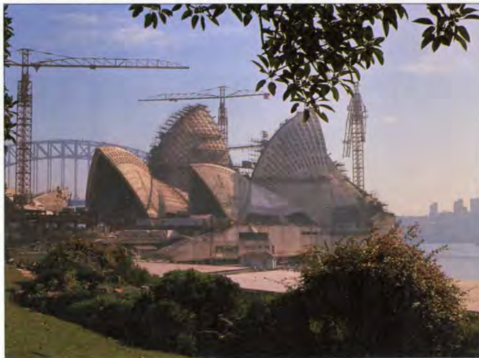
2. The Opera House under construction, photographed by Ove Arup.
