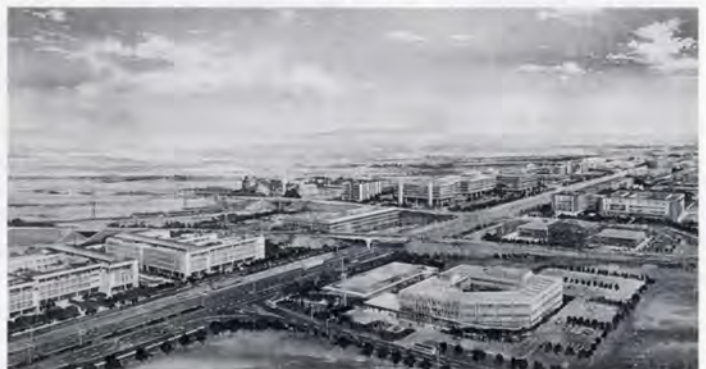
Torgauer Strasse, Leipzig, a 4.5km urban highway and bridge project.
