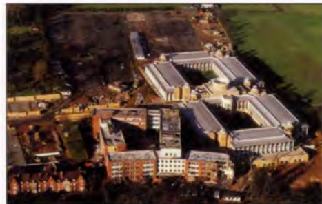
3. Commencing demolition of the old building.
