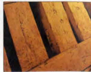
4. Some frame members were soaked in brine as an aid to preservation and marked 'SALT'.
