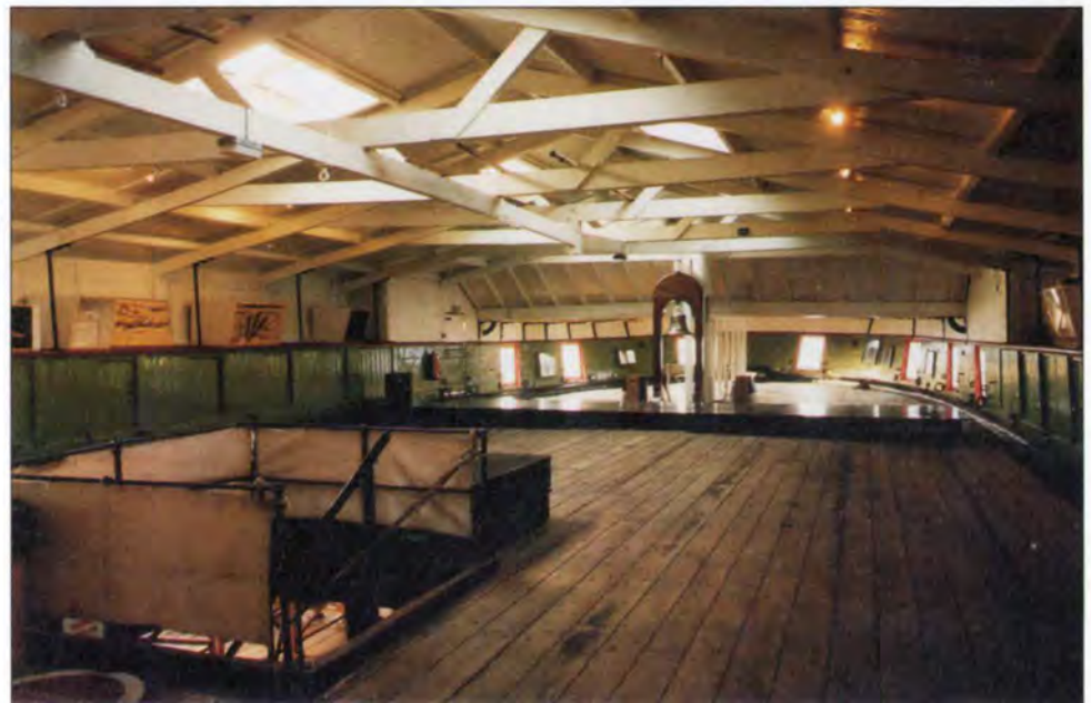
7. The quarter-deck with temporary roof.
