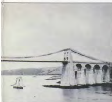
Menai Straits Bridge, 19th century before construction of the main span.
