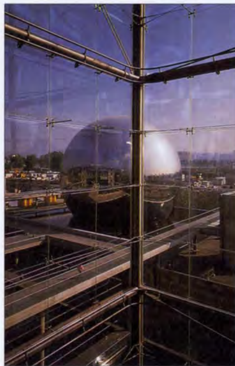
4. Glass façade at The City of Science and Industry, La Villette, Paris: One of Peter Rice's projects from the early '80s. (Photo: Martin Charles)
