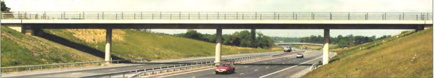
10. Four-span side road bridge.
