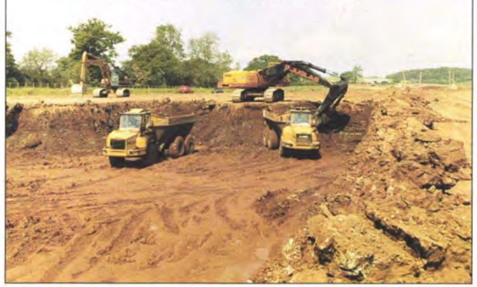
4. Earthworks in progress on Warwick South contract.
