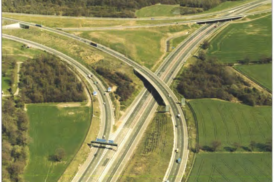
12. Junction between M42 & M40 at Umberslade Park: Warwick North contract.
