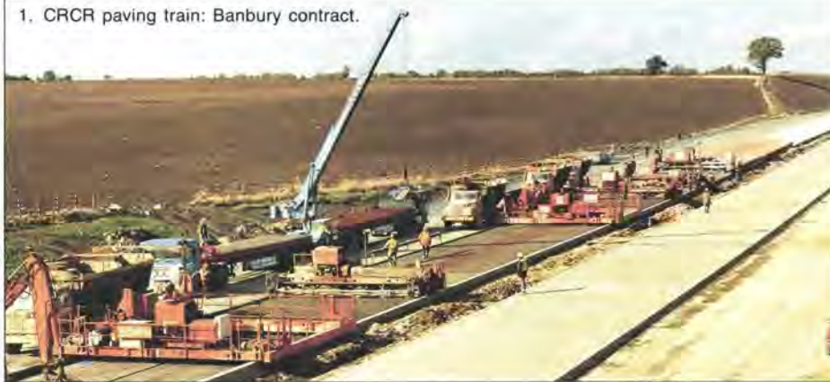
1. CRRC paving train: Banbury contract.
