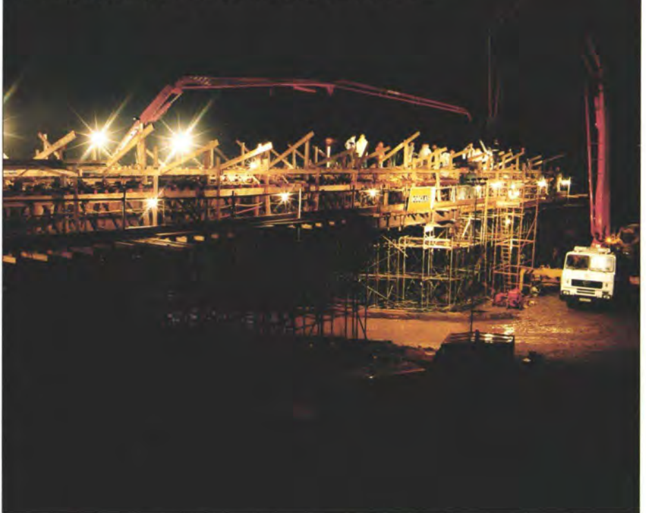
5. Concreting Henley Road Bridge deck: Warwick South contract.
