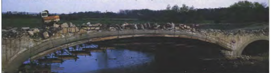
11. Demolition and reconstruction of the existing bridge over the River Avon.
