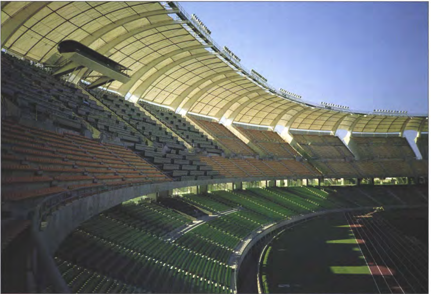
1. Western side, showing press accommodation on upper tier with TV gantry above: note translucency of membrane roof
