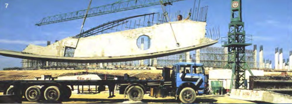
7. Precast radial segment unit to upper stand being hoisted during construction
