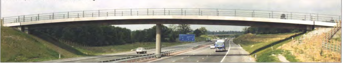
9. Two-span farm accommodation bridge.
