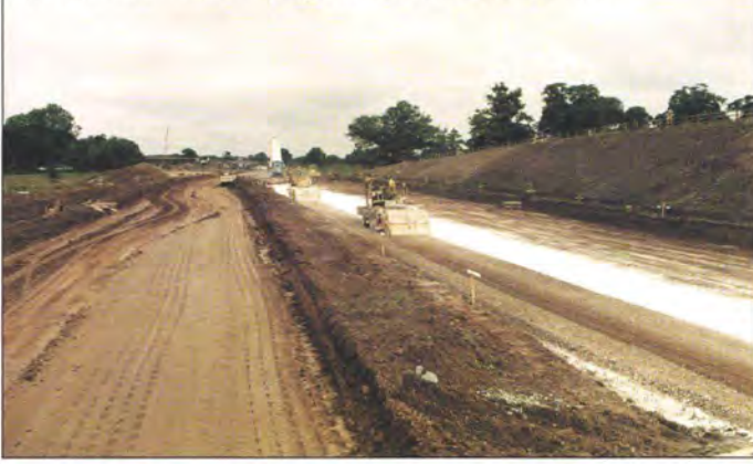
3. Lime stabilization in progress: Warwick North contract.
