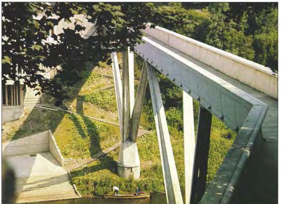
5. Kingsgate footbridge. (Photo: Ove Arup & Partners)
