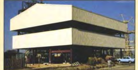
10. Afcott cotton farm: construction of oil refinery.
