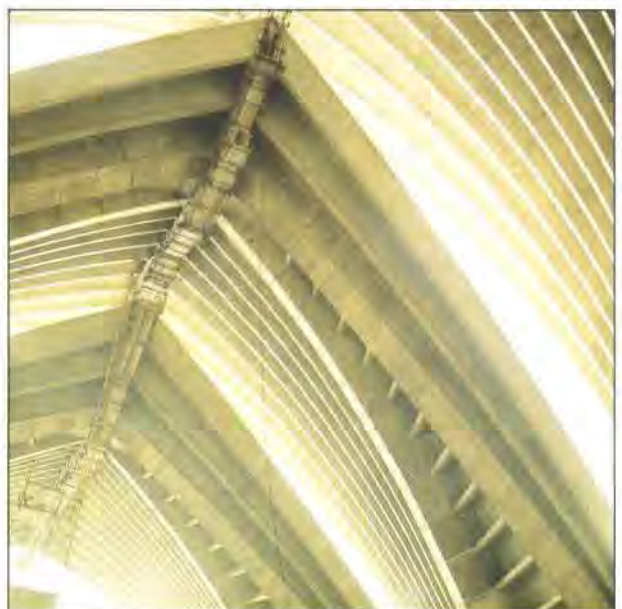
6. Sydney Opera House: model of segmented sphere solution to the design of the shells.
