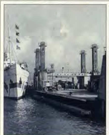
3. Mulberry Harbour pontoon: The crank-shaped fender can be seen just clear of the water. (Photo: Courtesy Imperial War Museum)
