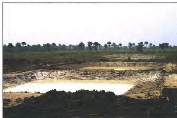
22. Construction of ponds.
