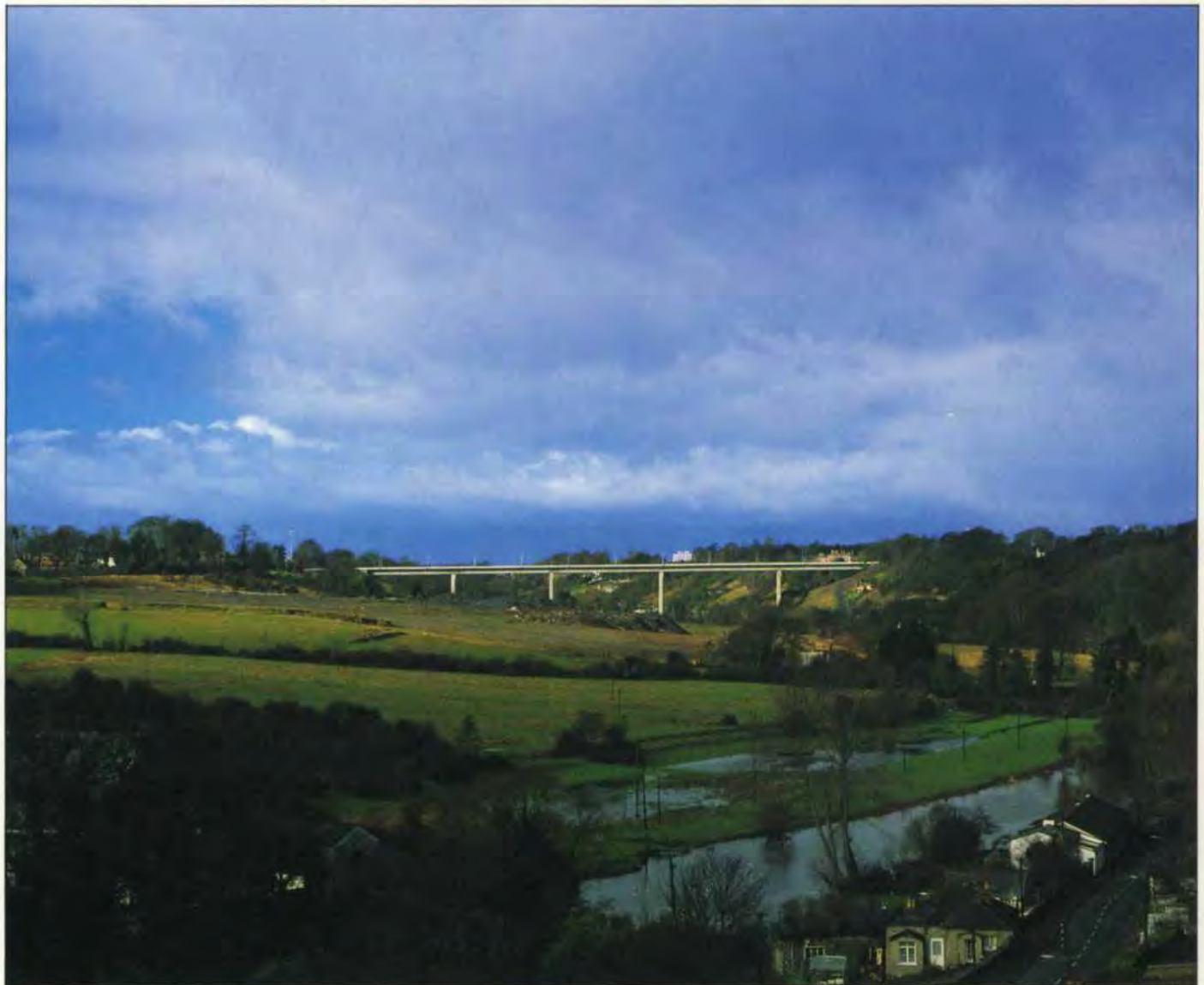
15, 16. The completed Liffey Valley Bridge.
