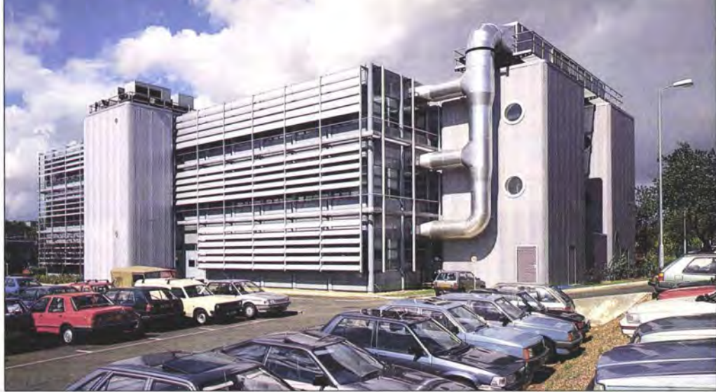
8. General view from north east.
