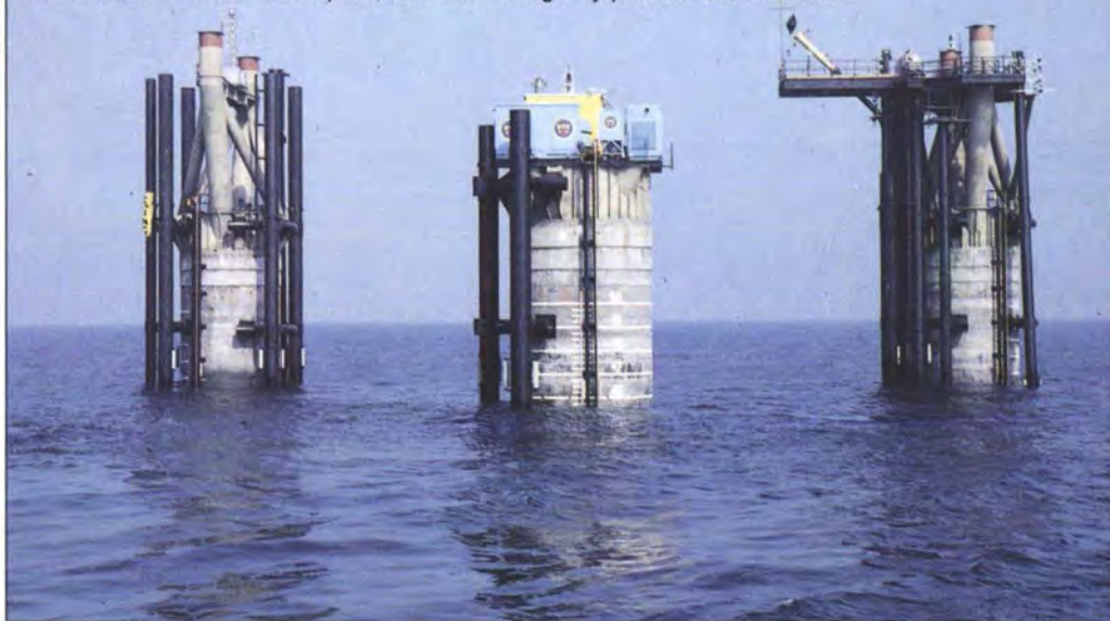
25. Offshore installation complete, with skirt having fully penetrated the seabed.
