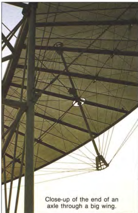
The big wings seen from underneath (the heavy radial lines are welded overlap seams in the membrane).
