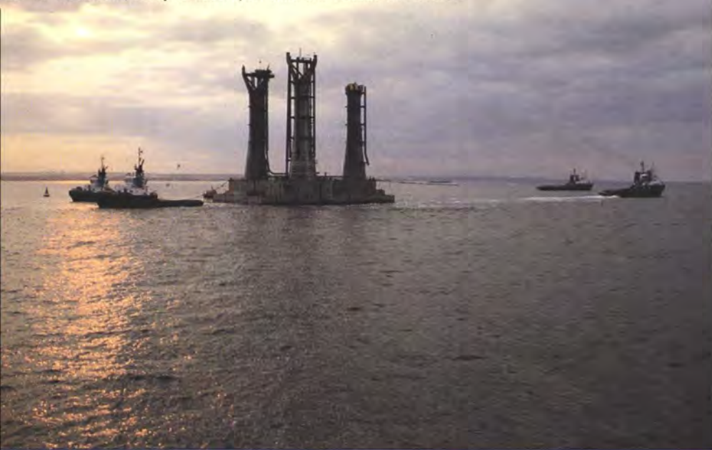
21. Offshore installation: start of flooding closed cells.
