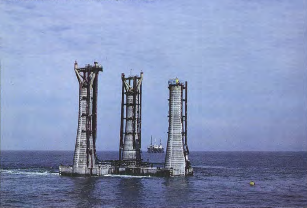
21. Offshore installation: start of flooding closed cells.
