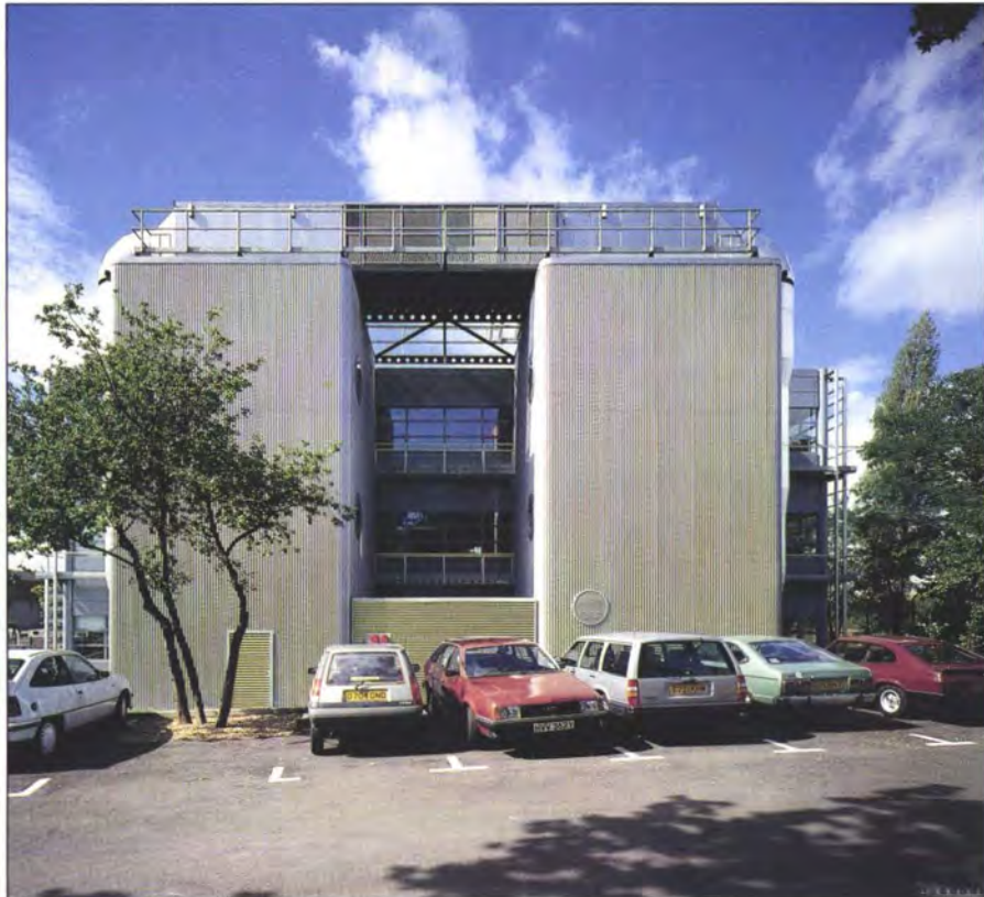
16. North side of the building showing pods, air-handling plant, ducts, and ground floor plantroom.
