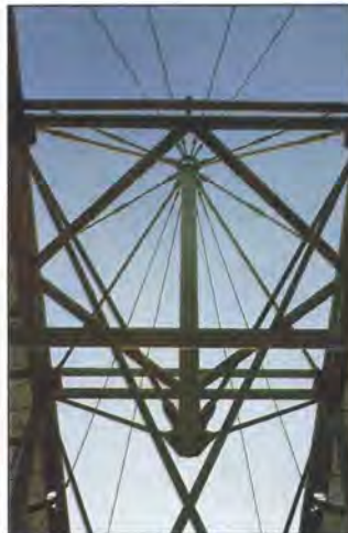
Above: Flying strut at the top of the pylon.
