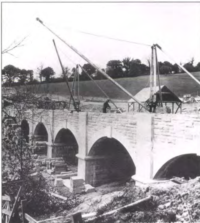
7. Hope Bagot Dingle: Construction of a masonry arch structure
