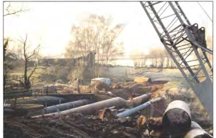
10. Rea River Crossing: The three old pipes are under the canopy on the left of the picture, with work proceeding on installation of the new 60in. main, December 1987.
