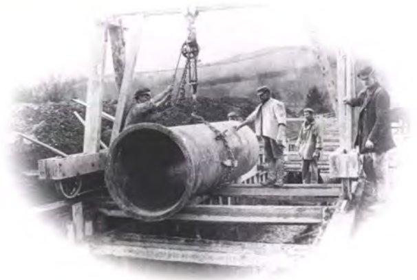
6. Siphon pipe: Installation on Wye siphon, 1897
