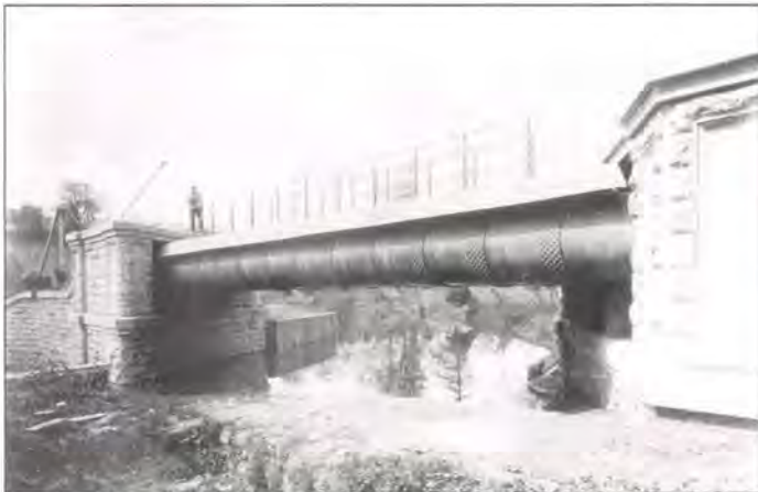
9. Rea River Crossing: Towards the completion of construction in 1902. Three 42in. pipes were installed at this stage.
