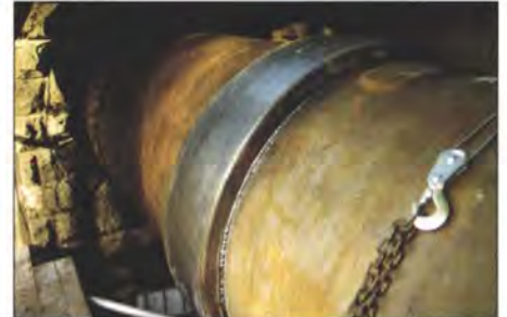
17. Hopton Brook repairs: Strengthening arrangement installed by Severn-Trent, winter 1988-89.
