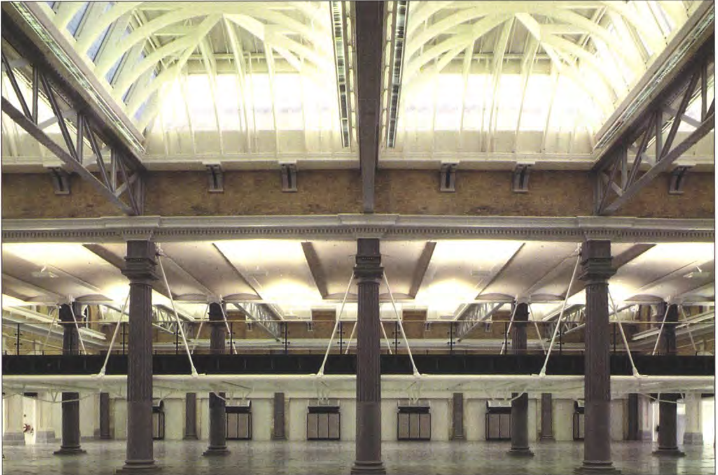
8. Interior showing new demountable mezzanine floor
