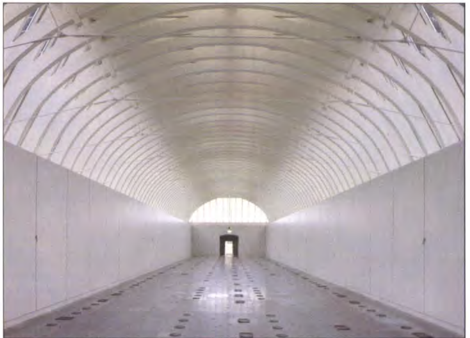
17. Interior of Haddock Gallery showing the effect of prismatic lighting system
