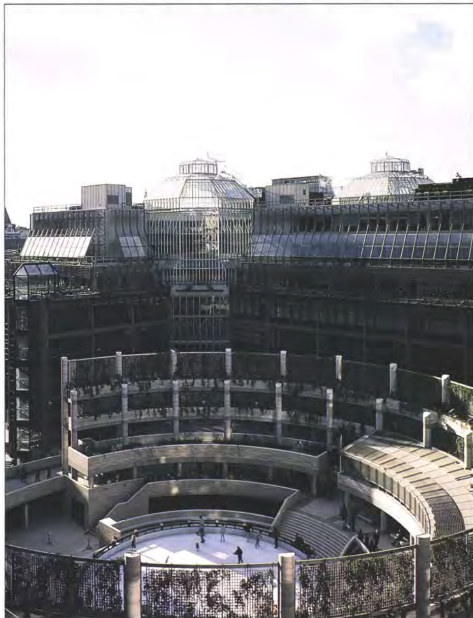
2. Looking south-west across Broadgate Square from Phase 4 level 8. (Photo: Jeremy Cockayne)
