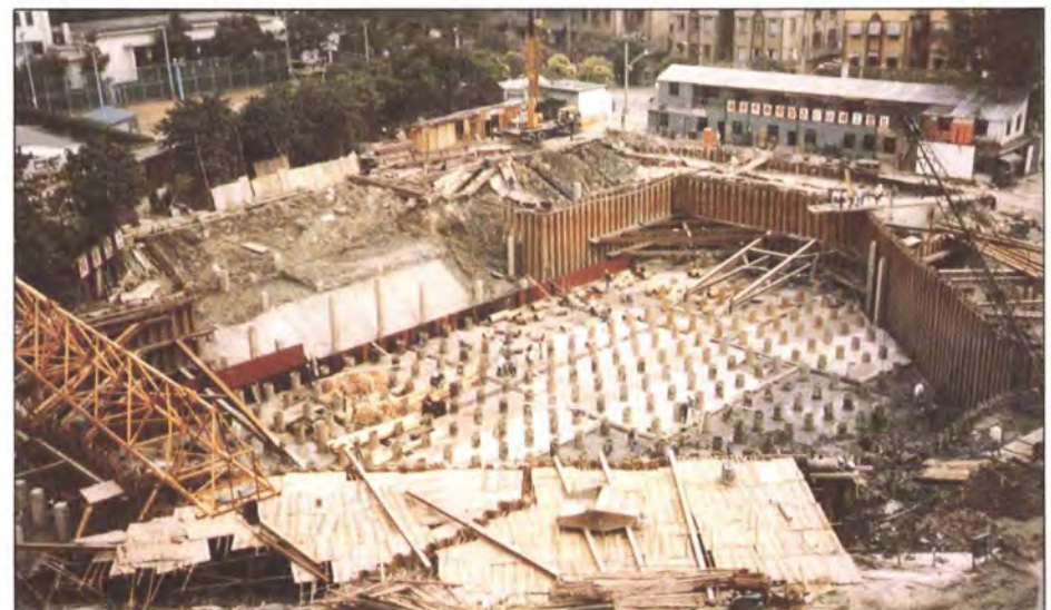
Jin Cang Mandarin Hotel: driven steel piles
