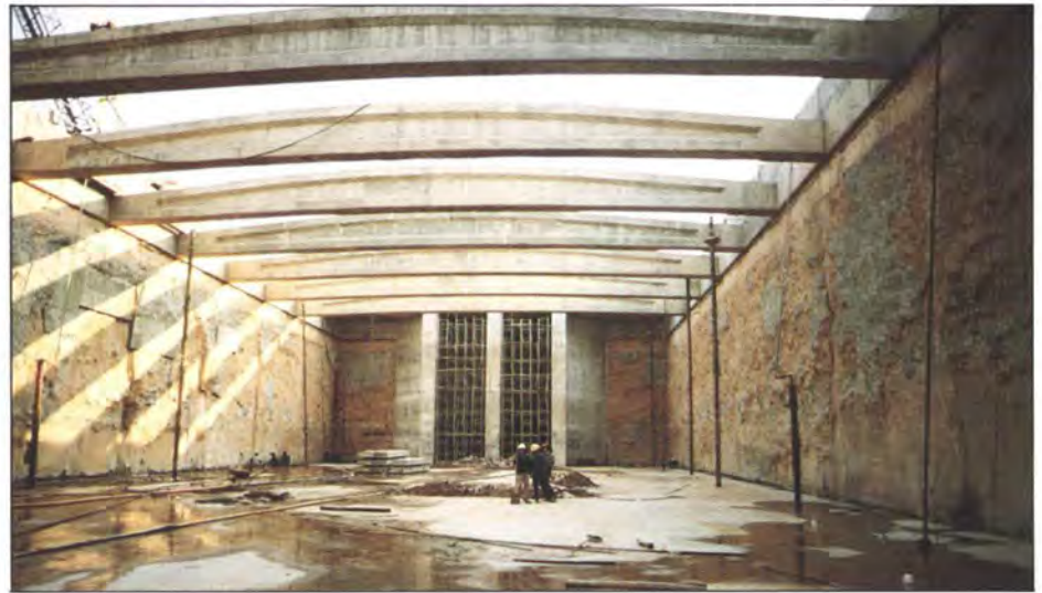
7. Shajiao Power Station: 1.2m thick diaphragm wall for stilling basin
