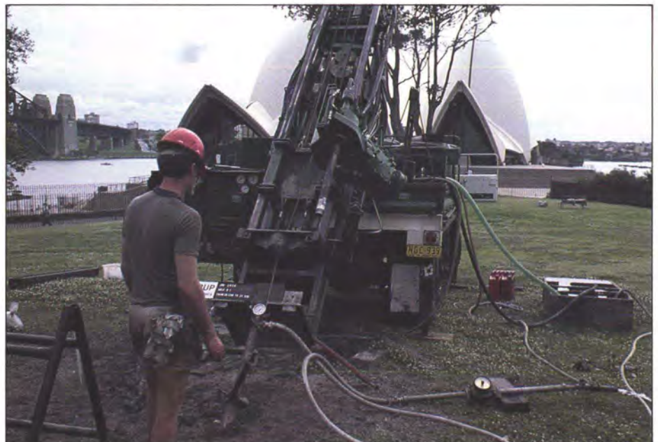
Proposed Bennelong Point underground car park: In situ permeability testing
