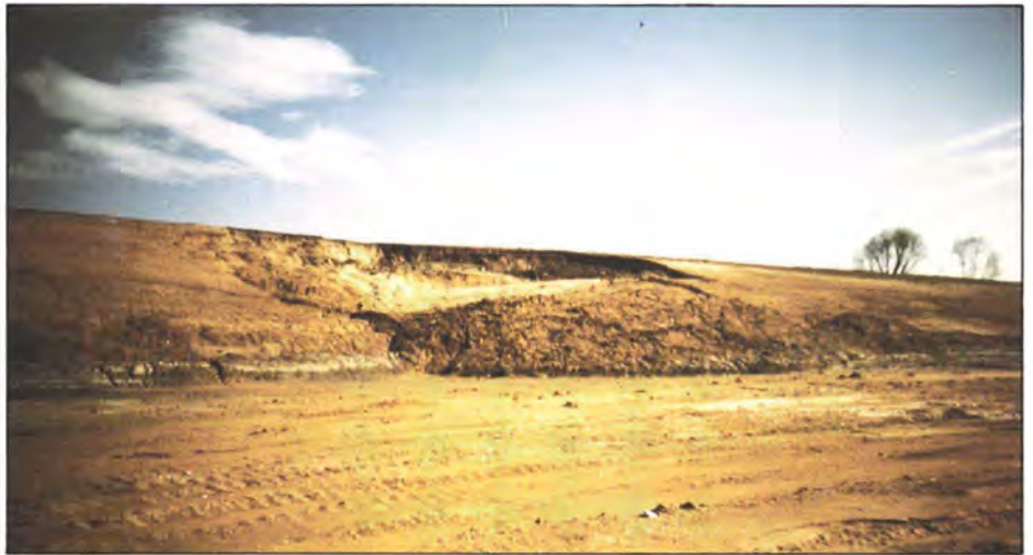
Above and below: Slope failure.
