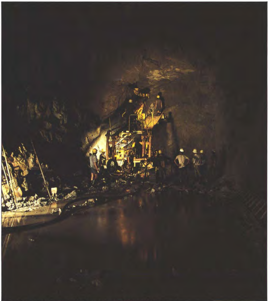
Sea water tunnel construction, Hongkong Bank (Photo: N. Farrin)
