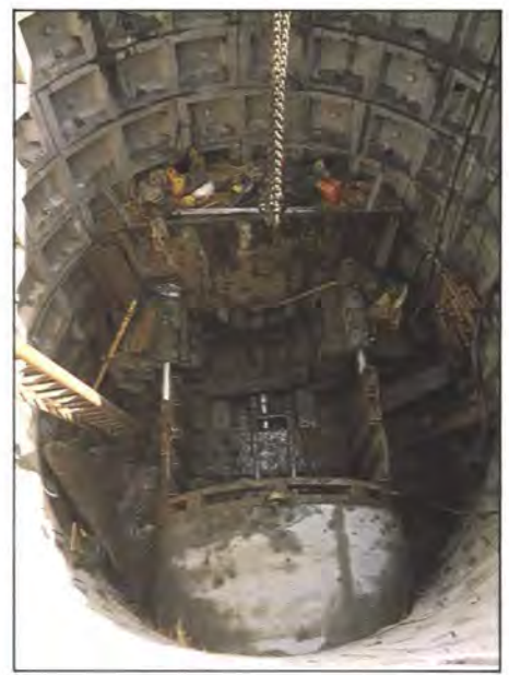
Access shaft, sewer installation, Dundee
