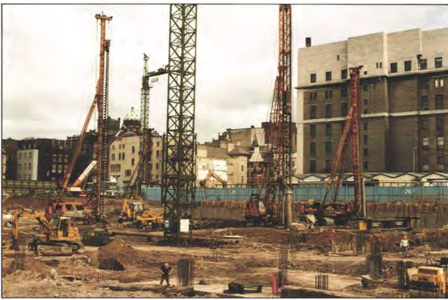
Continuous flight auger piling, St Enoch Square, Glasgow
