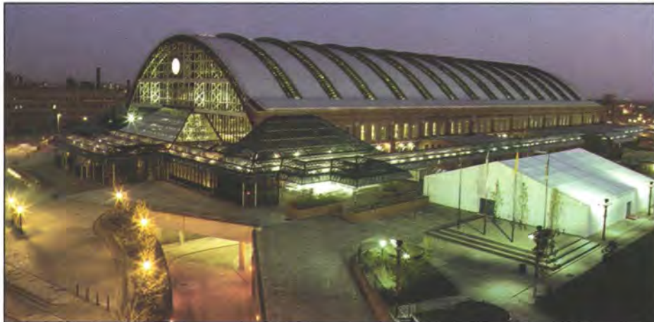
1. Central Station was closed by British Rail in 1969 (Photo: Barry Tyler)
