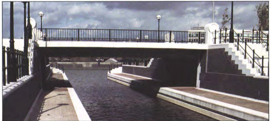
12. Completed canal and bridge (Photo: John Morgan)
