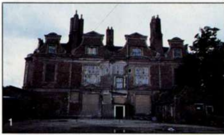
1. Courtyard elevation before commencement of works 2. Courtyard elevation after refurbishment 3. West elevation after refurbishment
