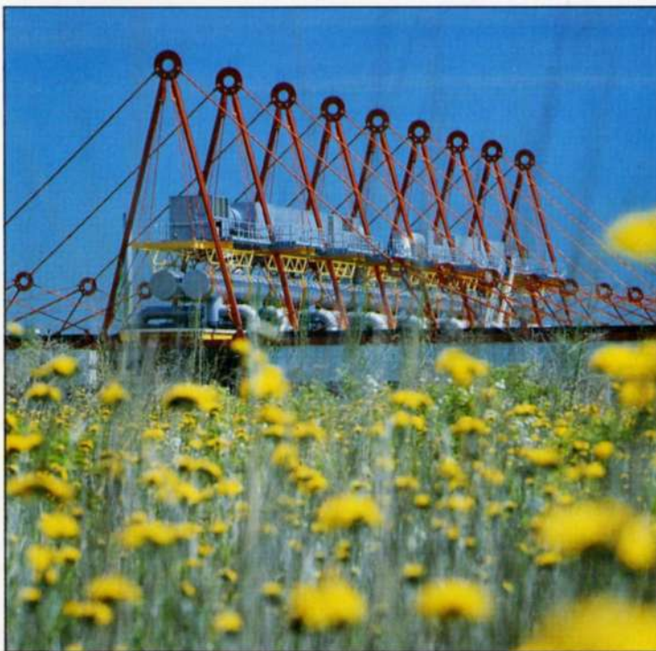
18. Air handling plant on yellow support platforms with primary ducts below (Photo: Otto Baitz)
