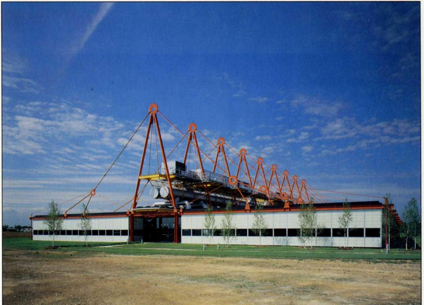
22. General view from landscaped parkland shortly after completion (Photo: Otto Baitz)
