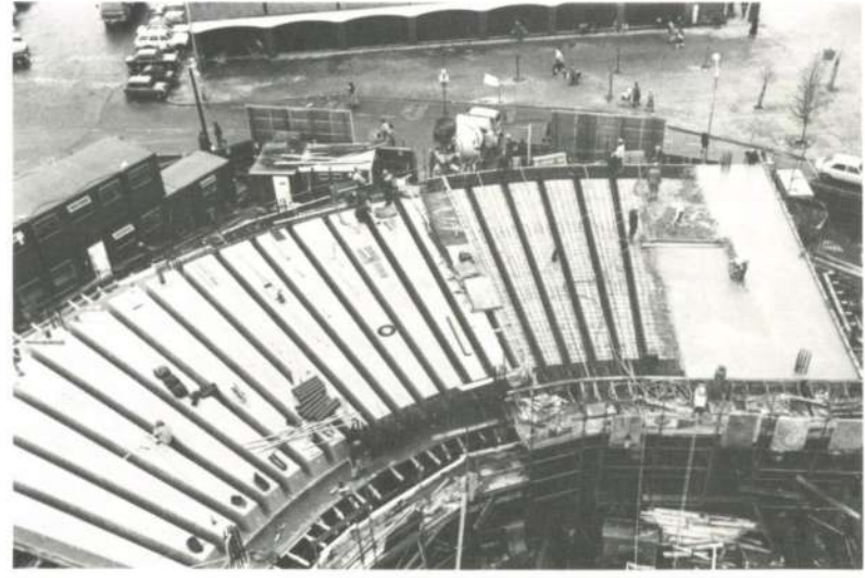
Fig. 9 Radial floor beams under construction
