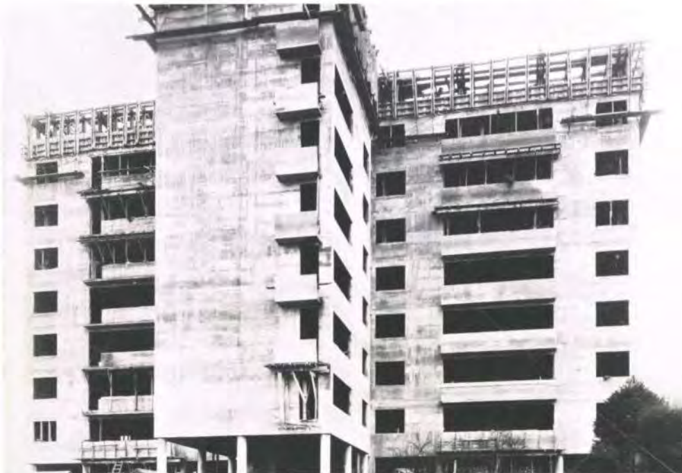
4 Construction and right: interior of Highpoint 1
