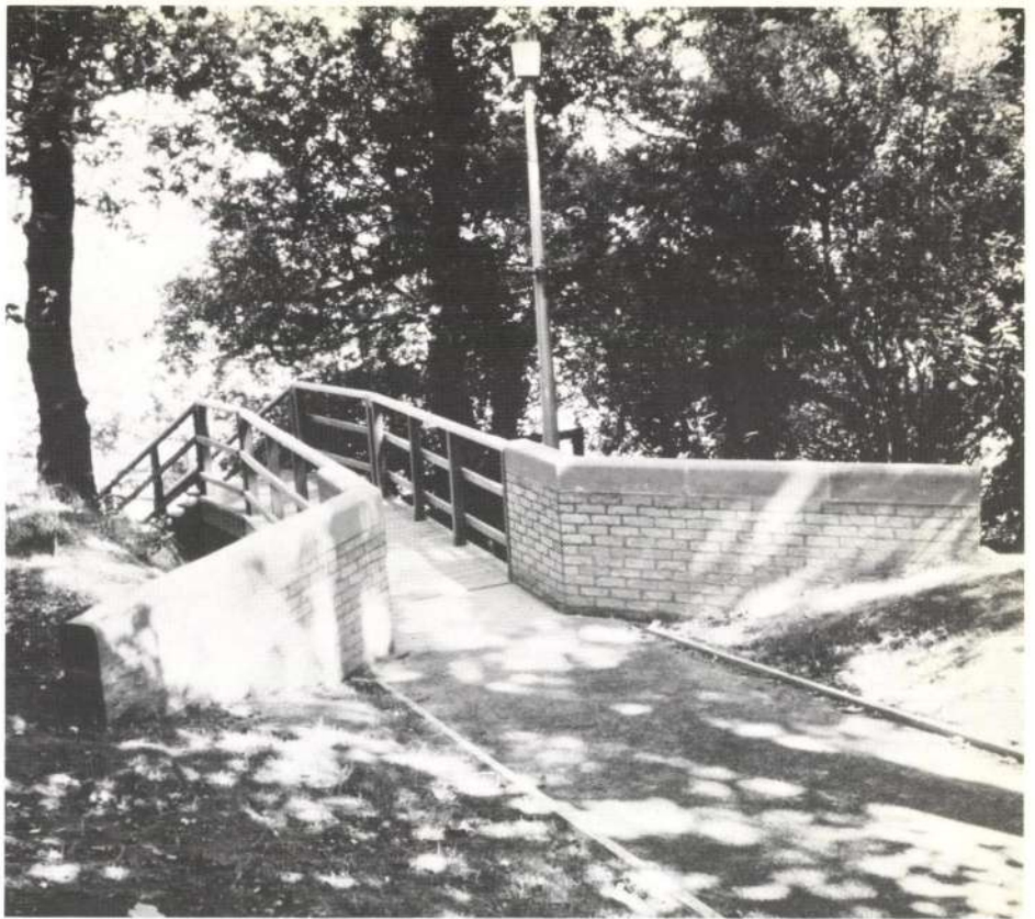
Fig. 1 The approach to Wylam footbridge showing the abutments in hand-made brick
