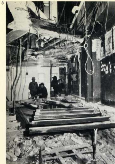
Fig. 3 Existing structural timbers forming galleries
