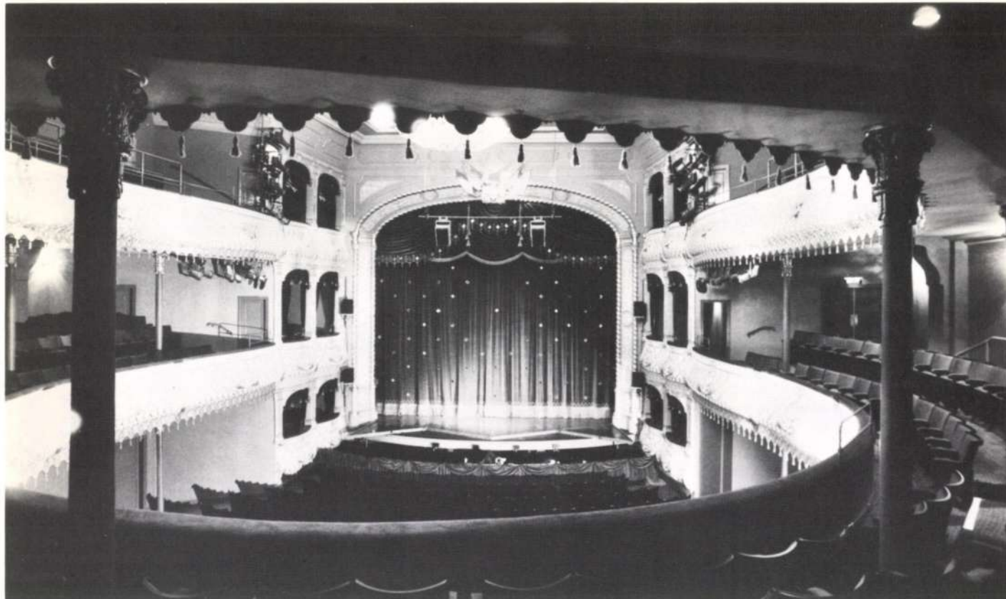
Fig. 15 Auditorium with reinstated boxes and circle seating. (Photo: Ove Arup & Partners)
