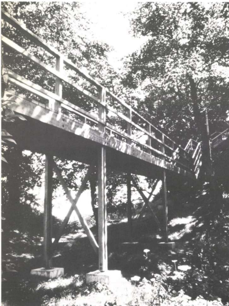
Fig. 5 Wylam footbridge: View from the woodland floor
