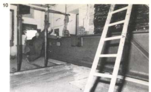
Fig. 8 Steel needles to support flytower wall before permanent structure installed
