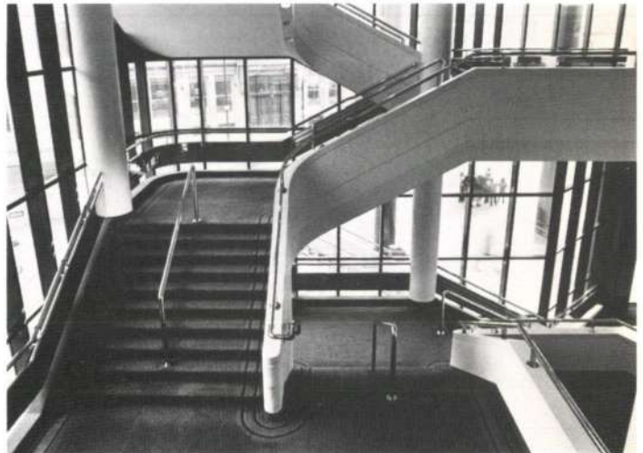
Fig. 6 Internal view of foyer stairway showing perimeter convactor heating.
