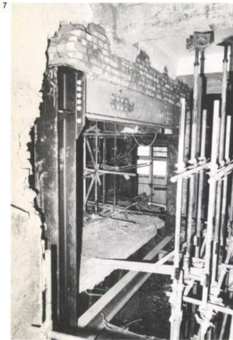
Fig. 10 Manhandling upper beam into place
