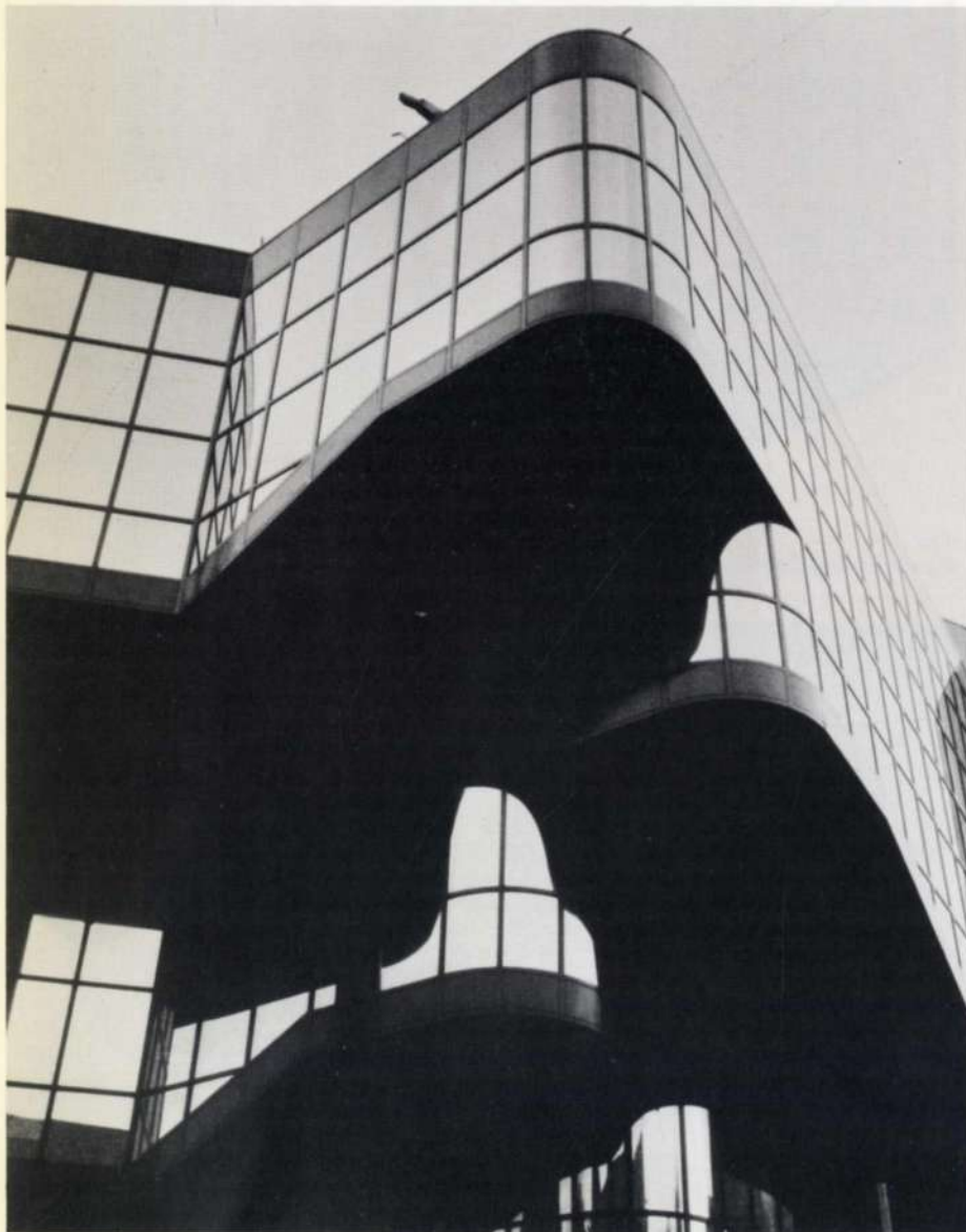
Fig. 7 External view of foyer cranked cantilever staircase and curtain walling.
