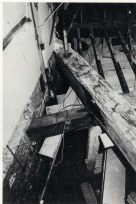
Fig. 5 End conditions at existing timber gallery supports
