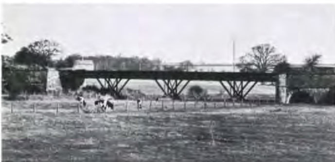
Fig. 5 Longdon-on-Tern aqueduct by Telford 1795 – an intuitive trial of cast iron for a greater project
