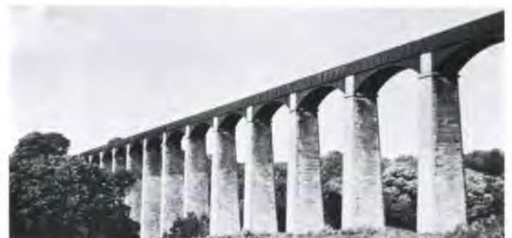
Fig. 6 Pont-Cysyllte aqueduct by Telford 1795-1803 – Hailed by Sir Walter Scott as the greatest work of art he had ever seen (Photo: Architectural Association)
