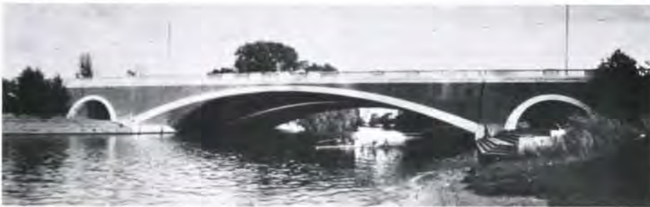
Fig. 3 Runnymede Bridge by Lutyens 1935 – Precedents (Photo: Ove Arup & Partners)
