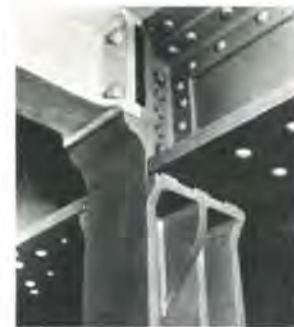
Fig. 8 Sheerness Boat Store by Col. Green 1858-60 – the frame emerges
