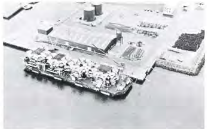
Fig. 7 Foundation template units on barge at Invergordon awaiting final shipment to Hutton TLP site, for installation
