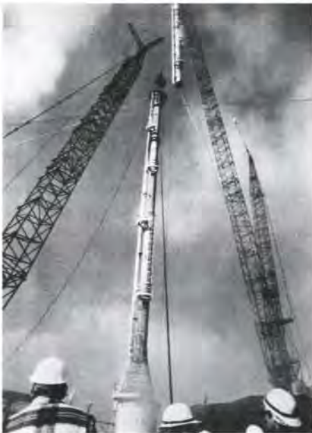
Fort McMurray flare stack, Canada: erection of guyed riser with riser fabricated in sections and erected in two parts. Designed by Ove Arup & Partners. (Photo: courtesy of Bechtel International)
