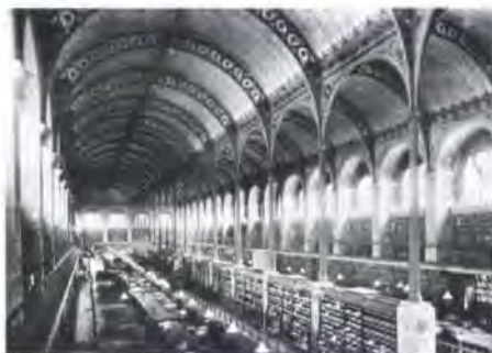
Fig. 11 St. Geneviève Library 1843 – banded barrel vaults in stone replaced by banded barrel vaults in cast iron (Photo: Architectural Association)
