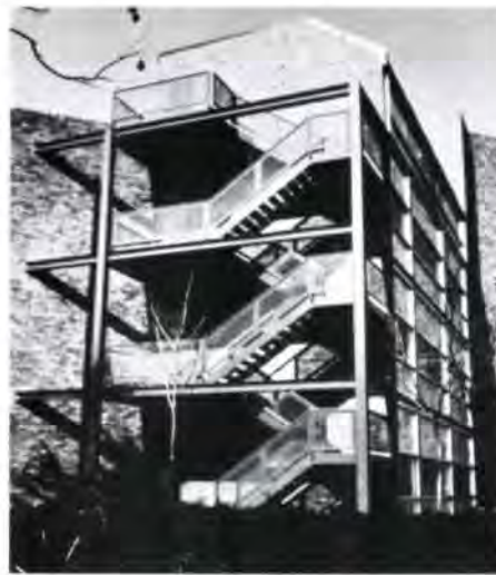
Fig. 7 11 Wellington Road, Parktown. Architects: Design Collaborative
