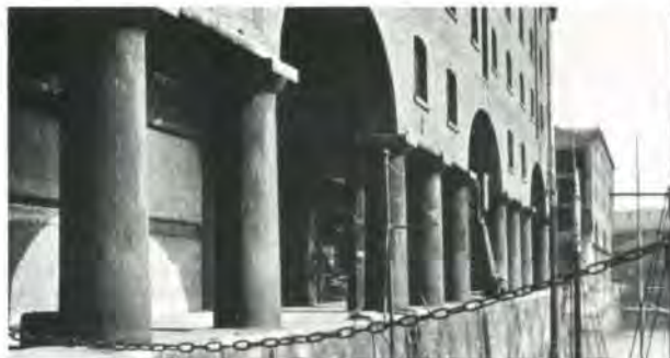
Fig. 7 Albert Dock buildings in Liverpool by Hartley 1848 – the Doric Columns are cast iron
