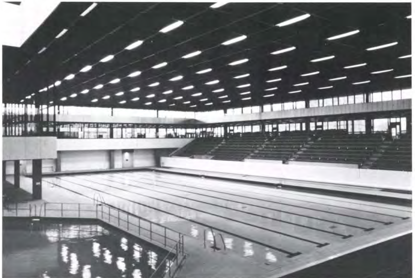
Fig. 2 The Royal Commonwealth Pool. Architects: Robert Matthew, Johnson-Marshall & Partners
