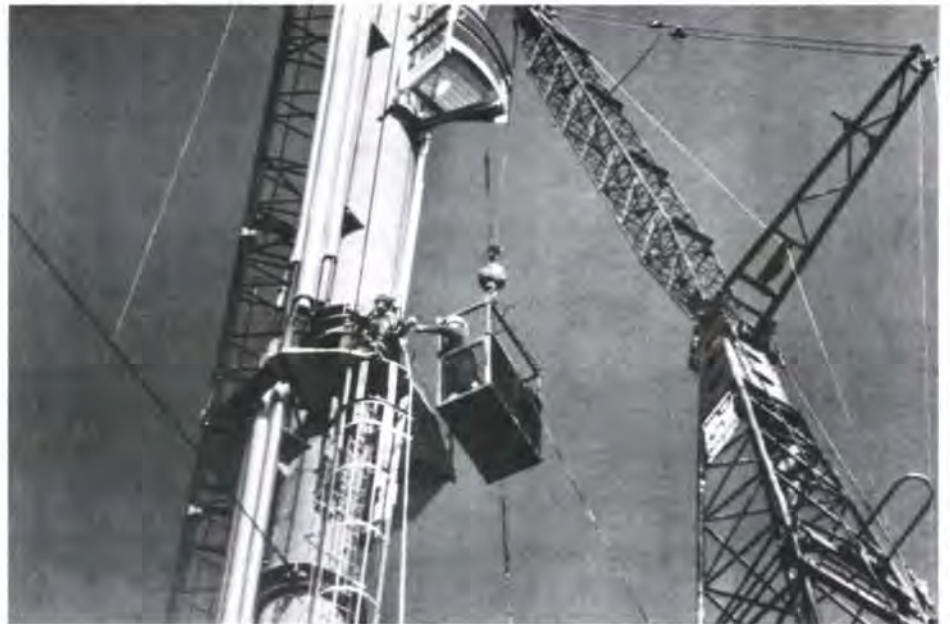
Fort McMurray flare stack, Canada: erection of guyed riser with riser fabricated in sections and erected in two parts. Designed by Ove Arup & Partners. (Photo: courtesy of Bechtel International)
