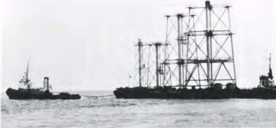
Fig. 4 Brent C flare tower: transportation of prefabricated sections. Arups carried out dynamic fatigue and analysis checks as well as being responsible for obtaining certification. We were also responsible for the appraisal of lifting and temporary works. (Photo: courtesy of Sea and Land Pipelines)
