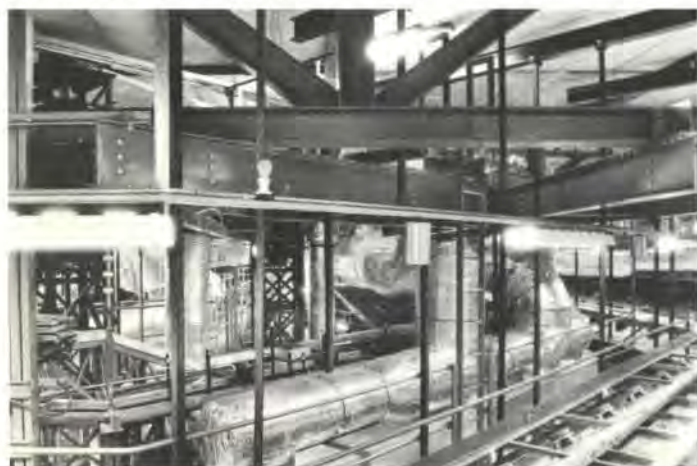
Fig. 9 Ceiling structure and services installations
