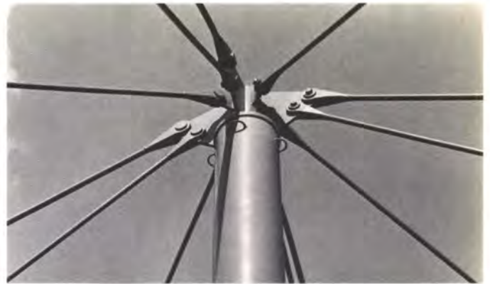
Fig. 13 Boom end detail
