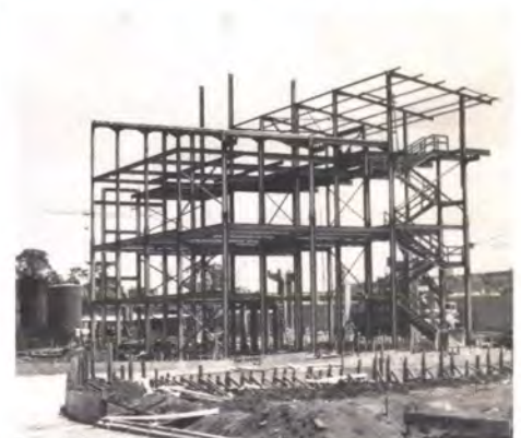
Fig. 15 Erection of refinery steelwork (Photo : Bill Haigh)
