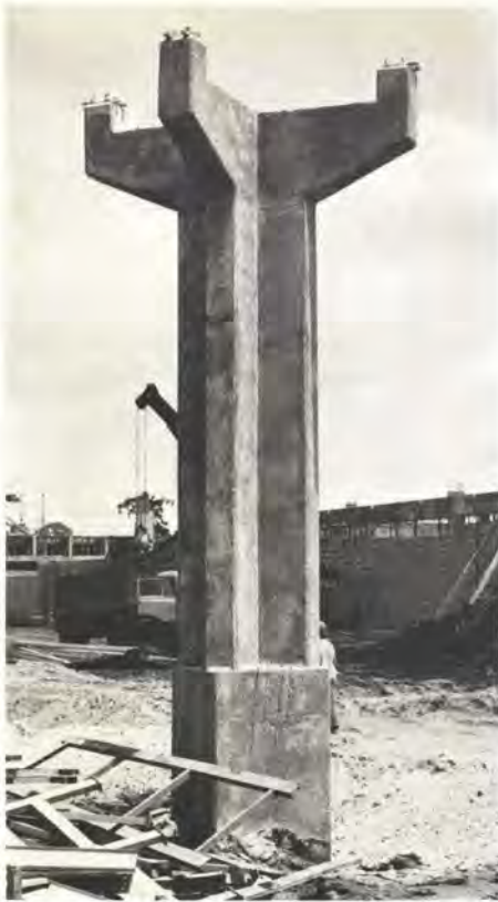
Fig. 16 Cruciform column to carry pipe bridge (Photo: Bill Haigh)
