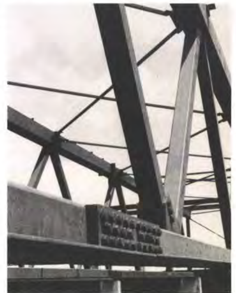
Fig. 21 Joint detail in tubular Warren truss (Photo: Bill Haigh)
