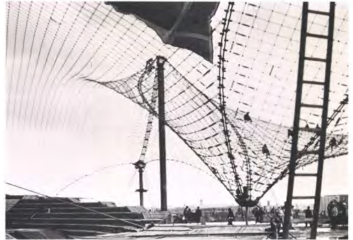
Fig. 4 Cable net at Munich (Photo : Joachim Schock)
