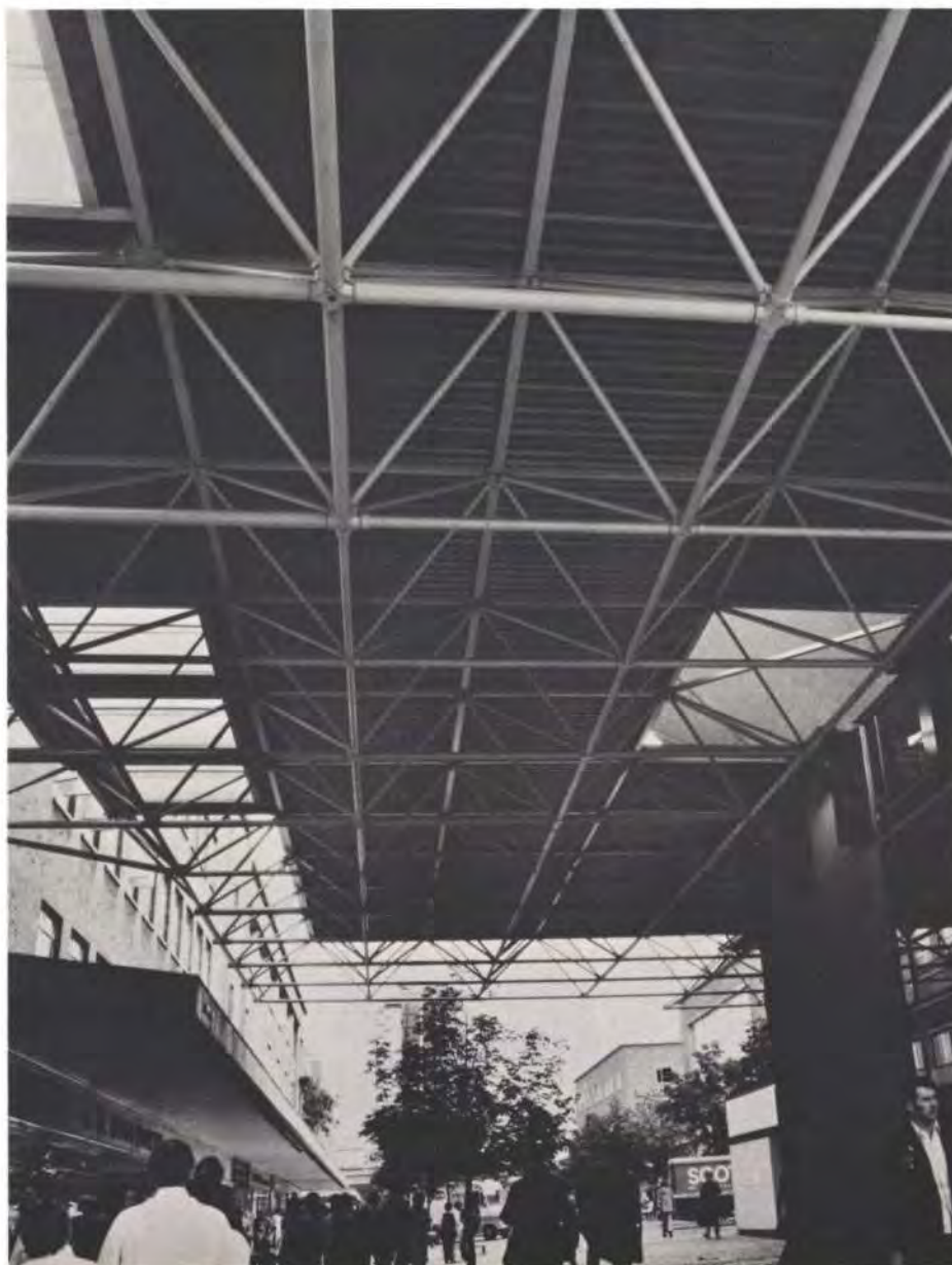
Fig. 19 below The unclad soffit of the wind canopy (Photo: BSC Tubes Ltd.)
