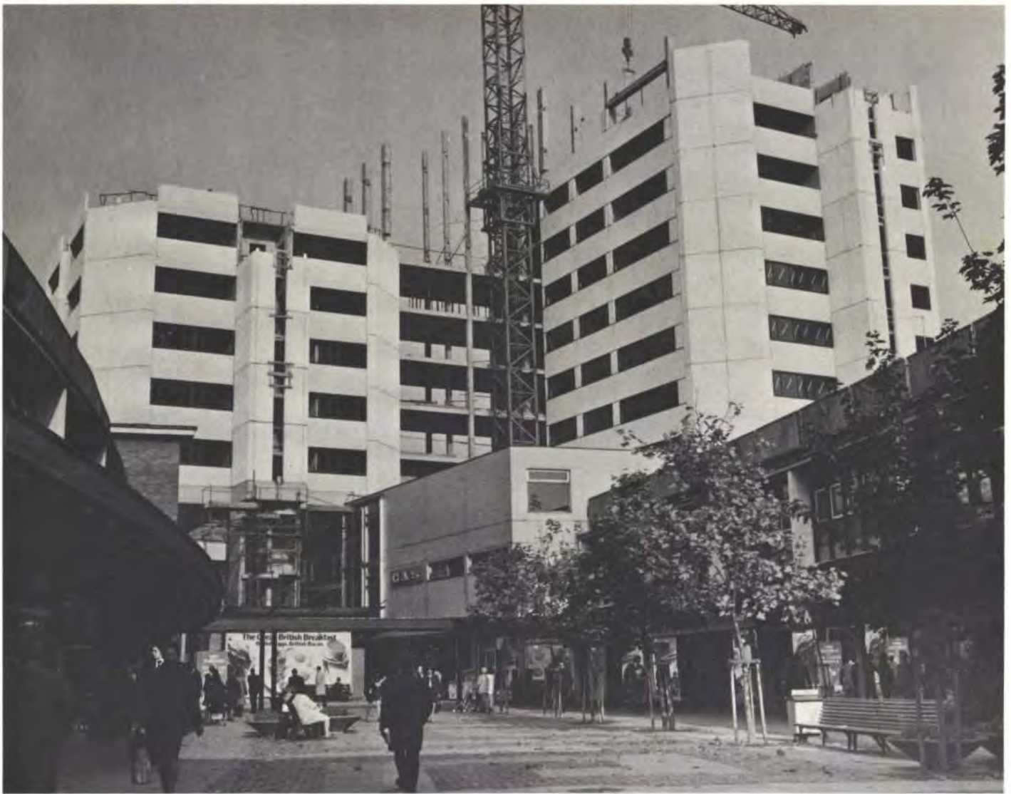
Fig. 14 Erection of precast superstructure (Photo: ICA Studios Ltd.)
