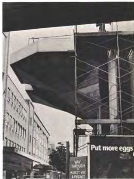
Fig. 7 The completed double cantilever showing access beneath for pedestrians and service vehicles (Photo: The John Madin Design Group)
