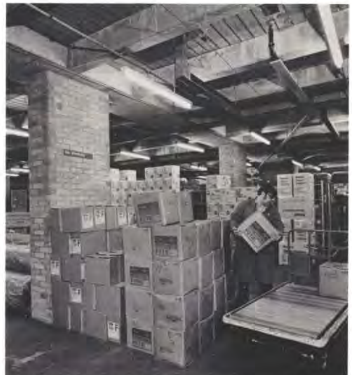
Fig. 18 The central stores, with the basic floor structure exposed (Photo: Allan Glenwright)
