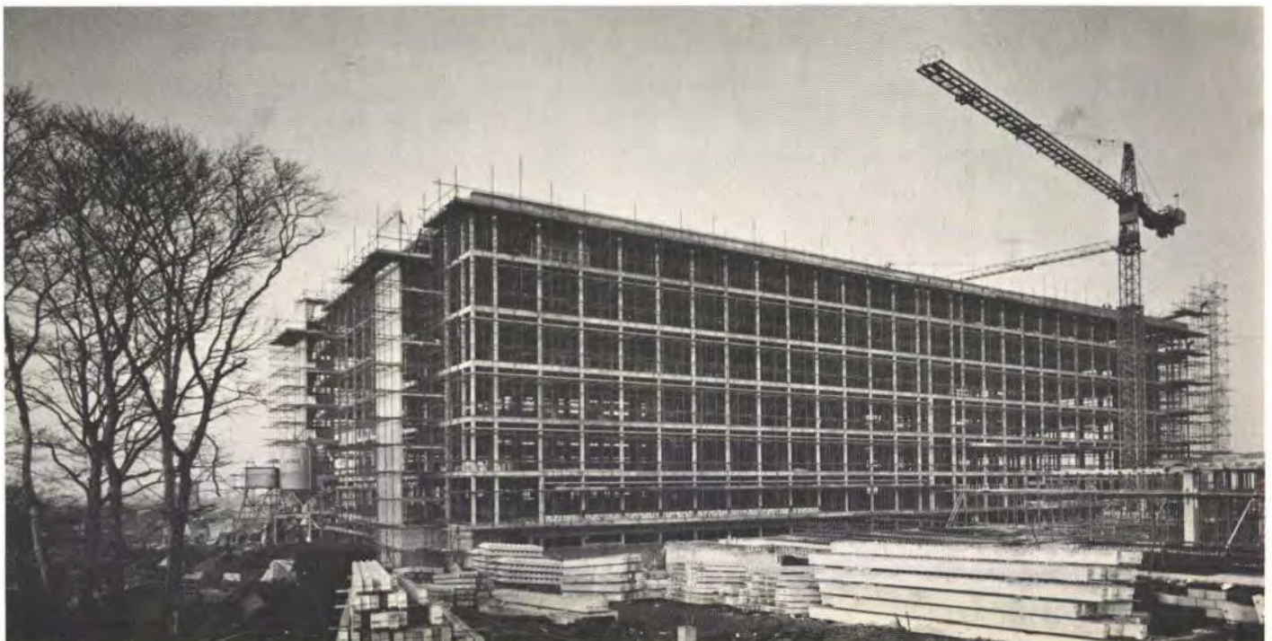
Fig. 6 The Ward Block under construction (Photo: Turners (Photography) Ltd.)
