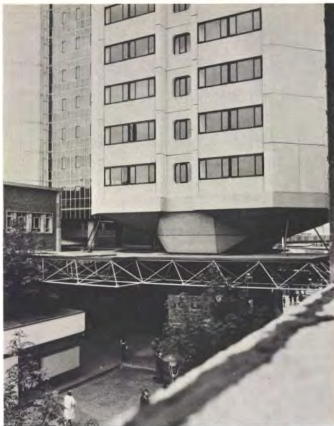
Fig. 16 Wind canopy supported on inclined hangers and fitting closely to the surrounding buildings (Photo: BSC Tubes Ltd.)
