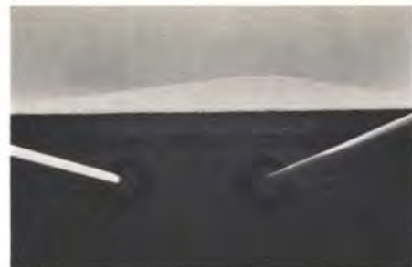
Fig. 17 Tubular hanger casings surround Macalloy rods (Photo: Ove Arup & Partners)
