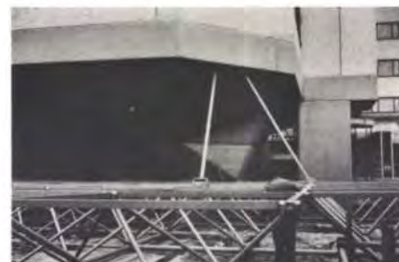
Fig. 18 Inclined hangers support the space frame (Photo: Ove Arup & Partners)
