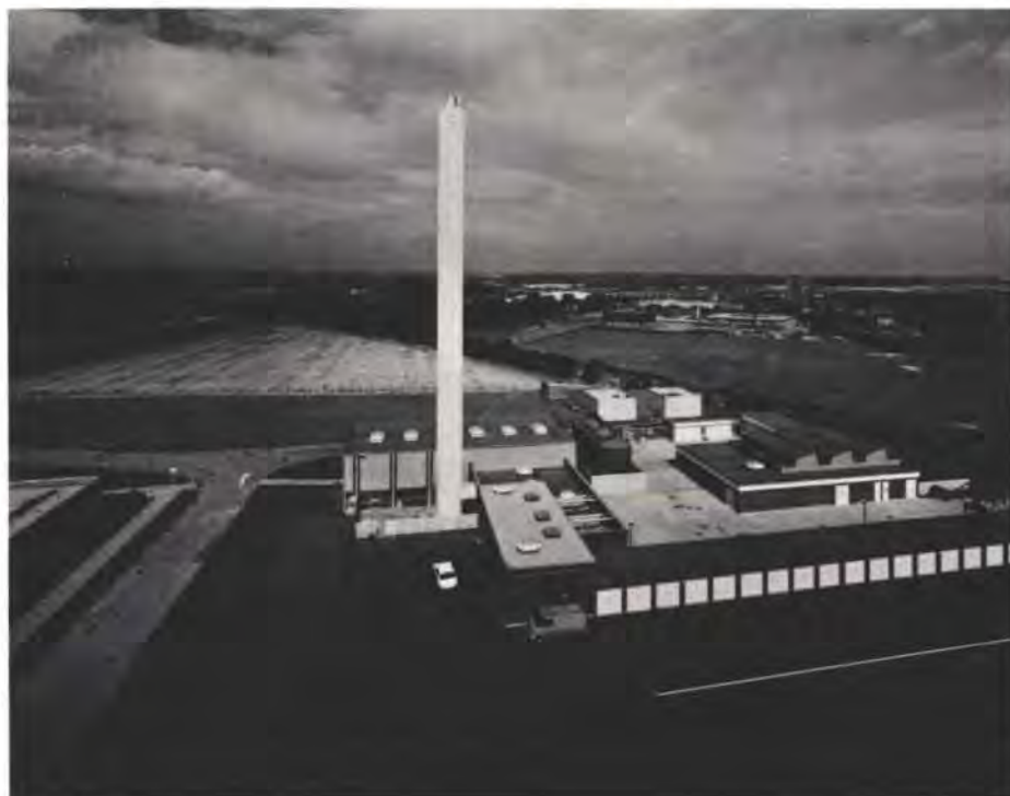
Fig. 13 The works area (Photo: John Laing & Son Ltd.)
