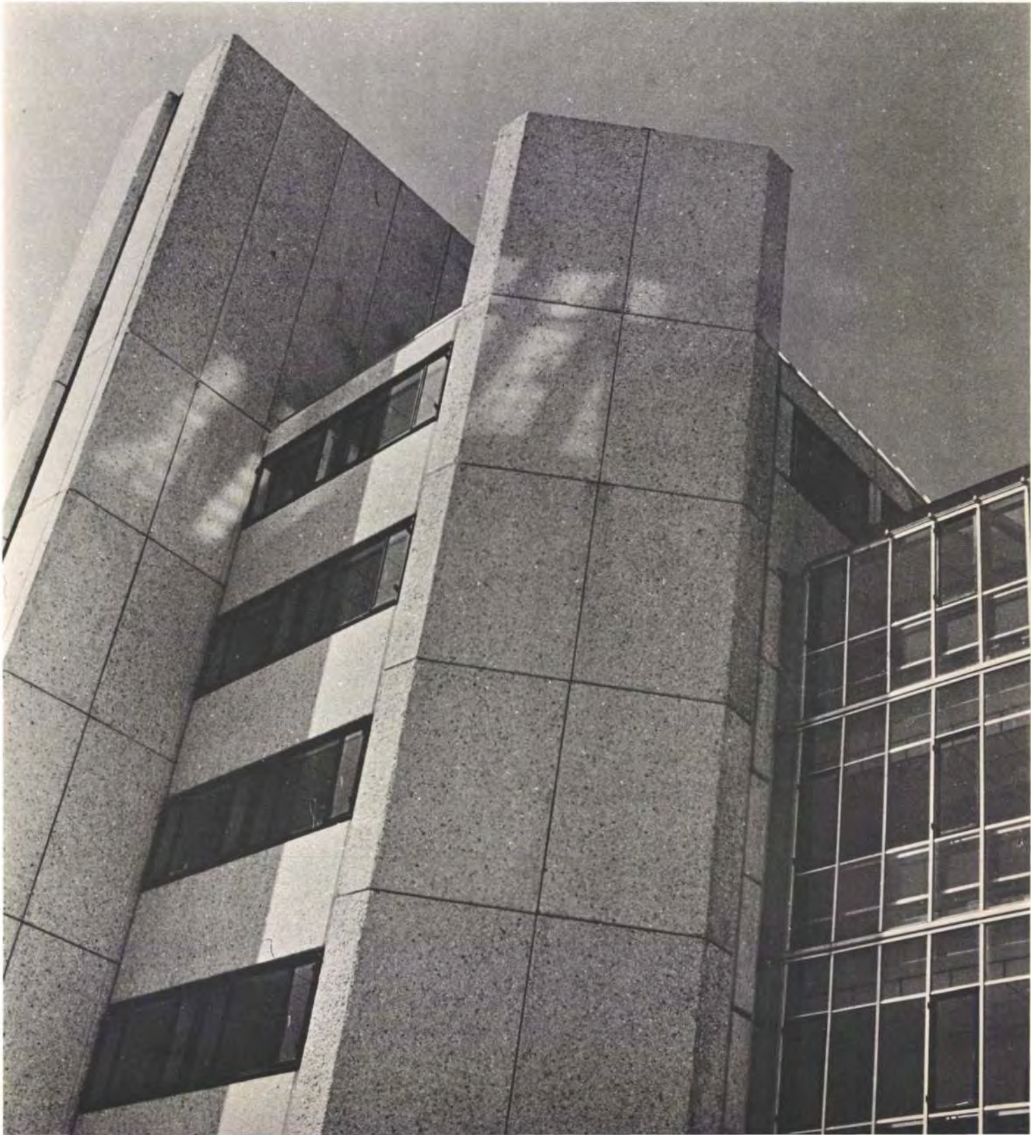
Fig. 21 below White finish on the precast splay-corner walls (Photo: Henk Snoek)
