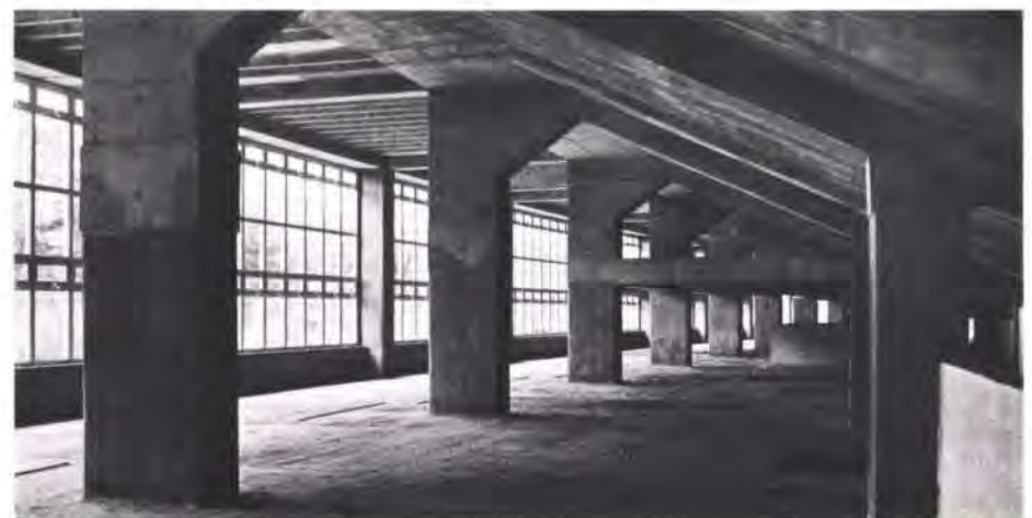
Fig. 16 Internal view of structure at level 2 (Photo: Harry Sowden)
