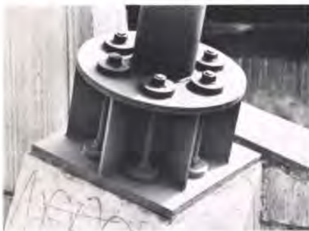
Fig. 4 Backtie-holding down detail (Photo: Harry Sowden)
