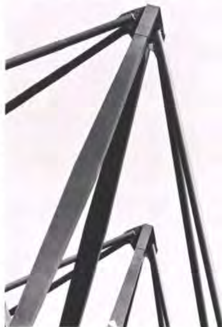
Fig. 14 Support pyramid showing capping piece (Photo: Harry Sowden)
