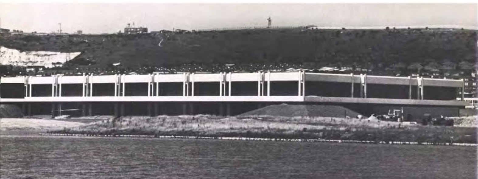
Fig. 29 (below) Phase 3: general view across lake (Photo: Arup Associates)
