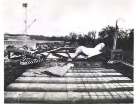
Fig. 15a Steel template (Photo: copyright Greater London Council)
