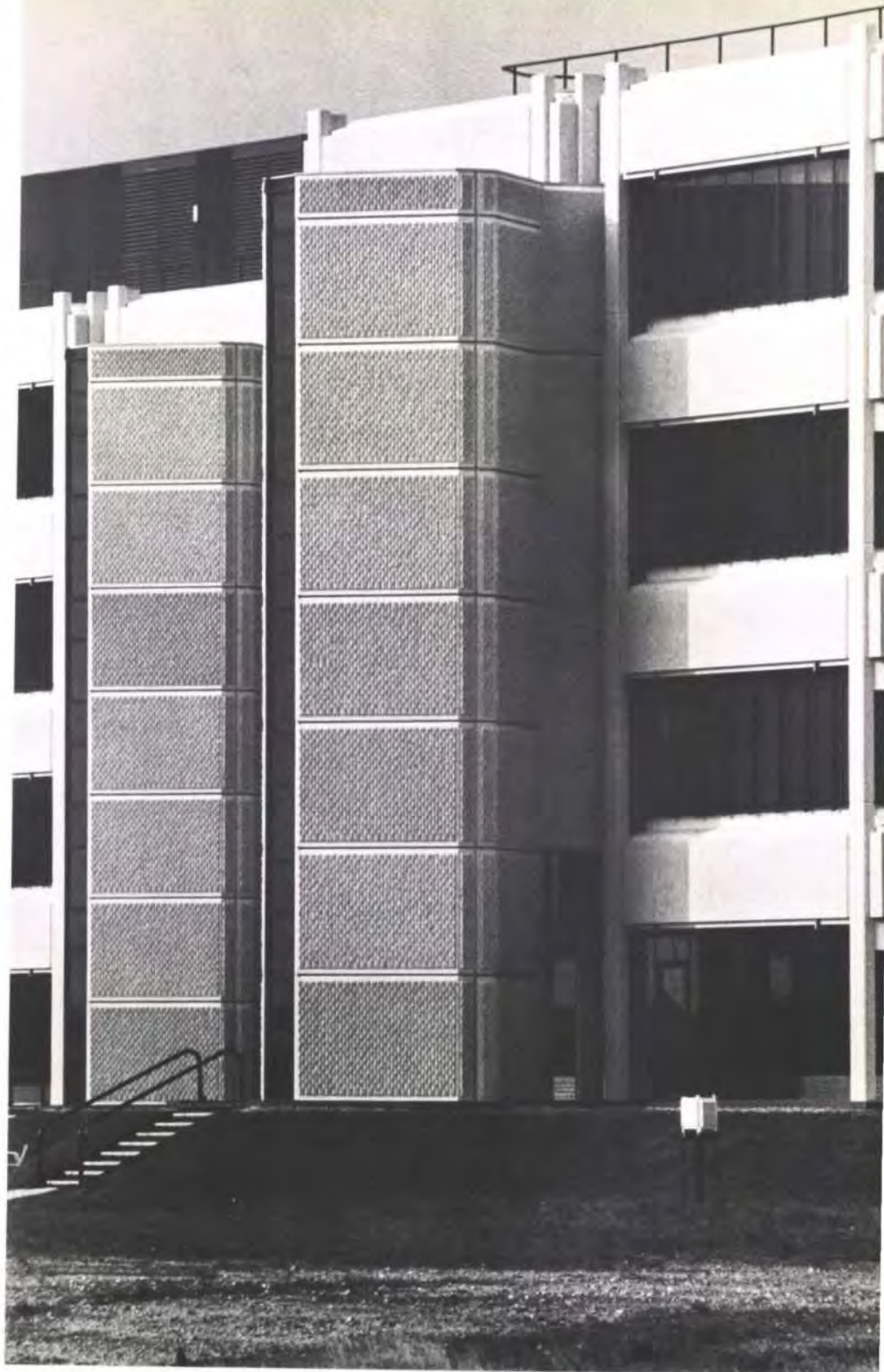
Fig. 14 Phases 1 and 2: escape stair towers (Photo: Arup Associates)
