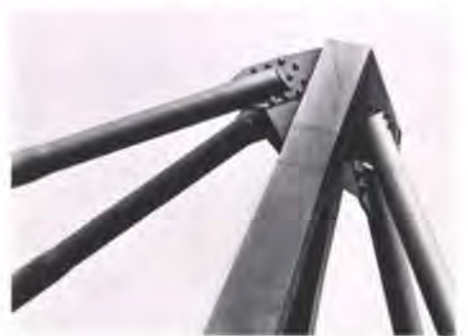
Fig. 6 Capping piece (Photo: Harry Sowden)
