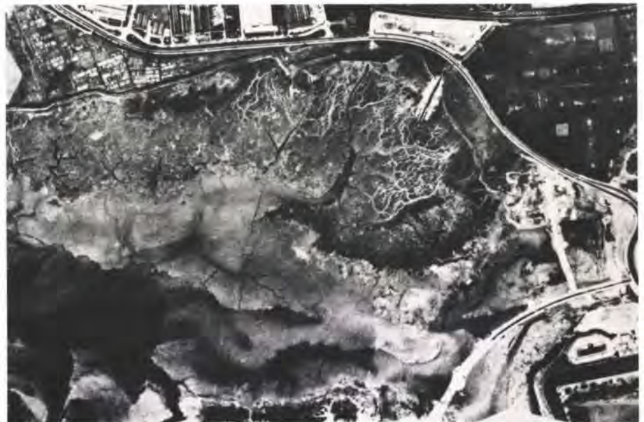
Fig. 1 The site prior to reclamation (Photo: Handford Photography)
