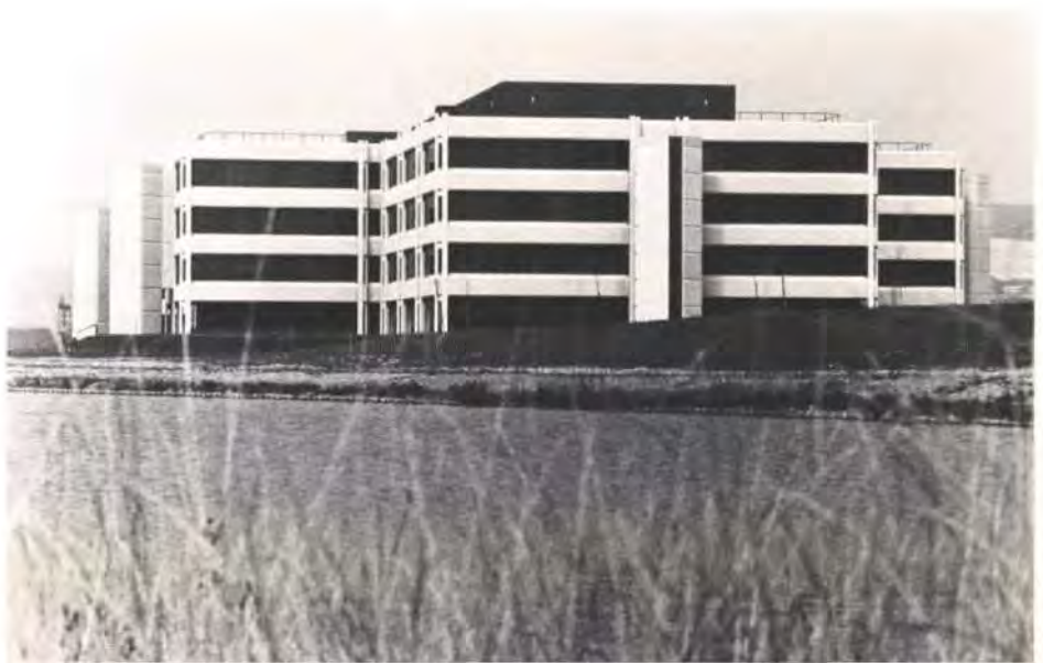
Fig. 11 (left) Phases 1 and 2 under construction (Photo: Arup Associates)
