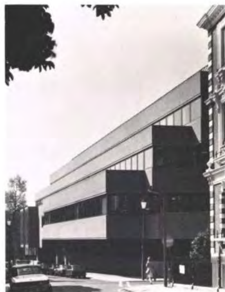
Fig. 5 Elevation from north side (Photo: Henk Snoek)
