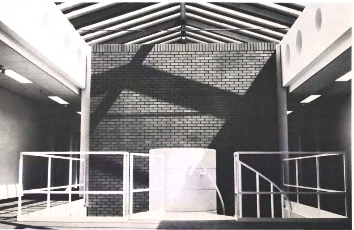
Fig. 35 Phase 3: stair landing at first floor (Photo: John Hopkins)
