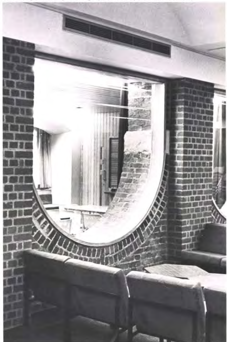
Fig. 11 The Waldegrave Hall: Close-up of glazed inverted arches, looking into cafeteria and showing ventilation grille through spandrel beam (Photo: Poul Beckmann)
