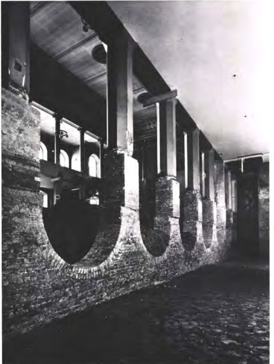
Fig. 2 Inverted arches under south aisle gallery (Photo: Thomas-Photos)
