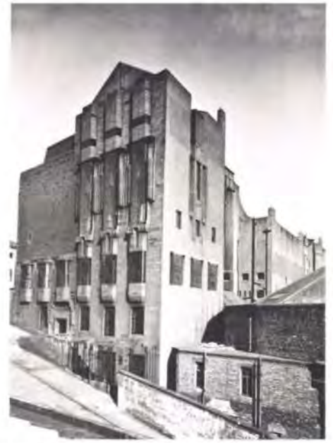
Fig. 5 West façade of Glasgow School of Art (Photo: Annan Photographer, Glasgow)
