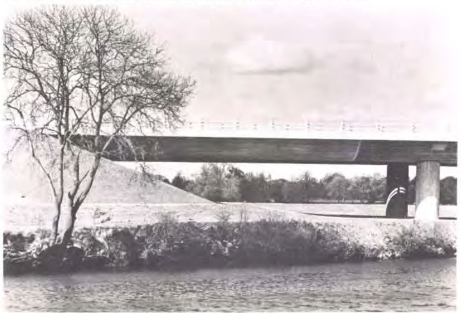
Figs. 6 and 7 The river columns relate to the river, the columns on land to the abutments
