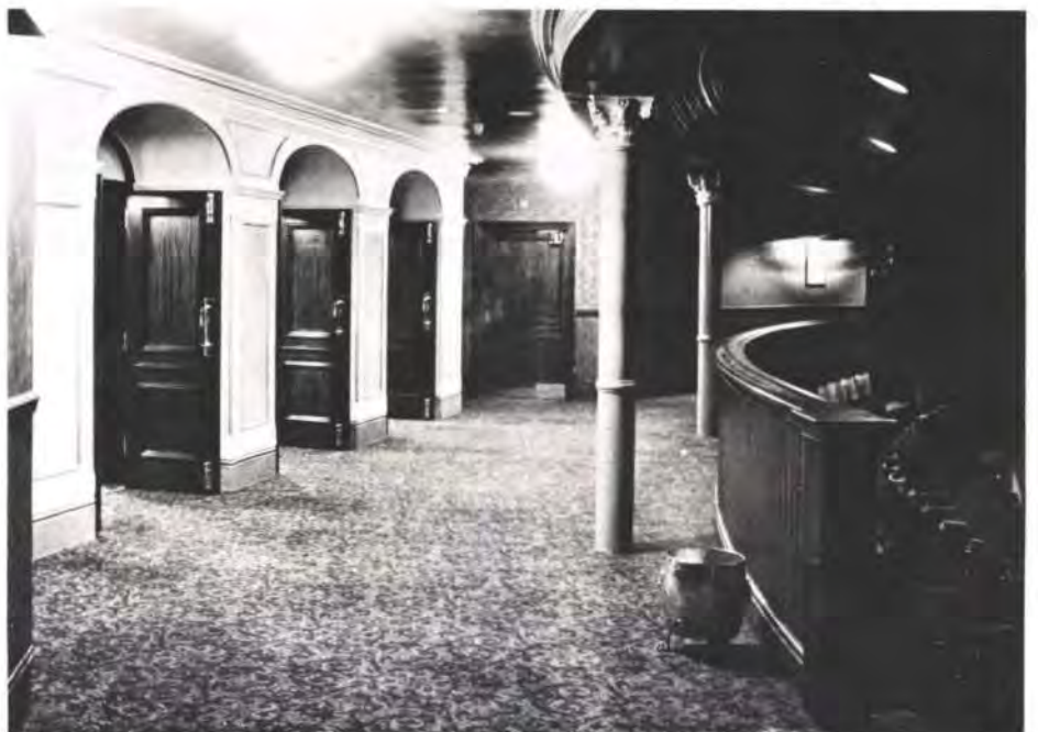
Fig. 12 The 1st tier, showing soffit lights and the fibrous plaster profiles which mark the air distribution outlets
