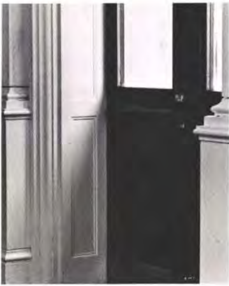
Fig. 8 Detail of joinery in the foyer
