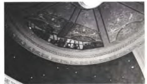
Fig. 10 Interior of the dome, showing trap doors concealing lighting for the stage
