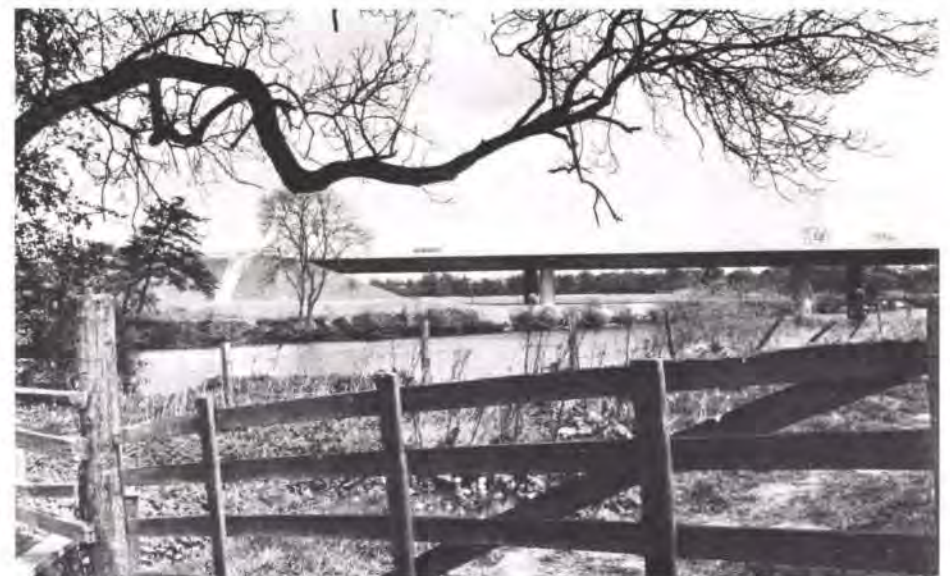
Fig. 10 The abutments are well back from the river banks and the character of the river is kept
