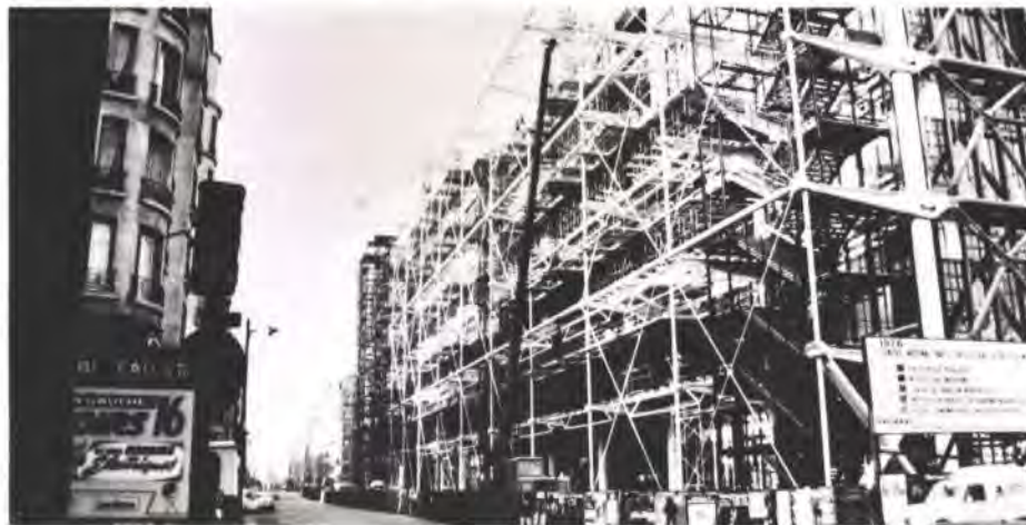
Fig. 1 Centre Pompidou, Paris (Photo: Mike Sargent)
