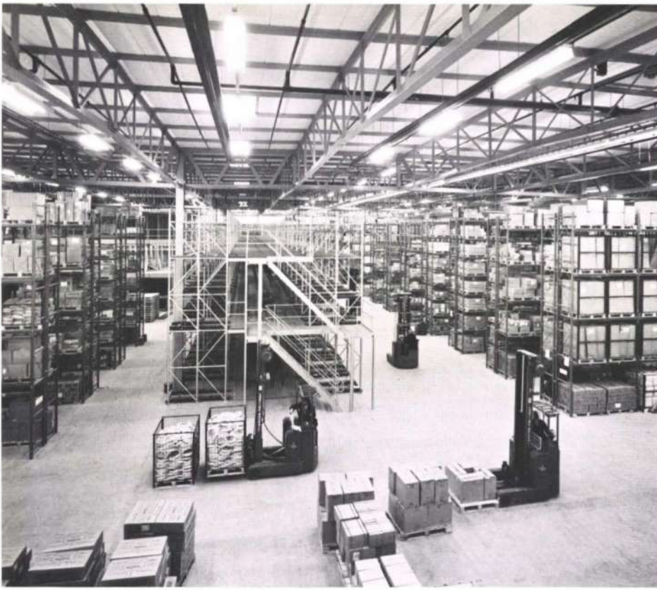
Fig. 4 Interior view of warehouse showing lattice truss roof. Three tier steel racking for 'Speedflow' system is in centre, while bulk storage racking is shown to either side
