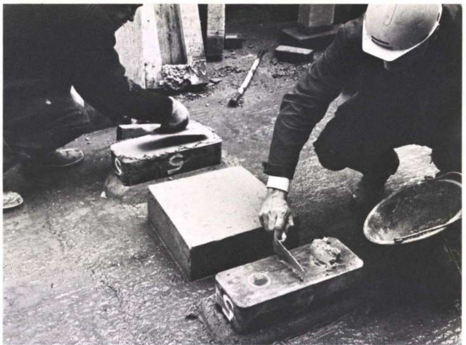
Fig. 4 Bedding in the bearings (Photo: Mark Gerson)
