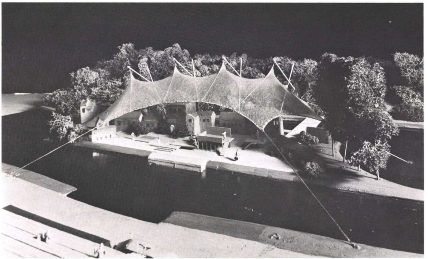
Fig. 13 Scarborough open air theatre: view of stage from seats
