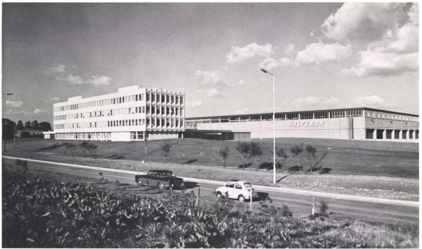
Fig. 2 Front view of office block and warehouse
