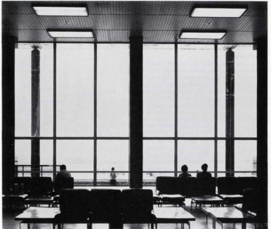
Fig. 7 View on to apron from public area of first floor departure concourse. Note steel cruciform columns supporting roof in the background
