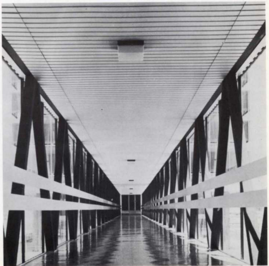
Fig. 4 below Detail of overhead pedestrian link between administrative office block and terminal building constructed with structural steel
