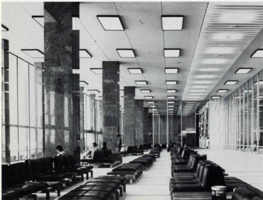
Fig. 6 The public section of the first floor departure concourses. Note the granite finish to columns
