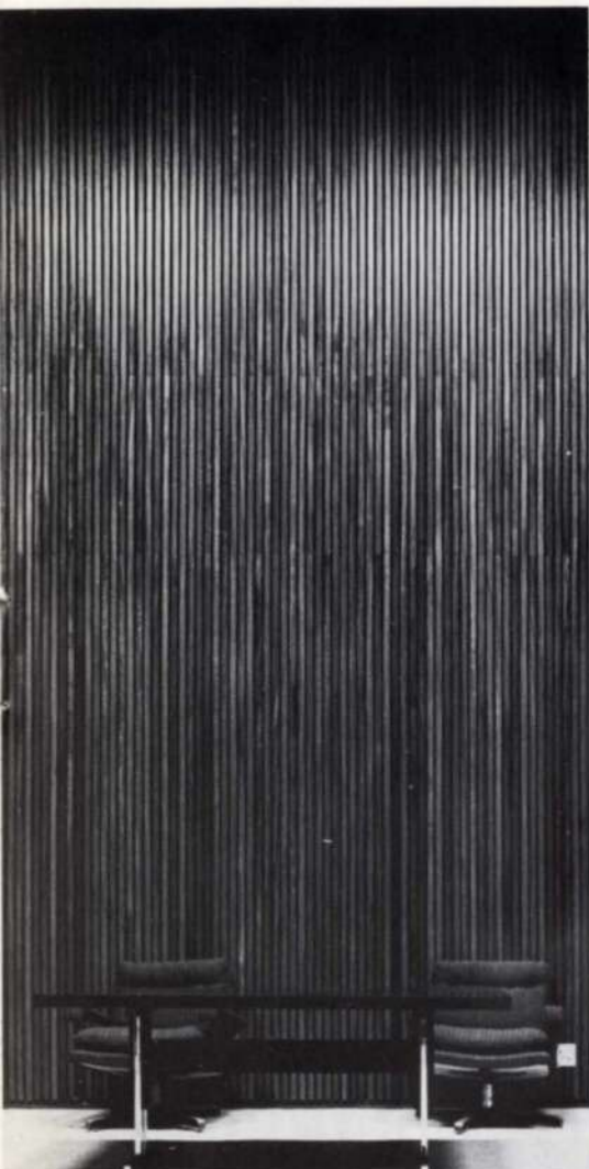
Fig. 2 Detail of strip timber panelling in TV auditorium
