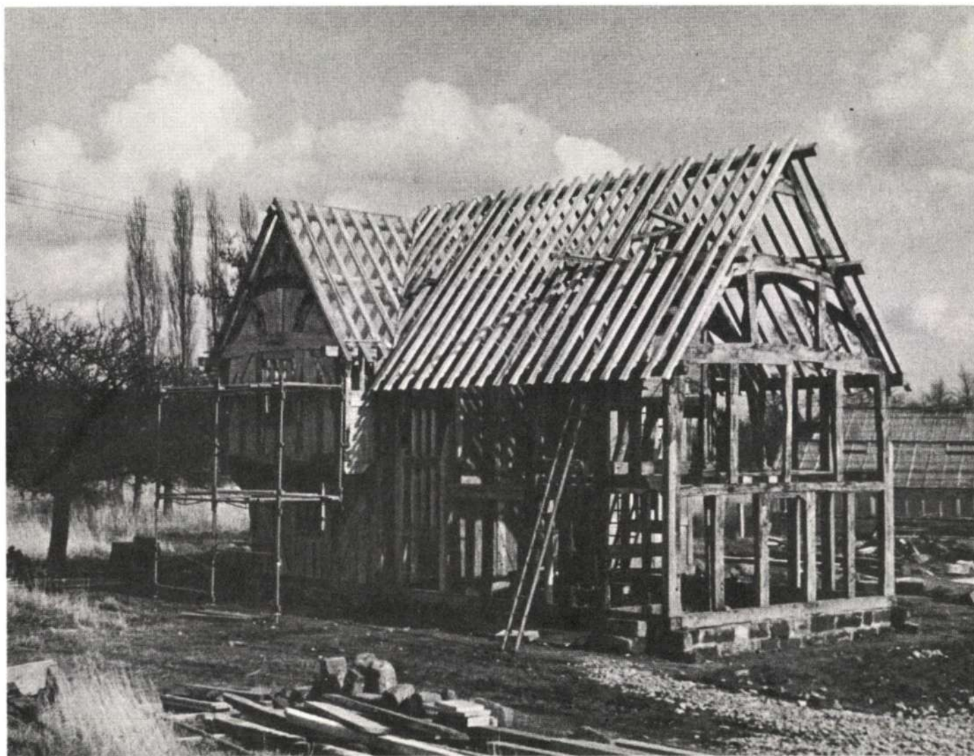
Fig. 3 The Bromsgrove House— frame of hall nearly completed (Photo: John Aulton)
