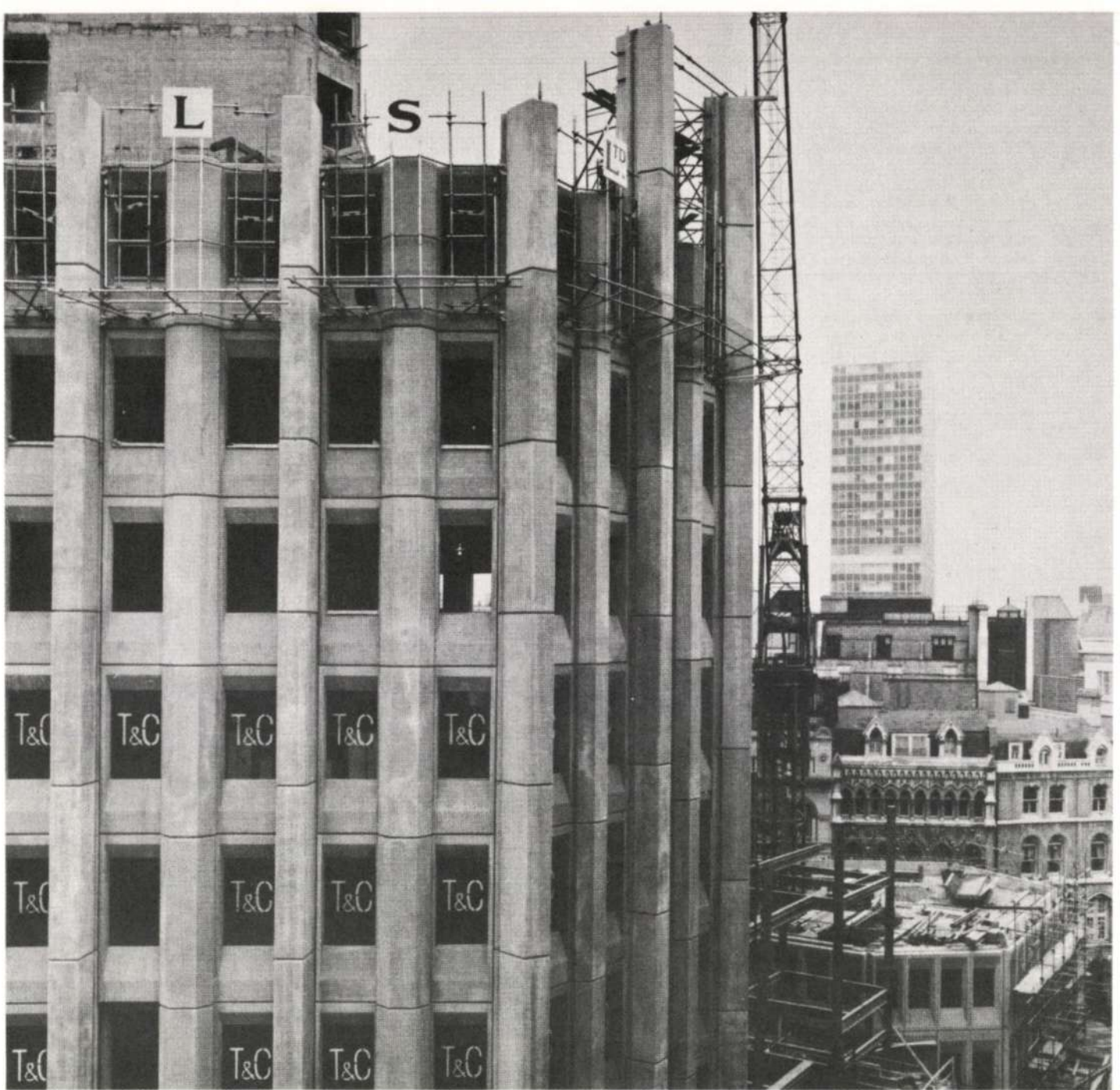
Fig. 12 Precast column and spandrel units (Photo: Sydney W. Newbery)
