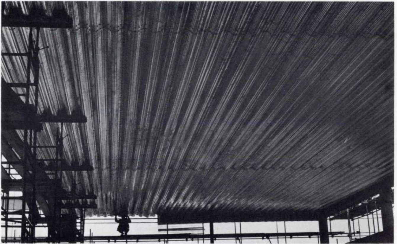
Fig. 5 Ceiling view showing soffit steelwork. (Photo: J. Levy)
