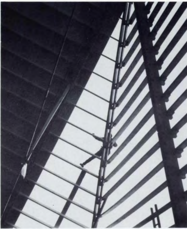
Fig. 27 Roof under construction Photo: Zetta Barron
