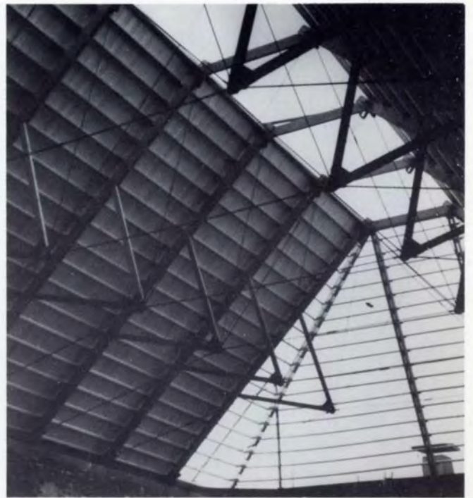
Fig. 28 Roof under construction Photo: Zetta Barron
