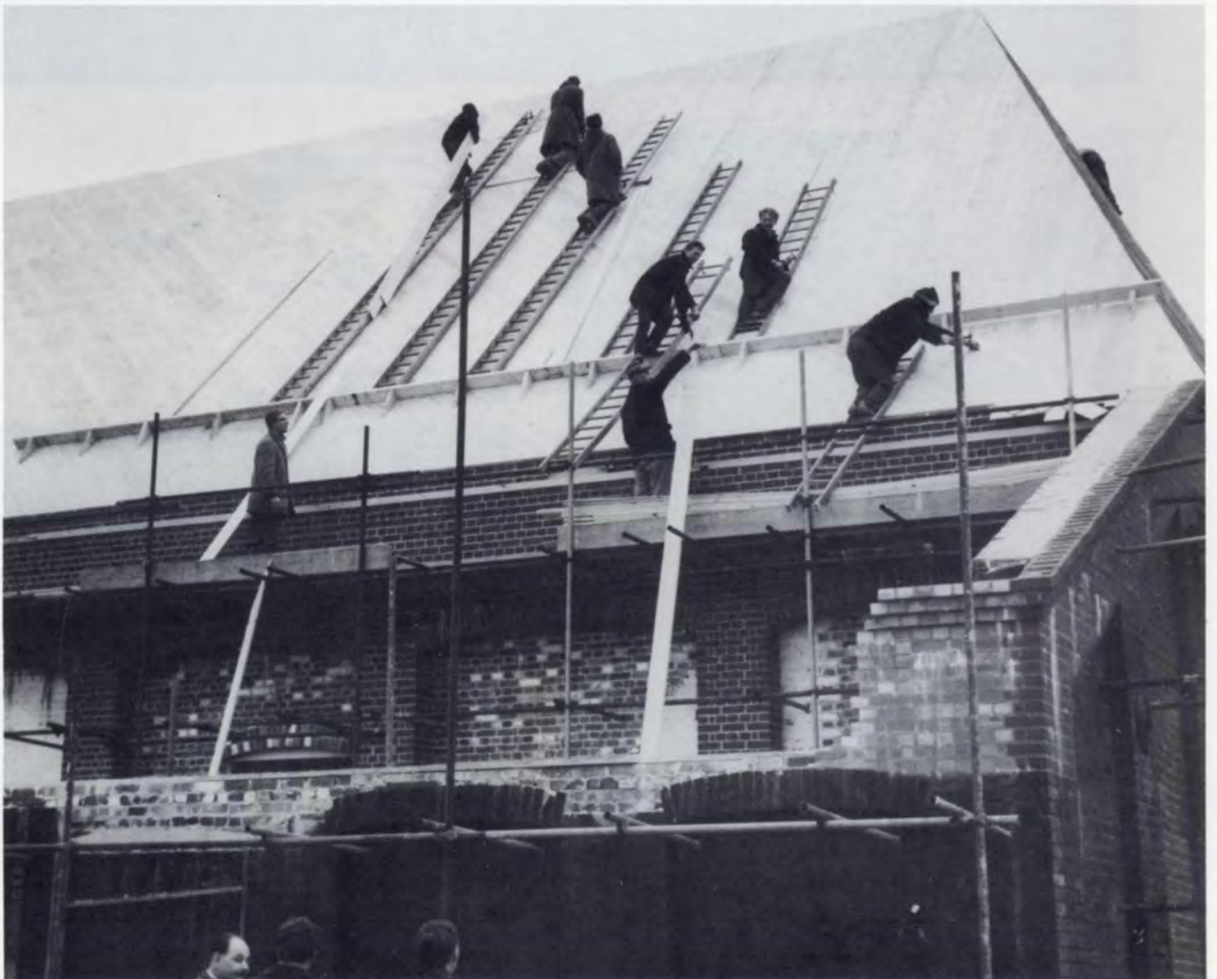
Fig. 29 Two layers of 1 in. boarding Photo: Zetta Barron
