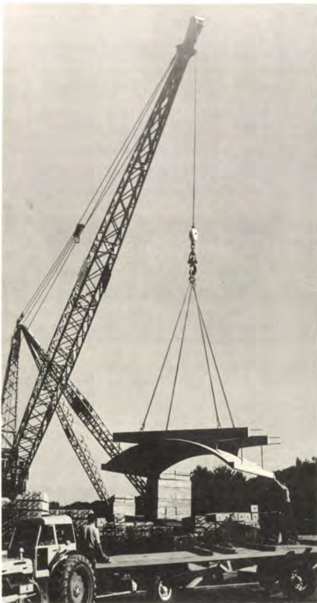
University of Sussex - Crane lifting vault unit
